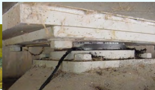
Excessive leakage of rubber
