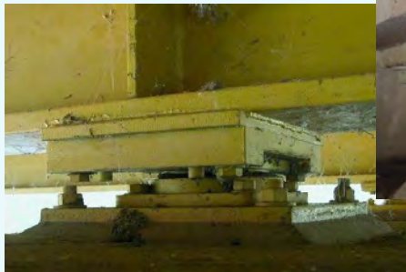
Bearing at extension limit
