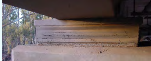
Cracking & splitting
