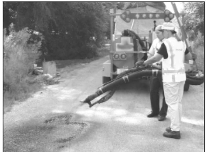
Teresa Price, IDOT, fills a pothole using spray injection technology with the assistance of Cliff Dickehut of Dura Patcher.
