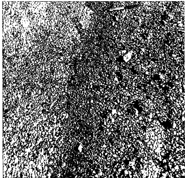
Figure 24. February 14, 1967. Closeup photographs of the condition of the SA-1 treated material where raveling has occurred.
