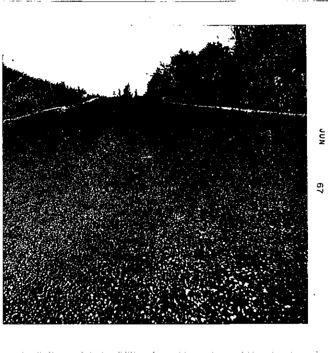
Figure 16. October 25, 1967. The appearance of the seal coated surface. Figure 17.
