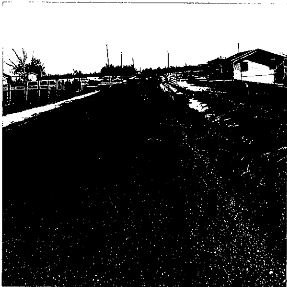
Figure 20. February 14, 1967. Raveling along the edges of the road.
