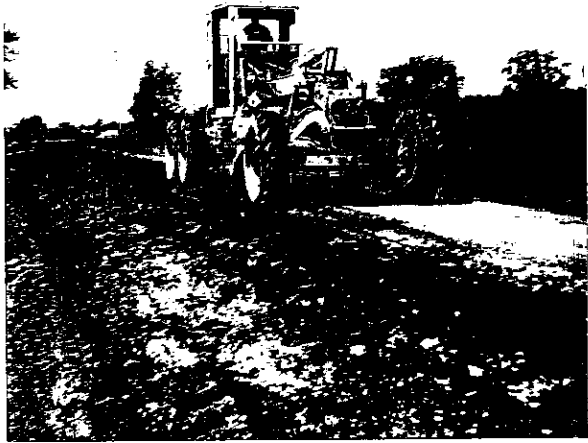
Figure 2. The grader scarifying the surface.
