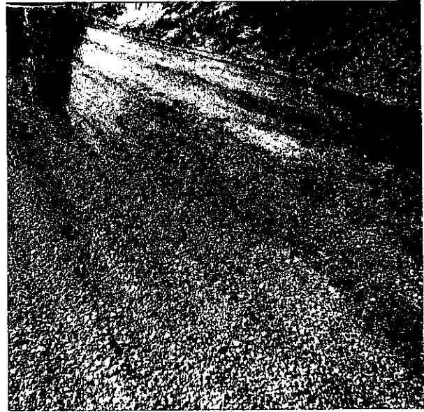
Figure 22. February 14, 1967. Raveling along the edges of the road.
