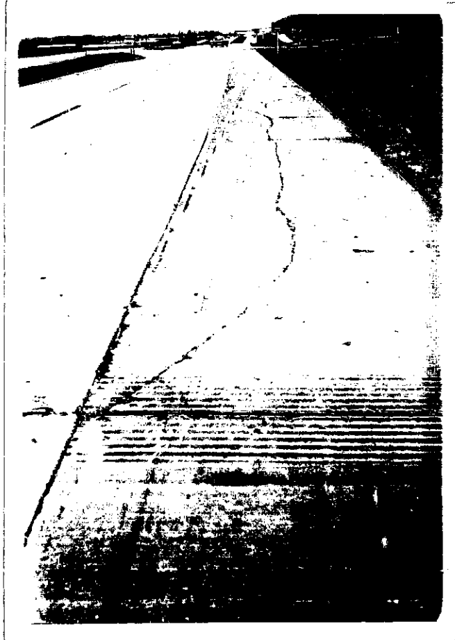
Figure 12. Longitudinal crack in this test section is caused by use of shoulder as a right-turn lane by heavy vehicles. Intersection can be seen in the background.
