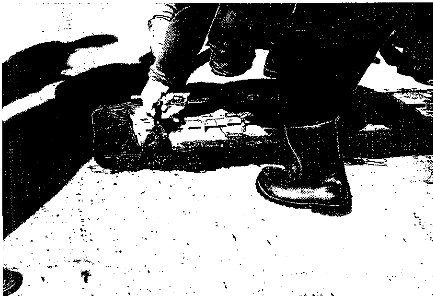
Bitumen being troweled over perforated metal strip to form smooth transition between sensor and pavement surface.
