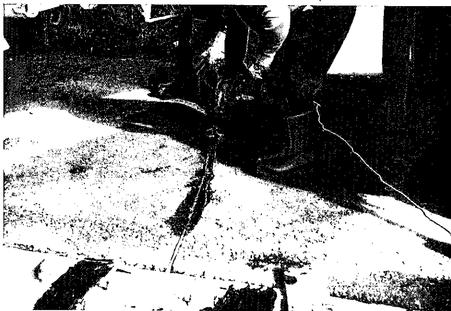
Cable slot being filled with bitumen. Note double fold of clothesline rope atop cable.
