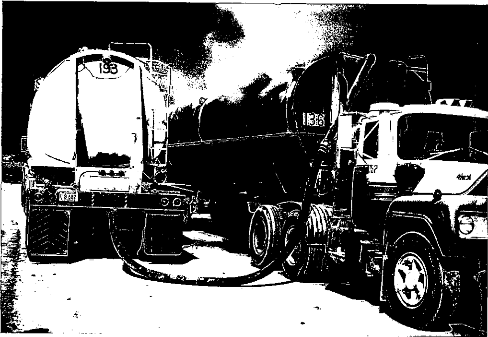
Figure 3. Transport tanker loading distributor truck for placement of lime on embankment
