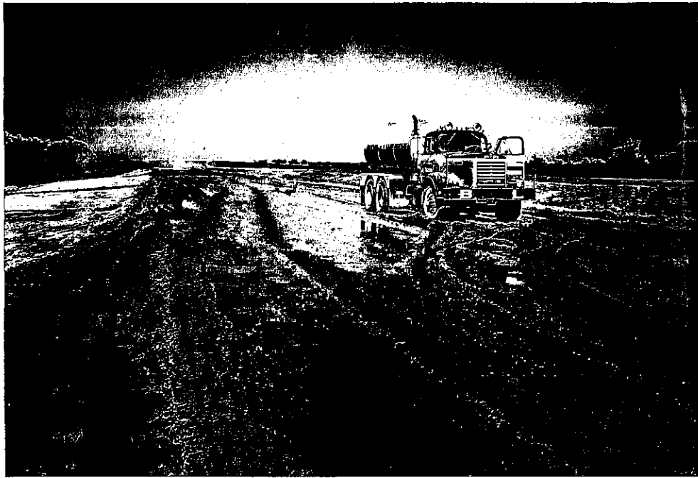
Figure 6. Water truck on embankment at completion of wetting operation
