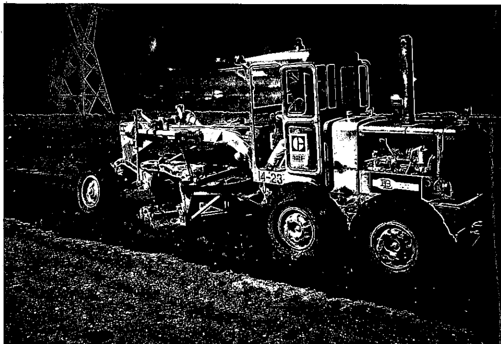
Figure 11. Motor grader scarifying soil
