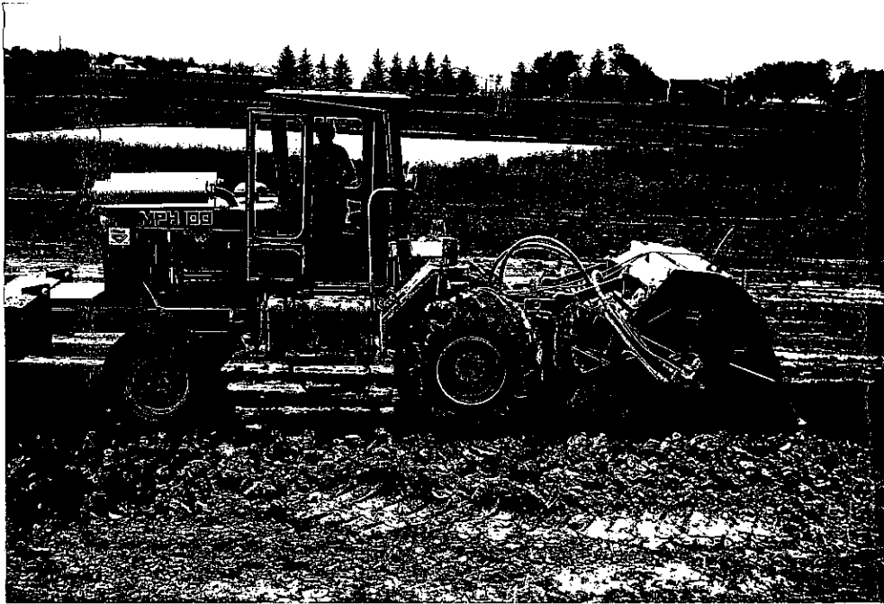
Figure 7. Tiller used at beginning of construction
