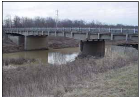
Existing US 45 Bridge over North Fork Saline River, Looking Northeast
