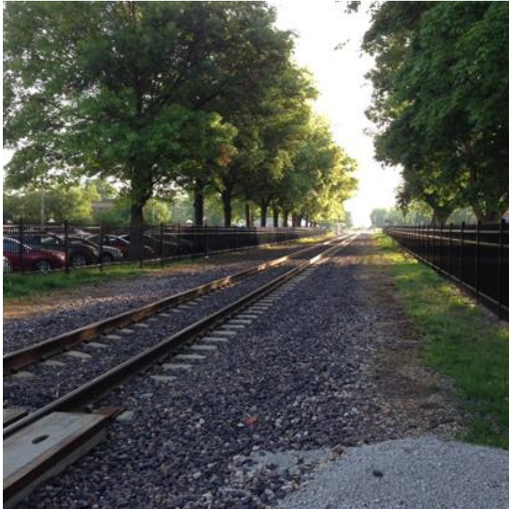
Figure 5.7 Fencing Installed in Dwight, Illinois as Part of Illinois High Speed Rail Project
