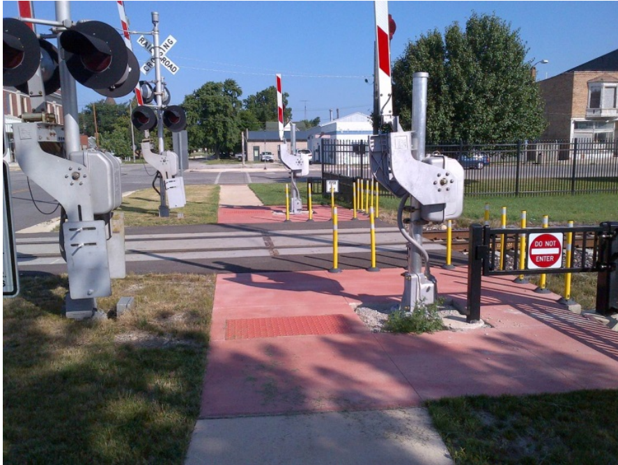
Figure 5.6 Quad Gate Arms in Odell, Illinois
