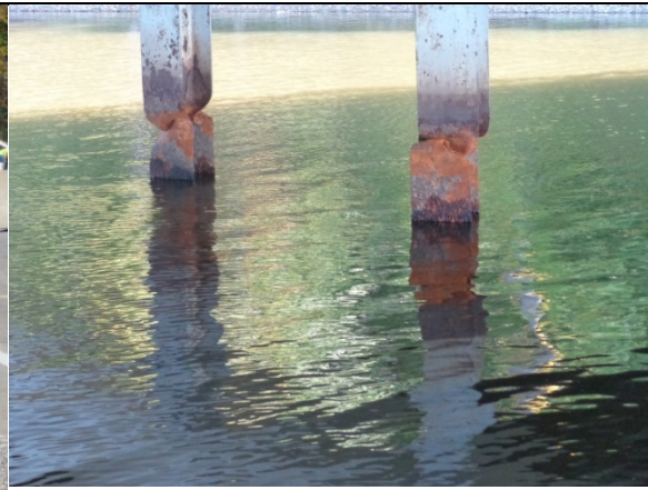
6. Photo - - October 6, 2016 - Facing east from west bank
