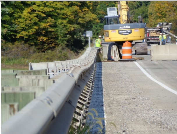
5. Photo -- October 6, 2016 - Facing west from east approach
