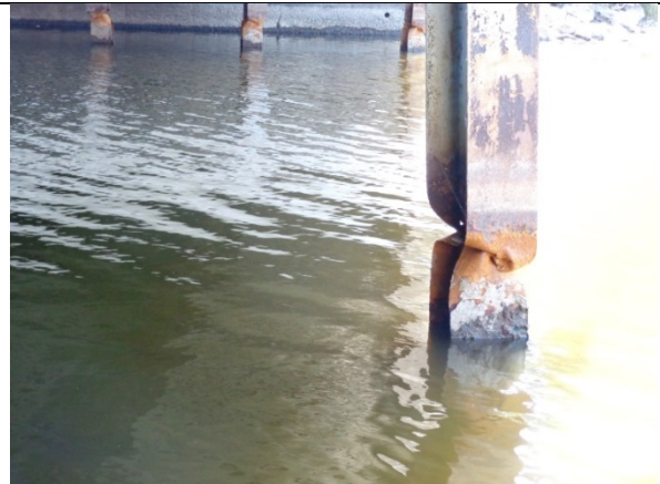
4. Photo - October 6, 2016 – Facing east from west bank
