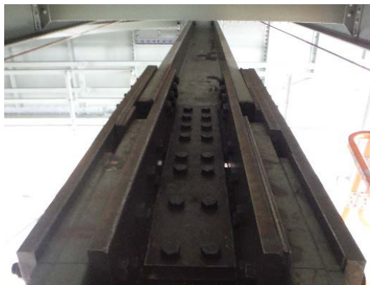
Figure 4 Splice plates on U19-19', looking west from panel point 19'. (HNTB)
