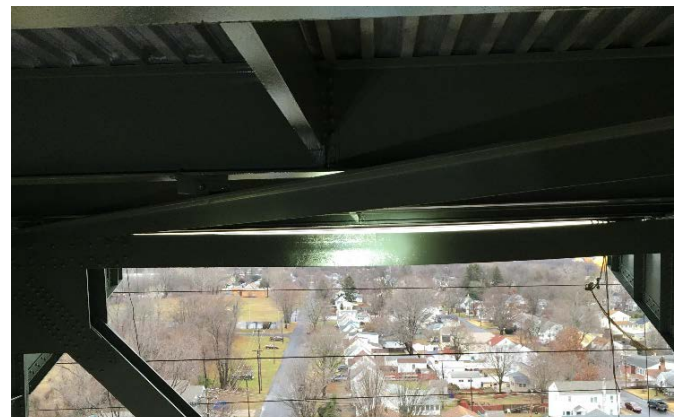
Figure 10 Elastic bowing in U19'-17', between panel points U19' and U18'. (HNTB)
