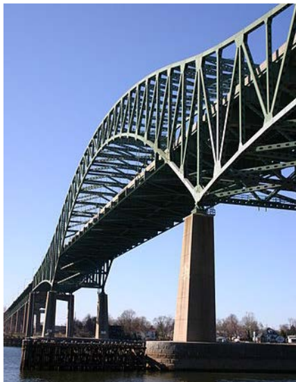
Figure 1 Main river span
