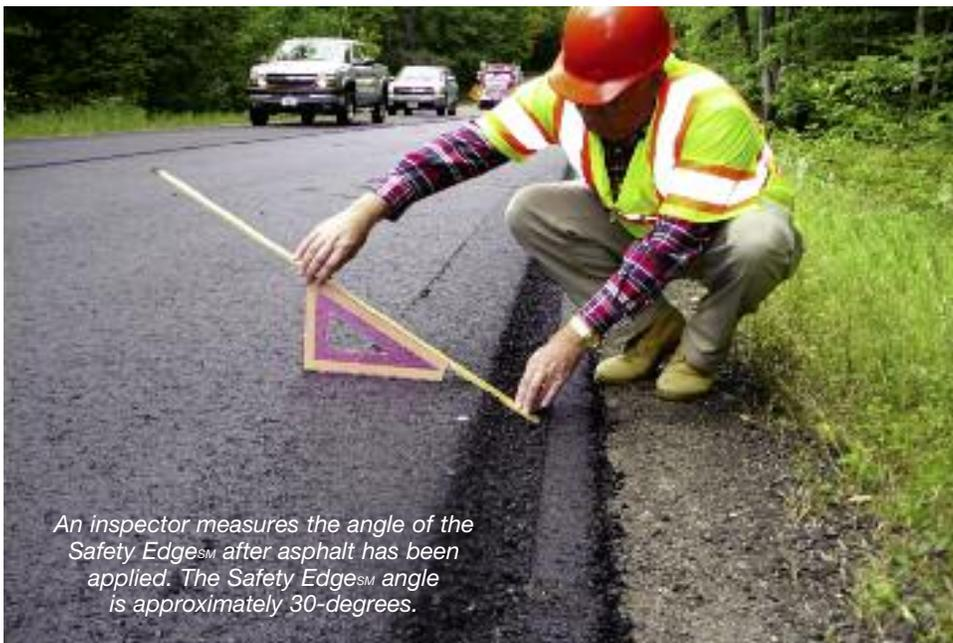
*An inspector measures the angle of the Safety Edge<sup>SM</sup> after asphalt has been applied. The Safety Edge<sup>SM</sup> angle is approximately 30-degrees.*
