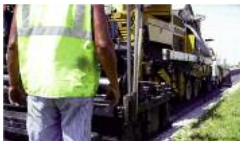
A road crew lays down the Safety Edge<sup>SM</sup> using existing pavement equipment that has been retrofitted at minimal cost.
