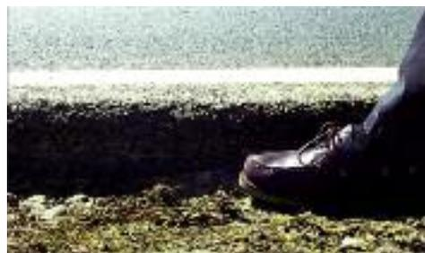
Shows a dangerous pavement drop-off without a Safety Edge<sup>SM</sup>. If a motorist inadvertently leaves the roadway, bringing the tires back onto the pavement is more difficult—and dangerous—with a steep-angled surface.
