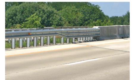
**MGS TERMINALS:** Several terminal designs have been modified or developed so they can be used to terminate the 31-inch high MGS design. These changes generally involve shallower embedment of standard terminal posts so the terminal railing matches the 31-inch height and developing adequate anchorage. MASH 16 terminals are available; see the IDOT Qualified Products List <http://idot.illinois.gov/doing-business/material-approvals/metals/index>.
