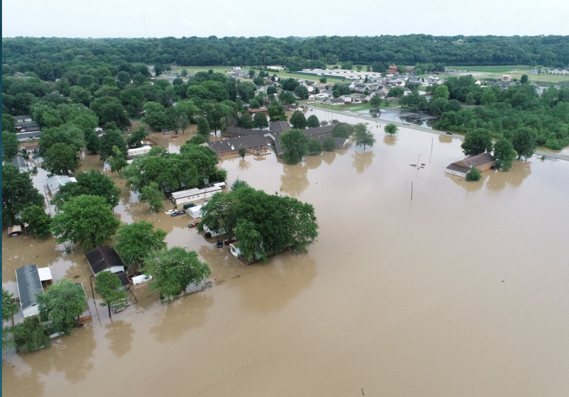
Caseyville – Little Canteen Creek Levee overtopped
