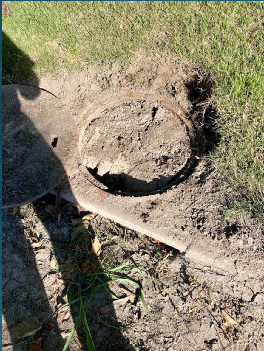
Plugged Storm Sewer Inlets
