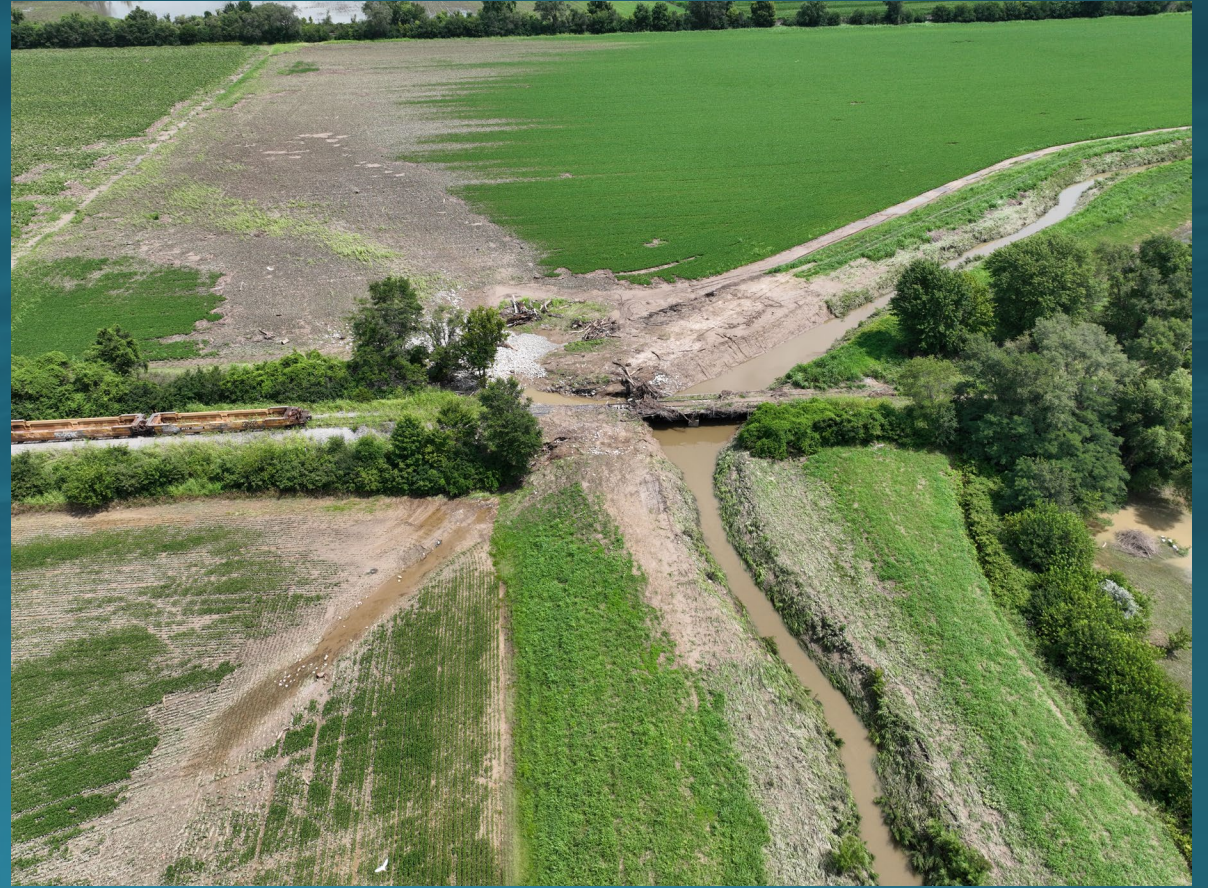
Caseyville- Notched the Little Canteen Creek Levee. Prevented the July 2022 flooding from re-occurring
