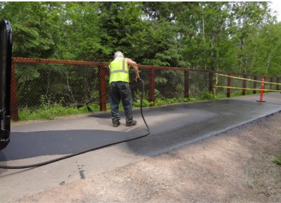
Figure 15-4: Fog Sealing a Shared Use Path
