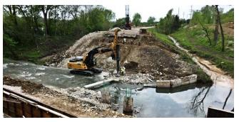
The \$1.5 million project involved the removal and replacement of the three-span U.S. 52 bridge as well as resurfacing, ditch work, culvert replacement and safety enhancements.
