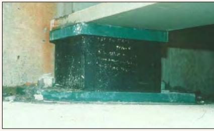
Lead Core Seismic Isolation Bearing
