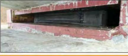
Element 310 - Bearings constructed primarily from elastomeric material (ex. rubber, neoprene) that may contain fabric or metal reinforcement
