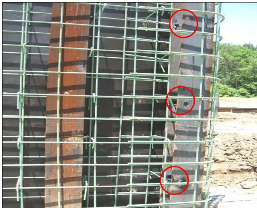
Example of Holes Cut in Piles for Form Ties
