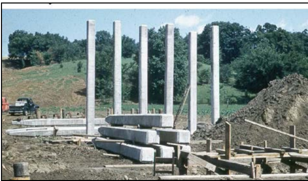
Concrete Piles: Friction Piles
