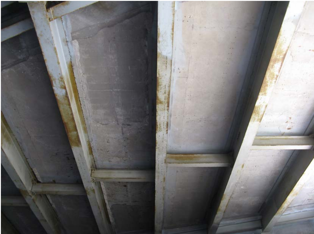
Photo 2 - Underside of Span 3, looking east
