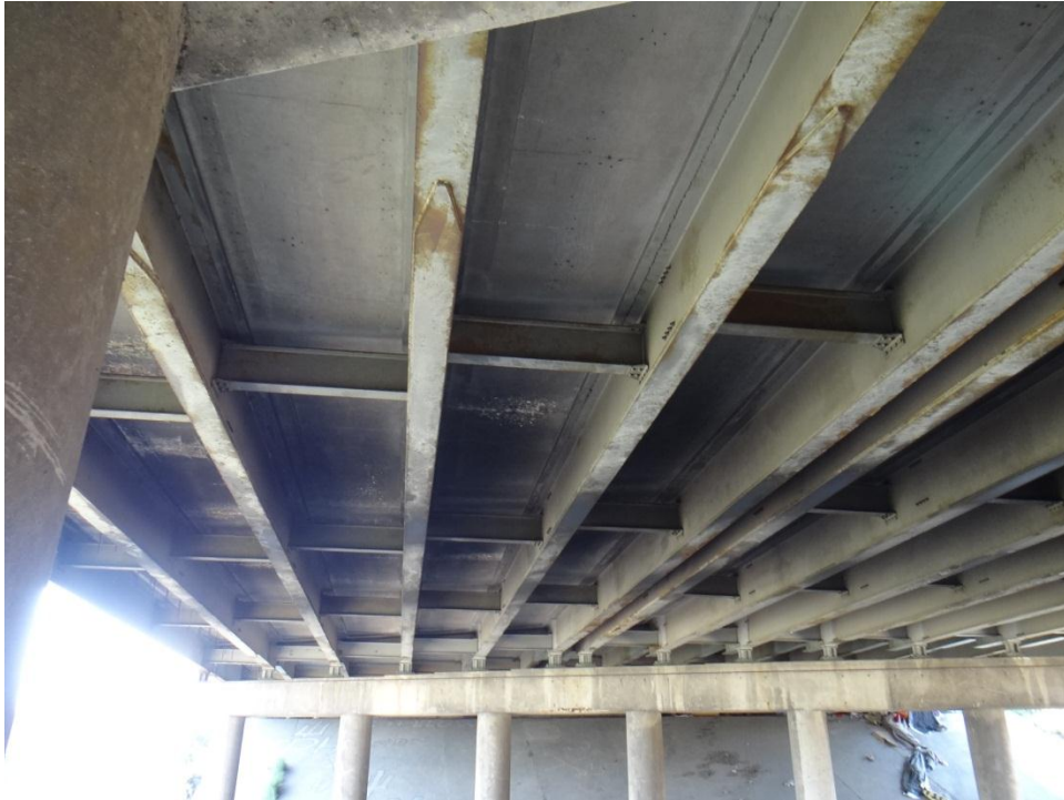
Figure 2. Typical view, deck soffit, looking west.
