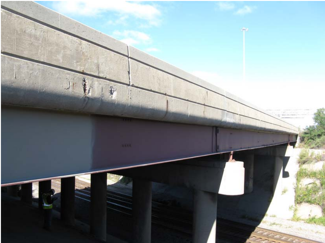
Photo 14 - South fascia beam, looking northeast
