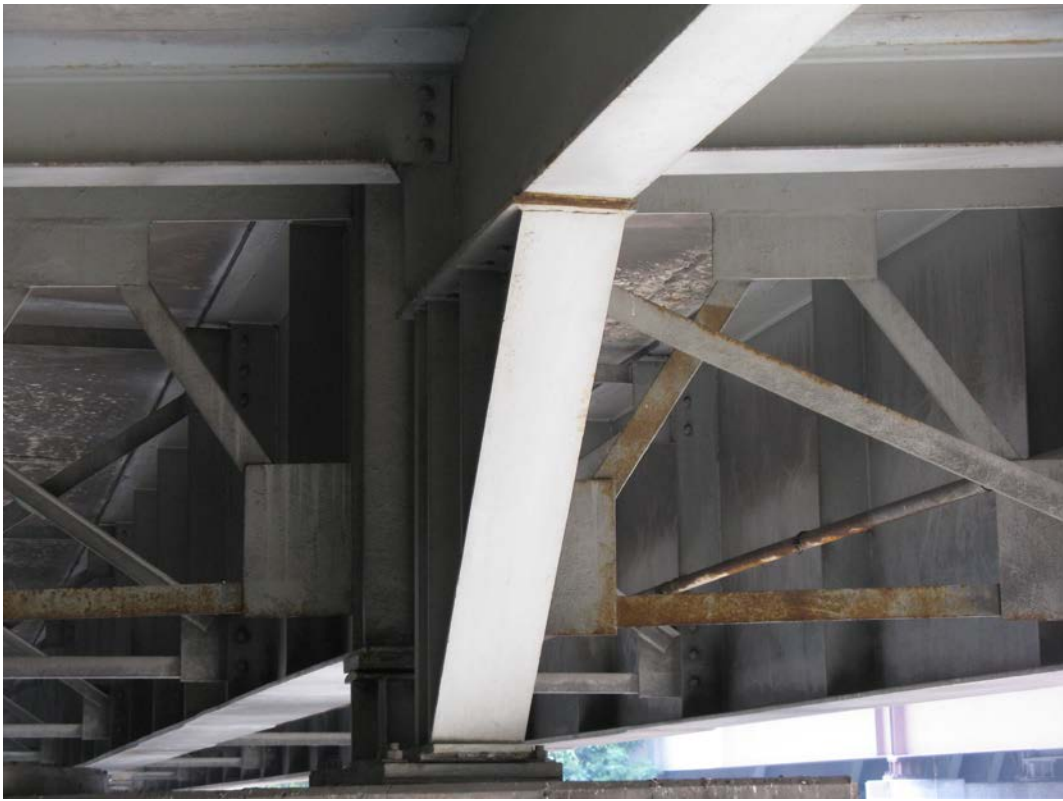
Photo 12 - Crack in built up pedestal on beam 9 from north at West Pier, west span, looking east
