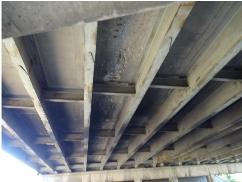
Figure 2. Typical view, deck soffit, looking west.
