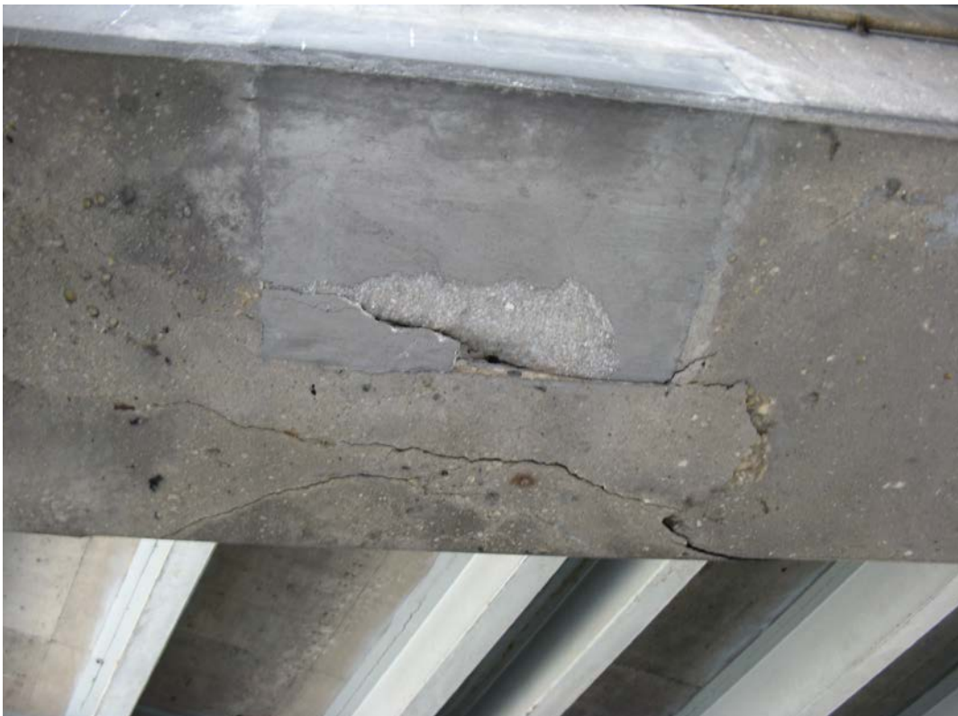
Photo 28 - Underside of East Pier cap between columns 1-2 from north, looking east
