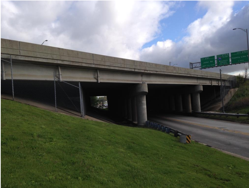
Photo 1: Structure overall, looking north east.
