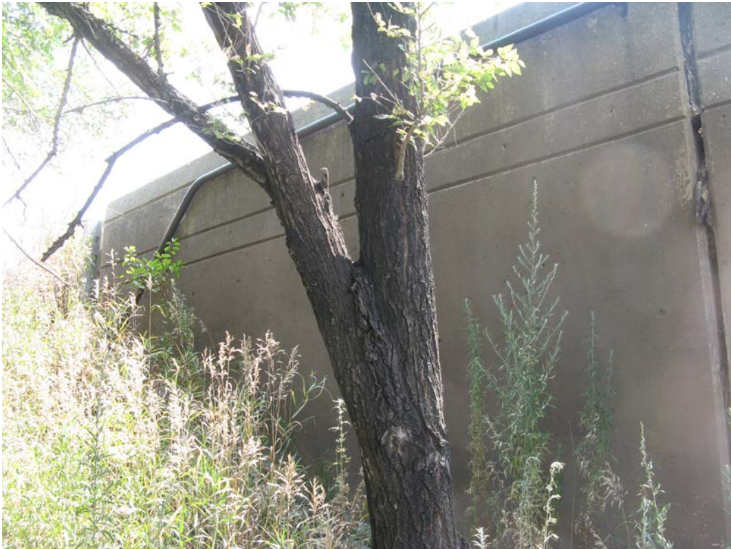
Photo 31 – Northeast wingwall, looking southeast
