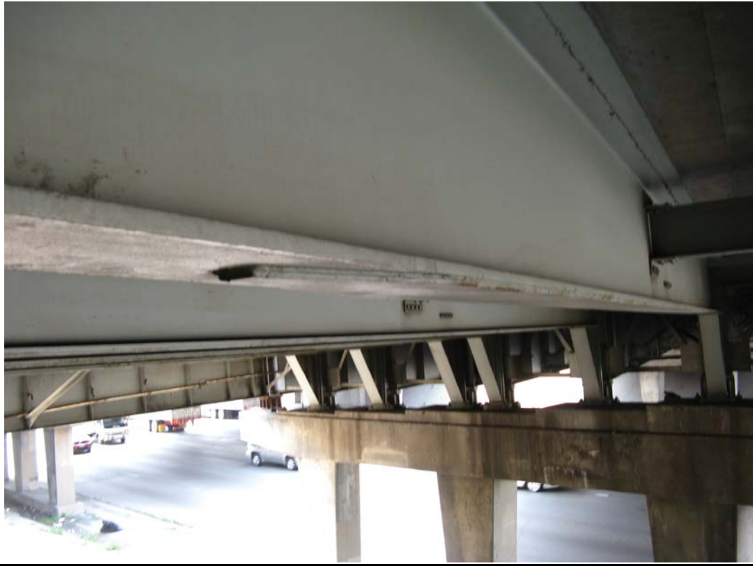
Photo 15 - Typical beam with cover plate in Span 1, Beam 4, looking southwest
