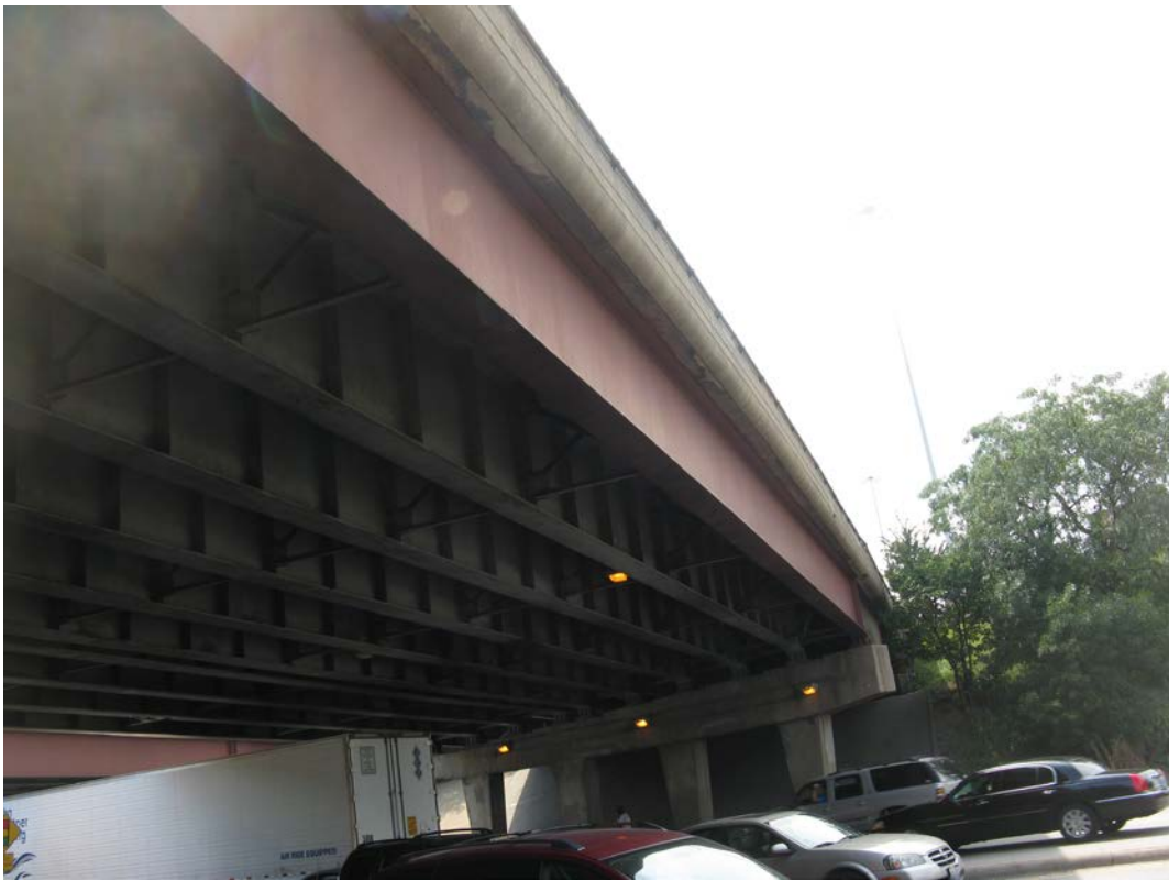
Photo 18 - North fascia beam, Span 2, looking west
