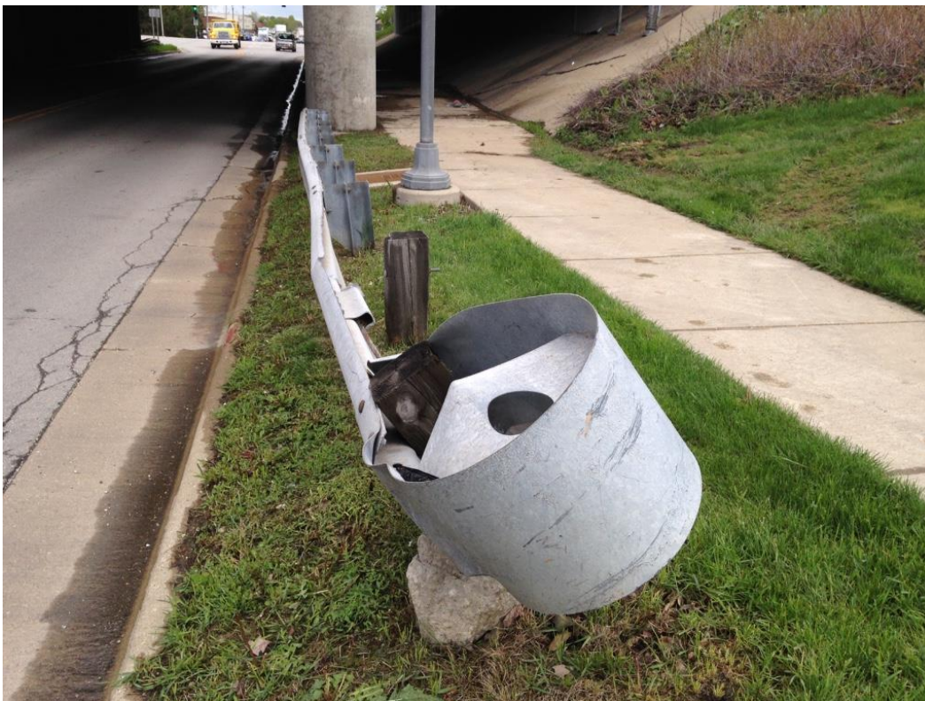
Photo 56: East approach guardrail on S Madison St. showing impact damage including detachment from first two wood posts.
