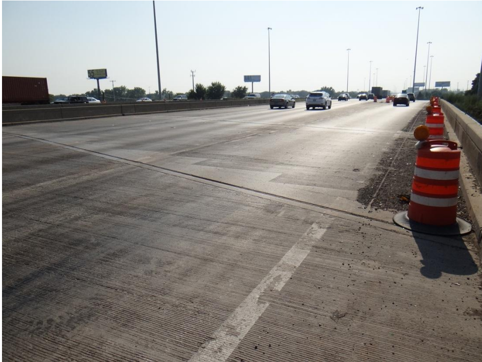
Figure 4. Typical view, deck top surface, looking southwest
