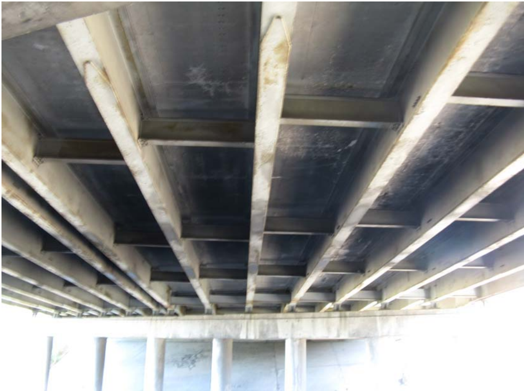
Photo 16 - Underside of Span 2 Beams, looking east
