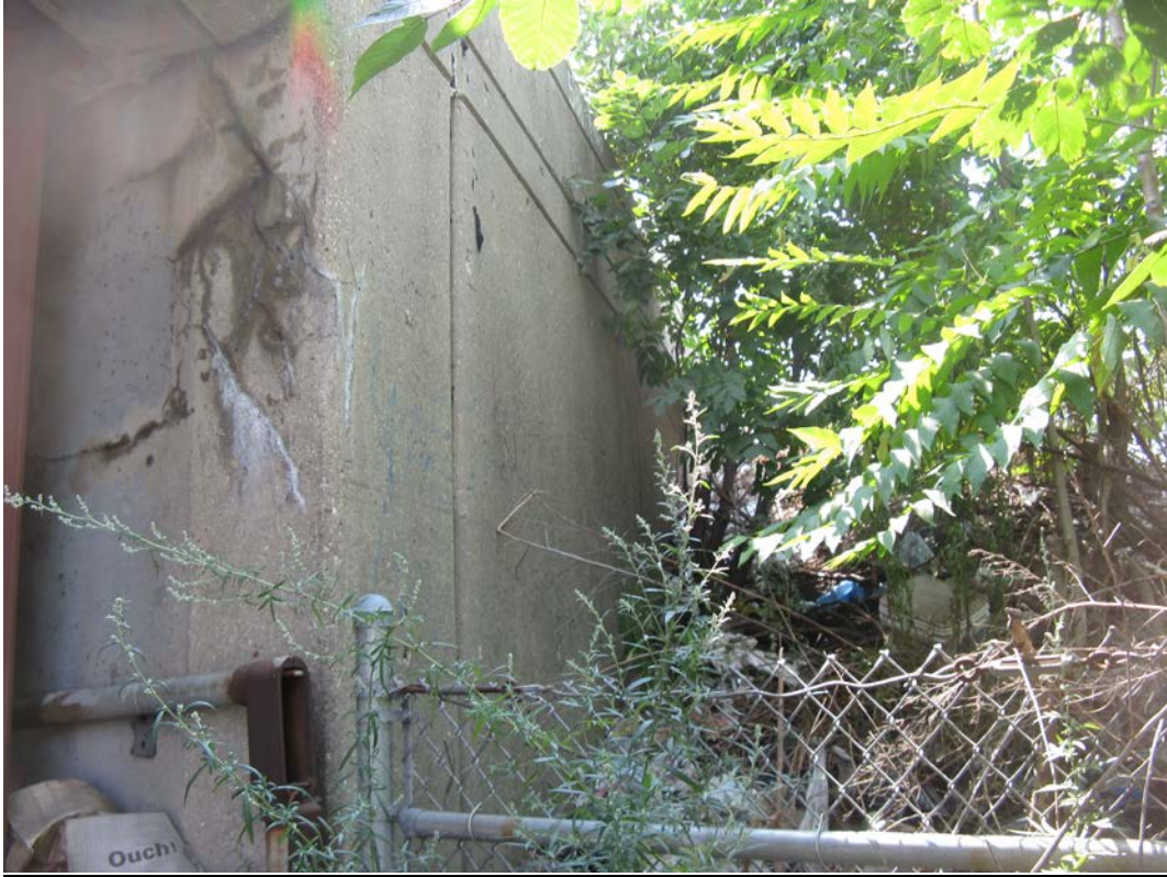
Photo 25 - Northwest wingwall, looking southwest
