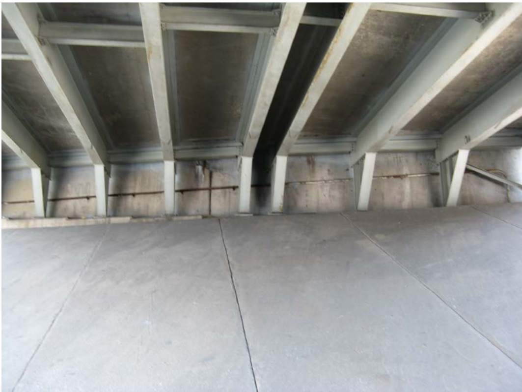
Photo 22 - East Abutment, looking east
