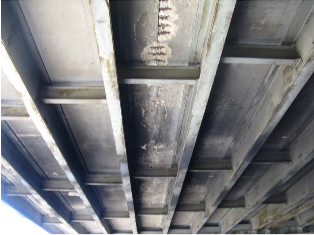
Photo 1 - Underside of Span 2, looking west
