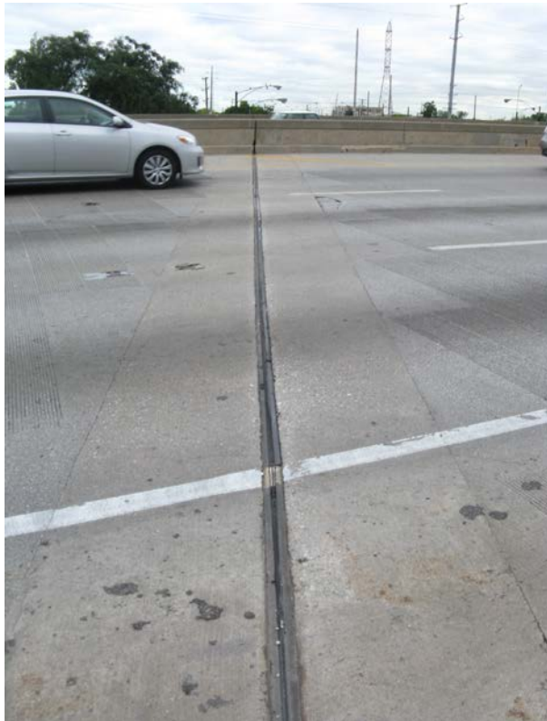
Photo 12 - Pier 1 joint, looking north
