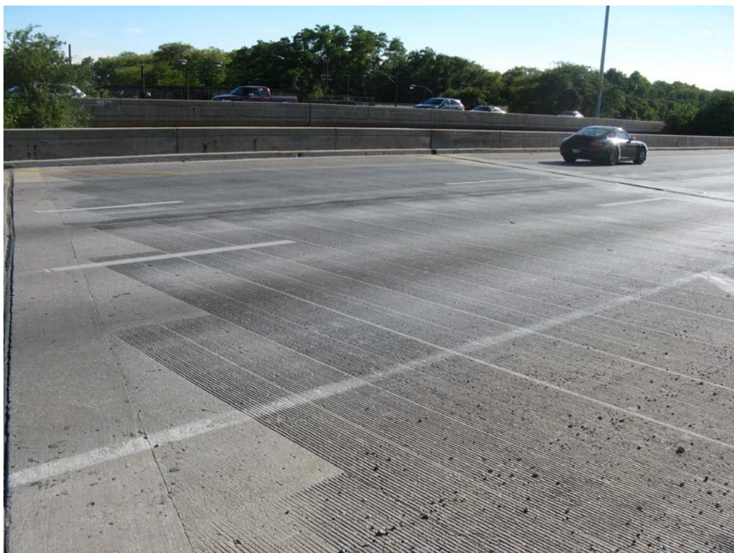
Photo 5 – Span 3, looking southwest
