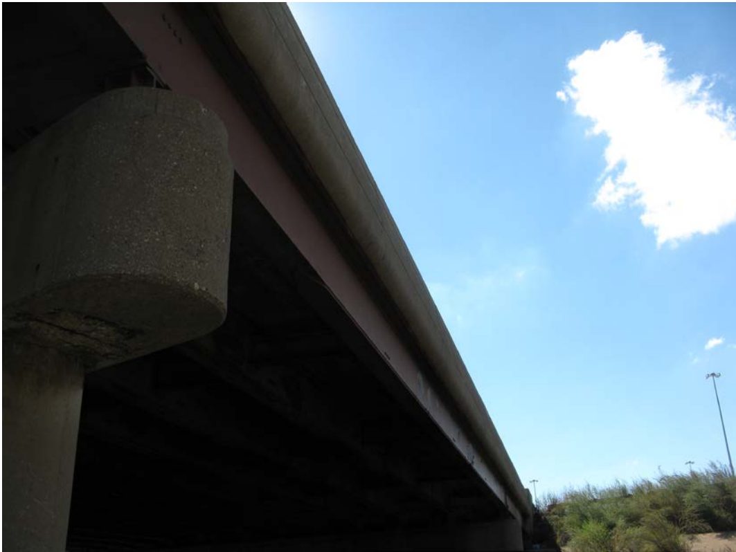
Photo 17 - South fascia in Span 3, looking northwest
