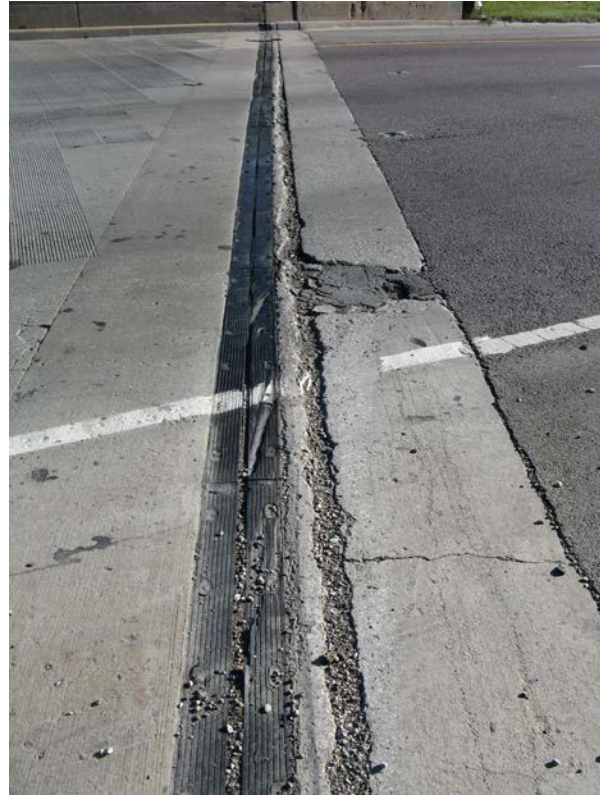
Photo 11 - West Abutment joint, looking south
