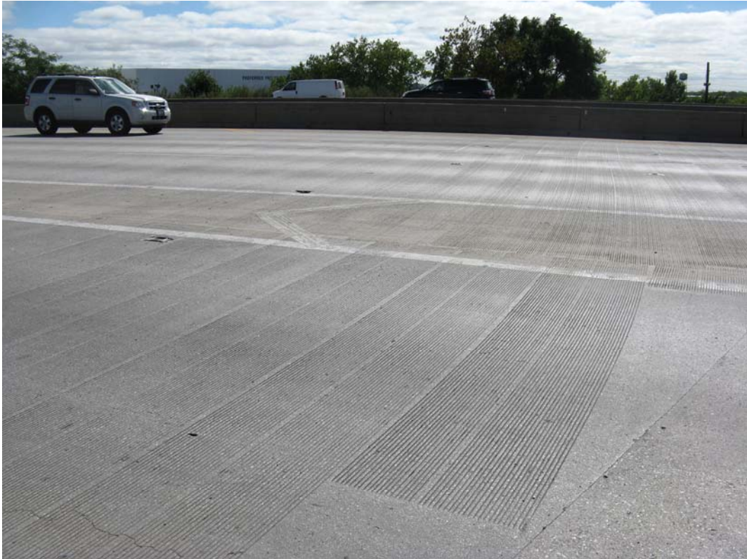
Photo 5 – Top of Deck, Span 1, looking south
