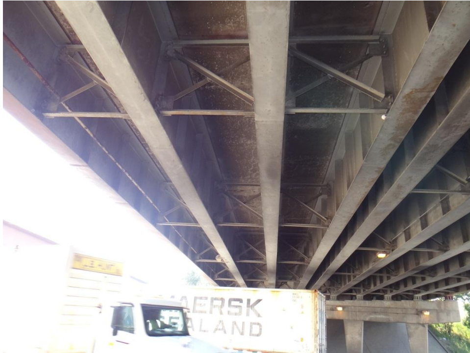
Figure 3. Typical view, deck soffit, looking west.
