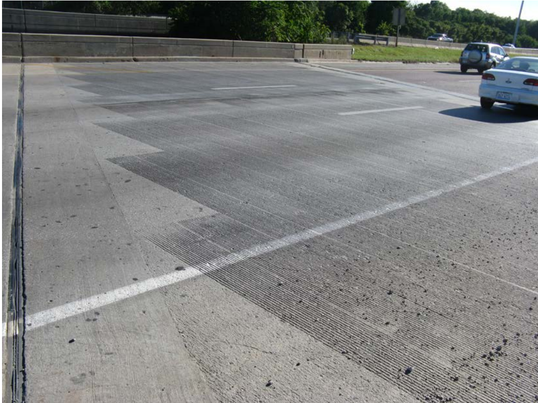
Photo 7 – Span 1, looking southwest
