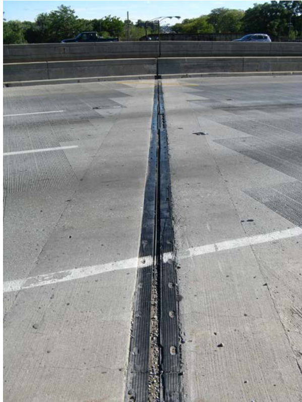
Photo 9 - East Pier joint, looking south
