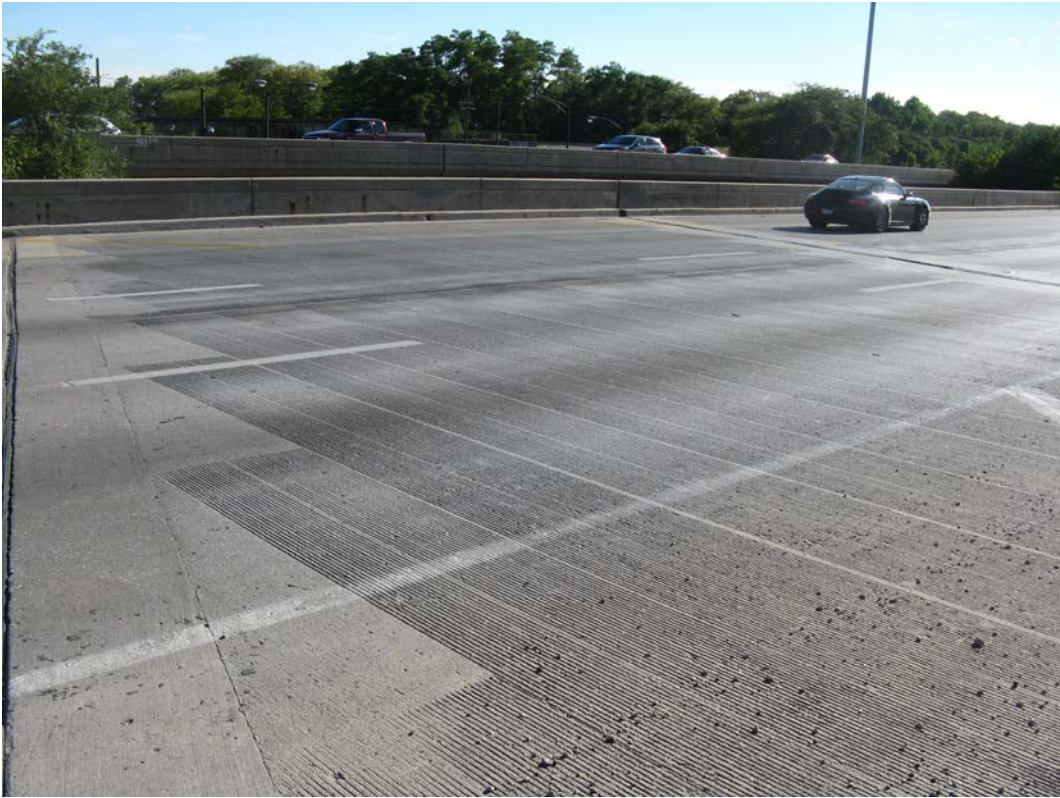
Photo 5 – Span 3, looking southwest
