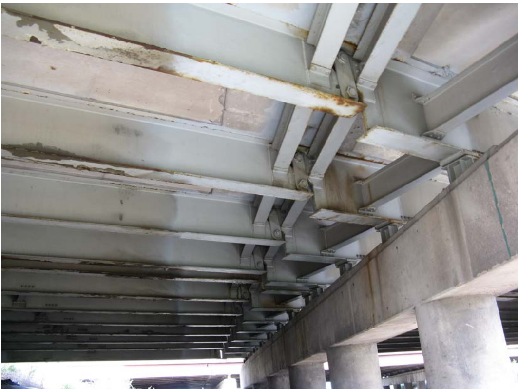
Photo 16 - Pin and link hangers in Span 1, looking north
