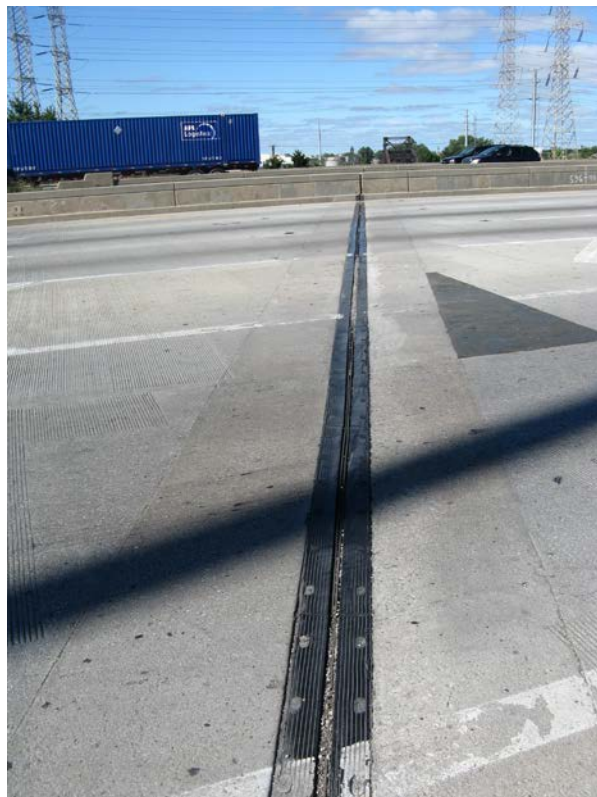
Photo 12 - Pier 1 joint, looking north
