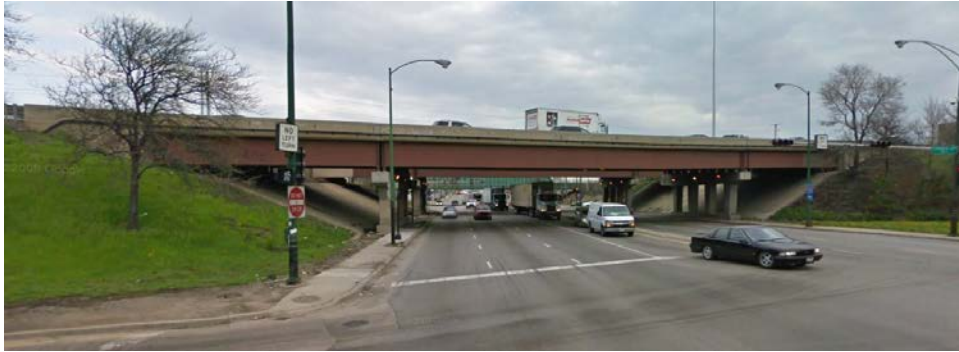
Figure 1. Elevation view, looking north. Photo from Google Streetview
