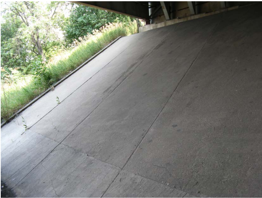
Photo 38 - North half of east slopewall, looking northeast
