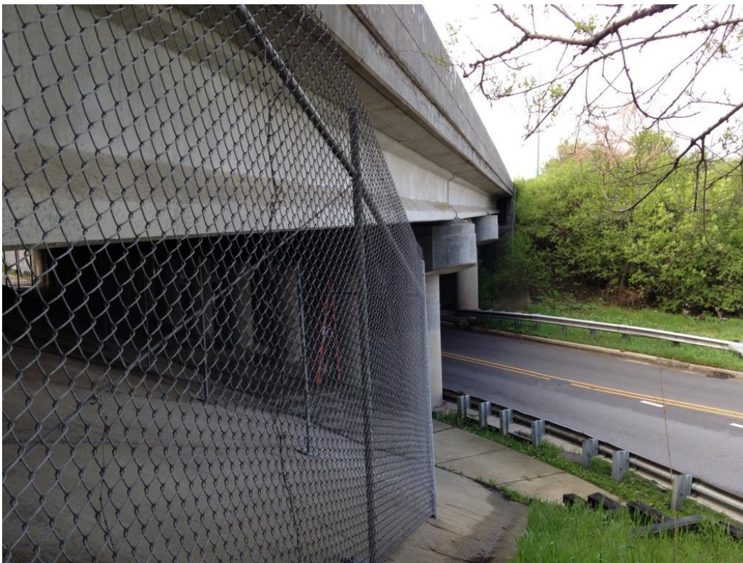
Photo 14: North side of structure looking southwest along fascia.
