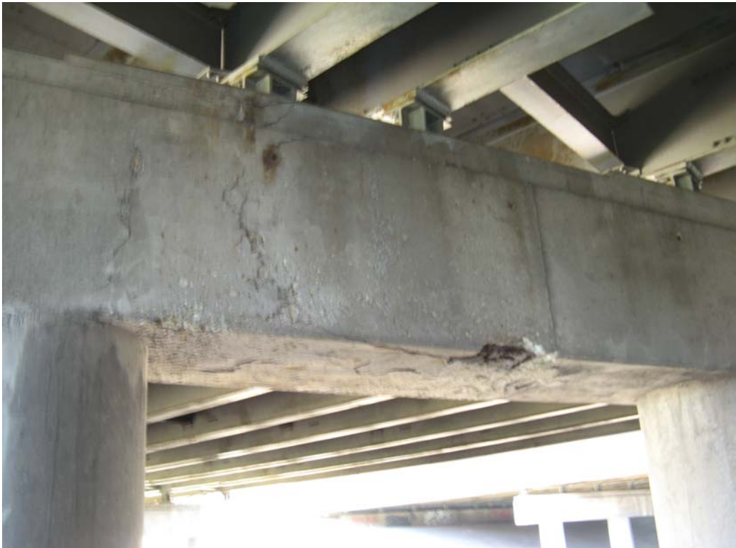
Photo 26 - Underside and face of Pier 1, looking east
