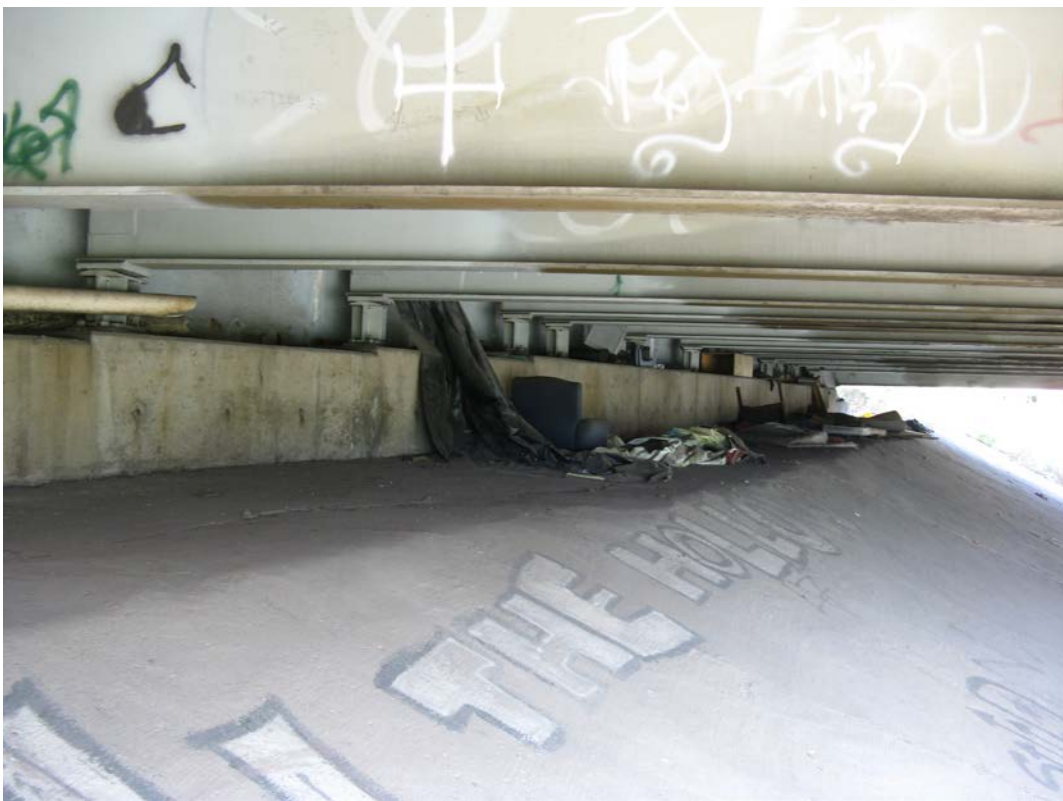
Photo 20 - West Abutment, looking northwest
