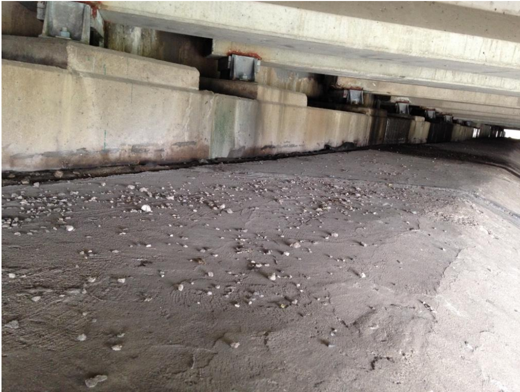
Photo 25; East abutment overall looking south along abutment from north end.
