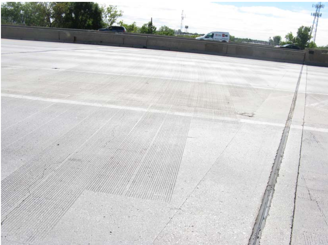
Photo 4 – Top of Deck in Span 1, looking south
