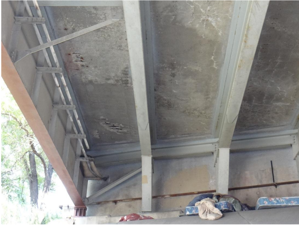
Figure 2. Typical view, deck soffit, northeast corner.
