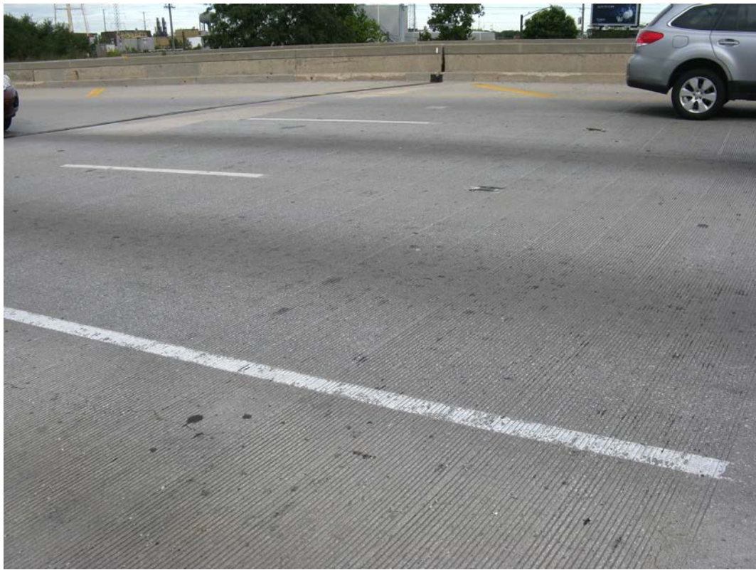
Photo 8 Span 3, looking northwest
