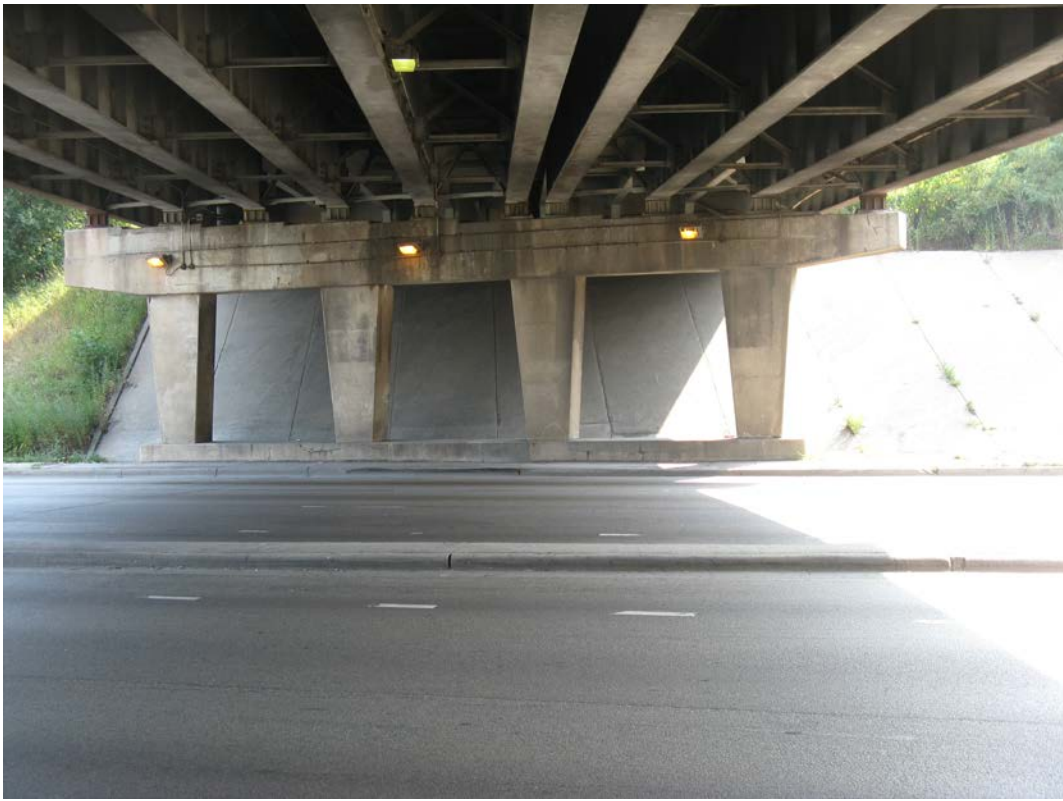
Photo 32 - East Pier, west face, looking east
