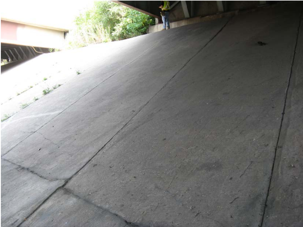
Photo 33 – East slopewall, north half, looking northeast
