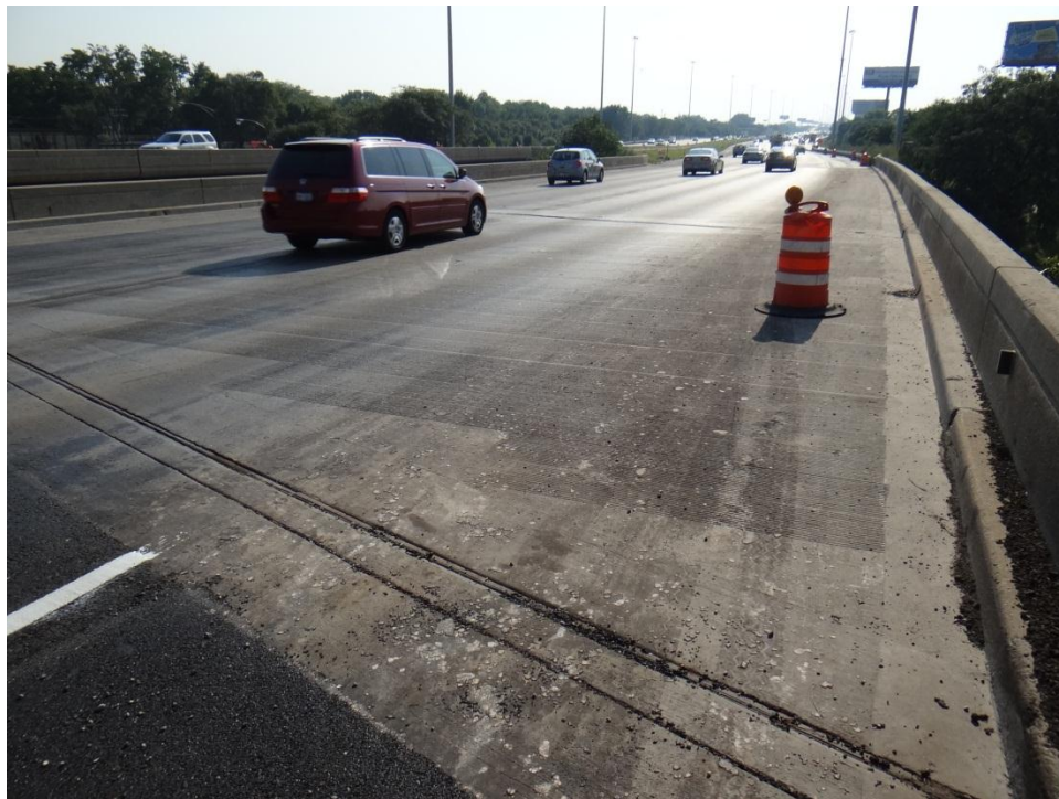
Figure 4. Typical view, deck top surface, looking southwest
