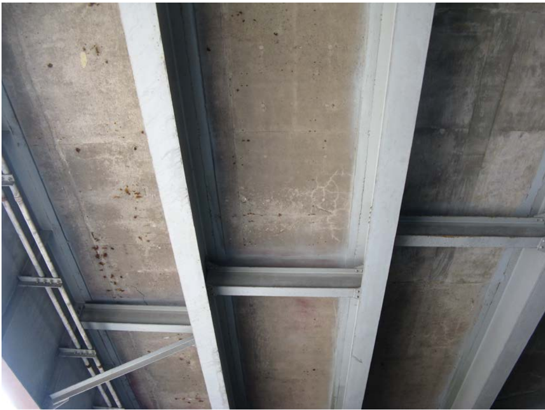
Photo 4 - Underside of deck, Span 1, south end, looking west
