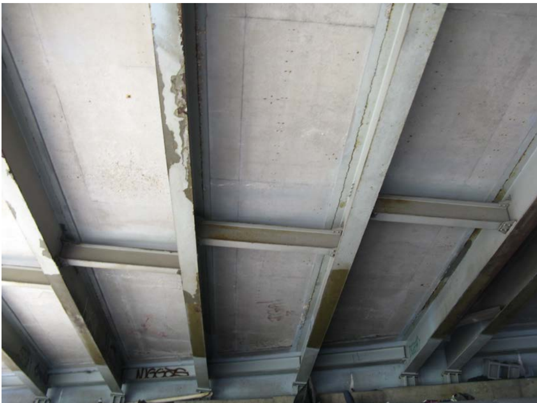
Photo 2 - Typical underside of Span 1, looking west
