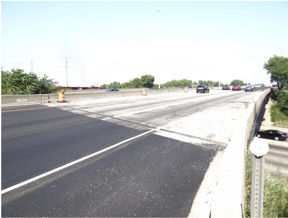
Figure 4. Typical view, deck top surface, looking northeast
