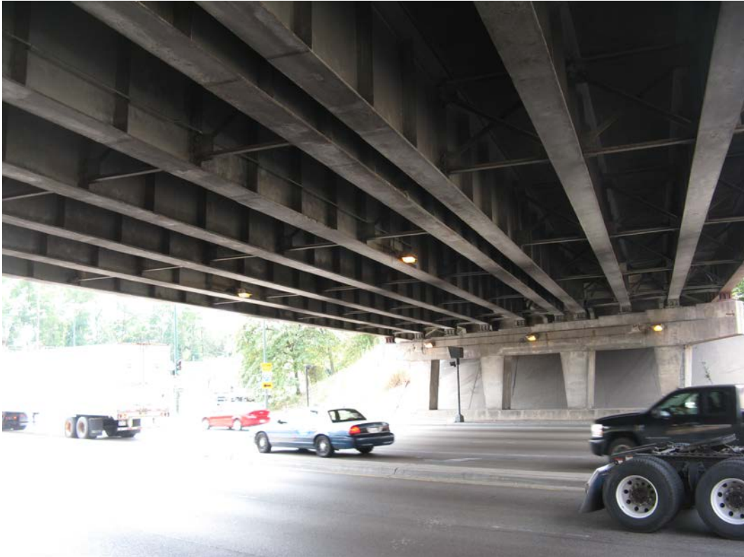
Photo 15 - Typical superstructure in Span 2, looking southwest
