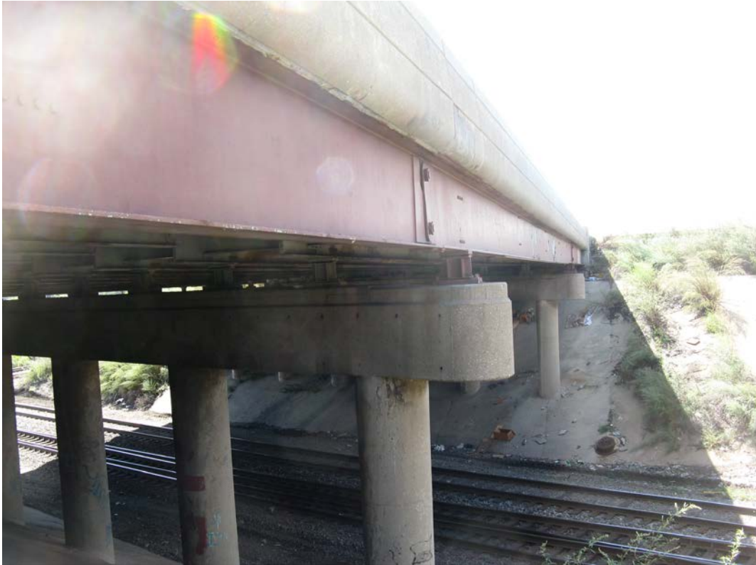
Photo 15 - North fascia, looking southwest
