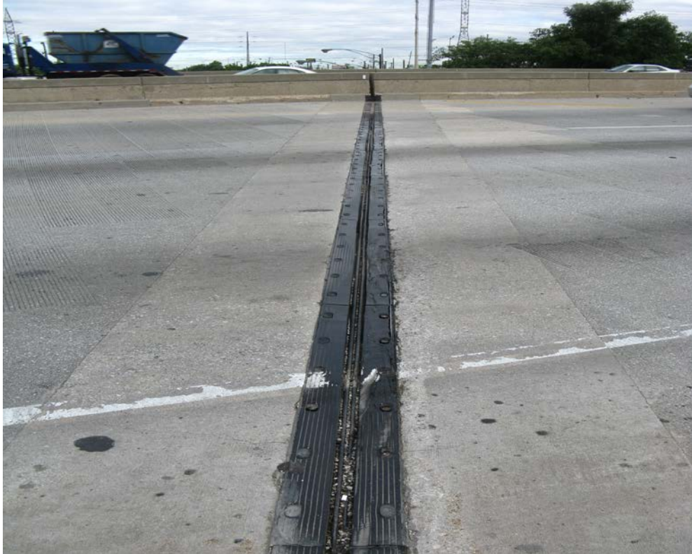
Photo 13 - Pier 2 joint, looking north
