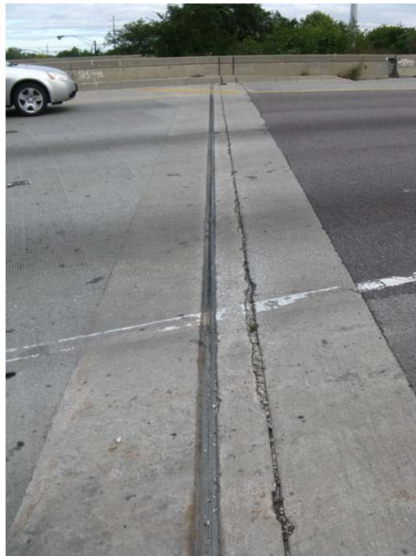
Photo 14 - East Abutment joint, looking north
