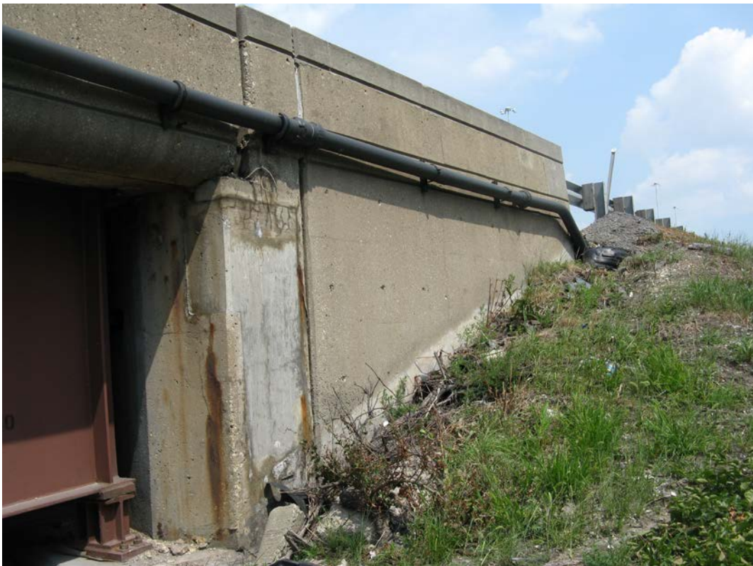
Photo 26 – Southeast wingwall, looking northeast
