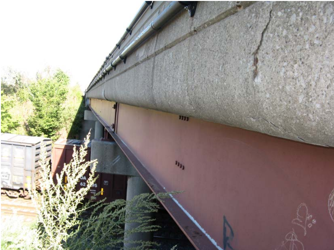
Photo 17 - North fascia, looking southeast
