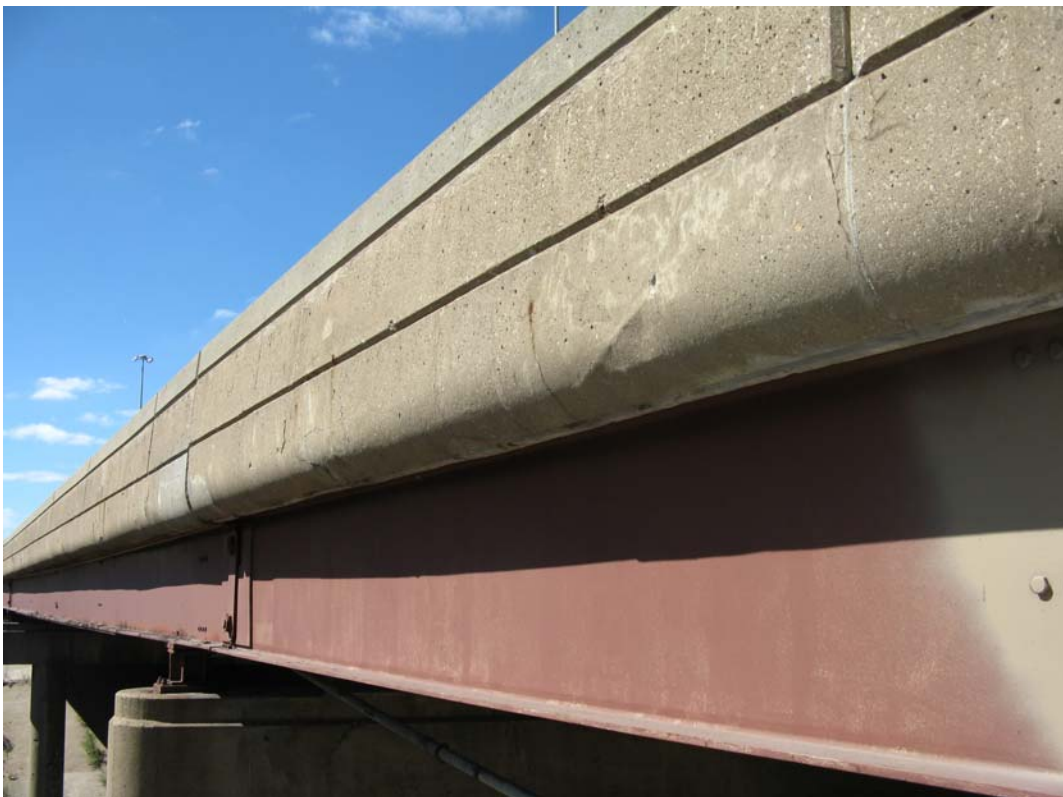
Photo 8 - South parapet in Span 3, looking northwest
