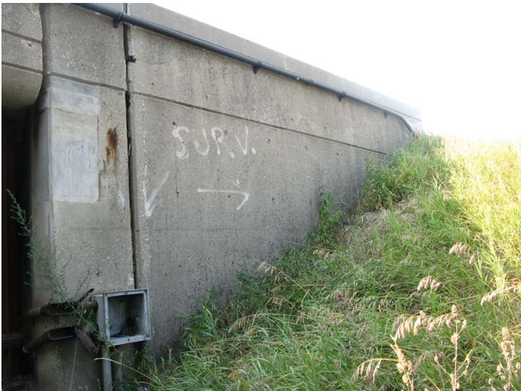
Photo 28 - Northwest Wingwall, looking southwest
