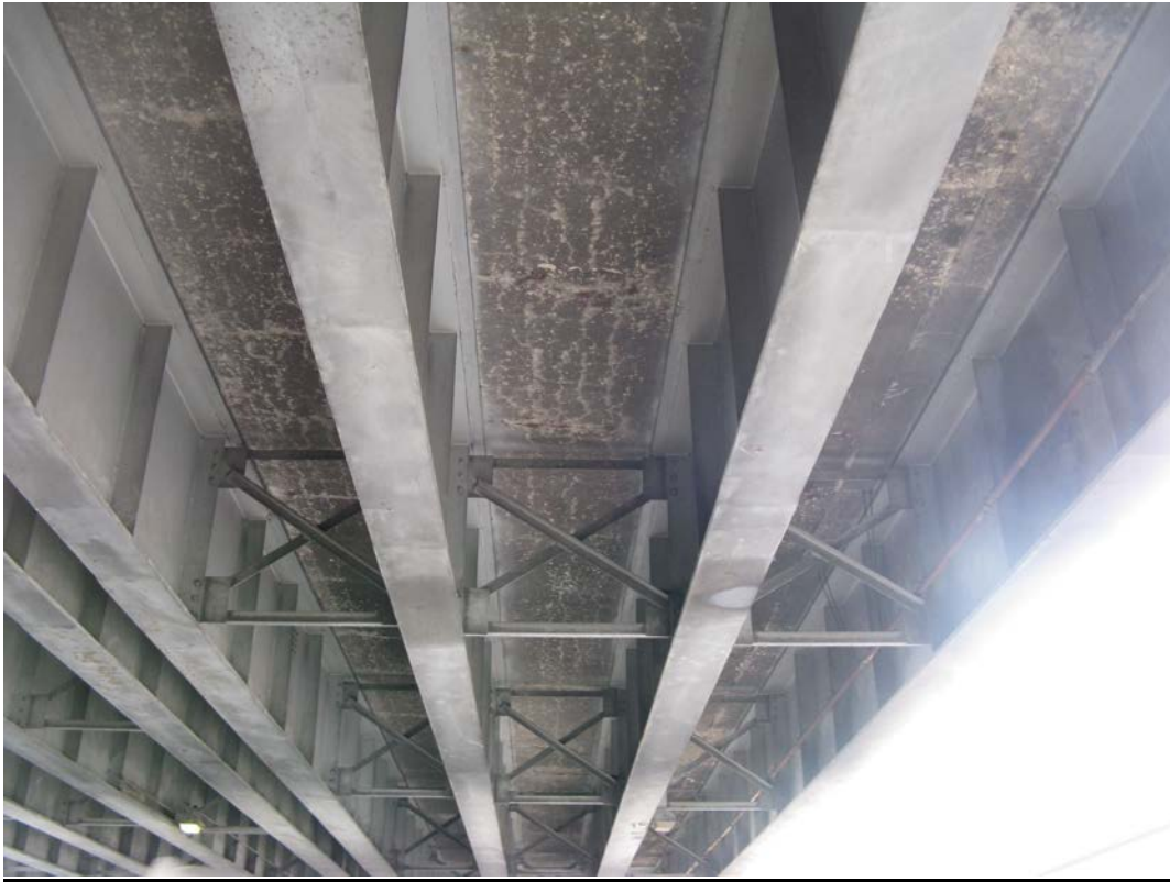
Photo 3 - Underside of Deck, Span 2, south end, looking east
