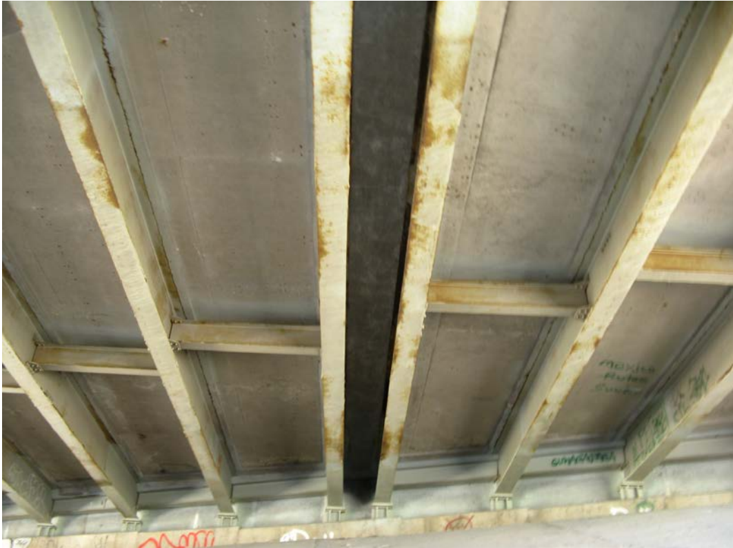
Photo 3 - Typical underside of Span 3, looking east
