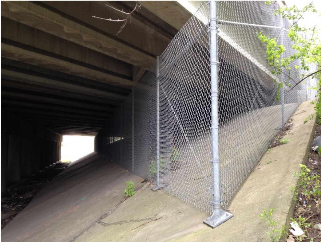
Photo 55: East slopewall looking south showing fence around east abutment.
