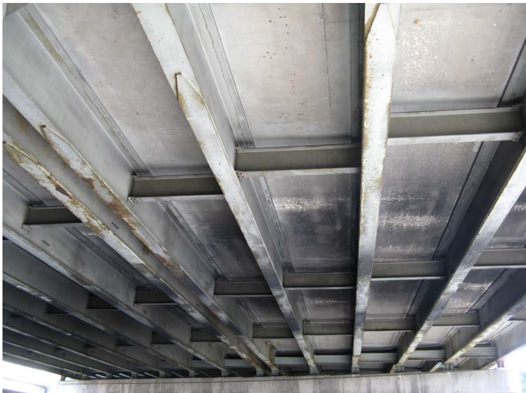
Photo 14 - Underside of Span 2 Beams, looking east
