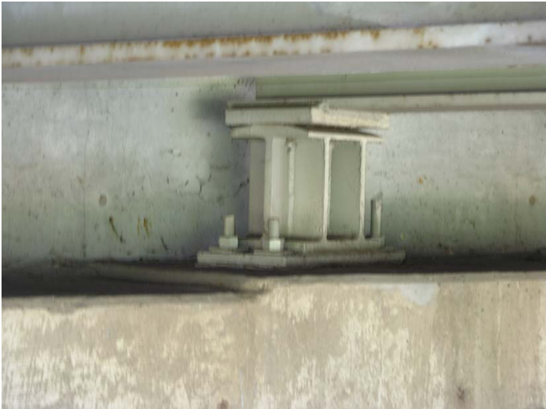
Photo 19 - Typical bearing at East Abutment, looking southeast
