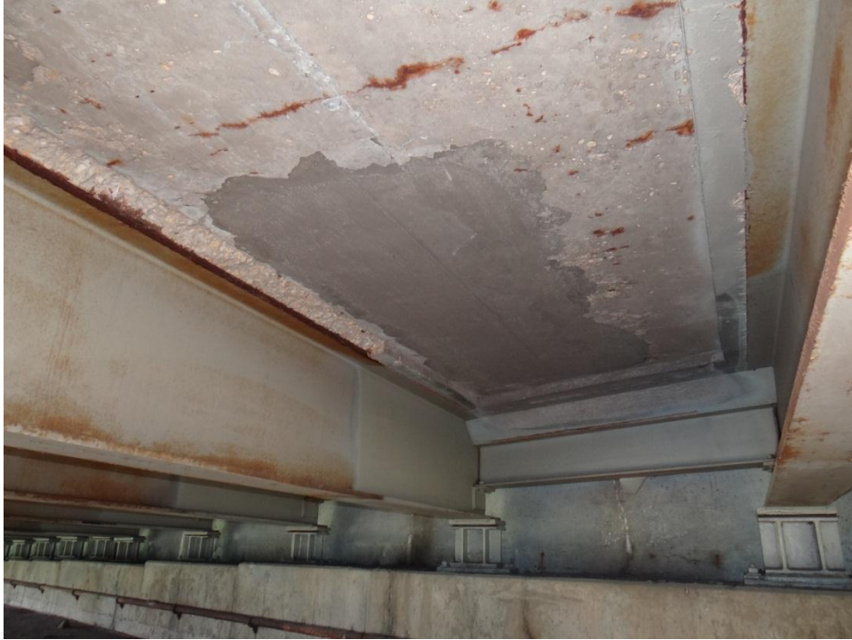
Figure 3. Typical view, deck soffit, looking east.
