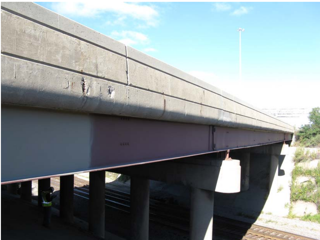
Photo 18 – Span South fascia, looking north
