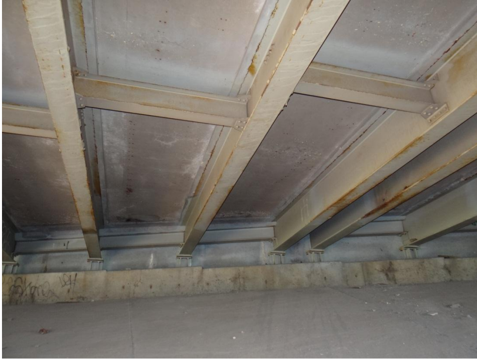
Figure 3. Typical view, deck soffit, looking east.
