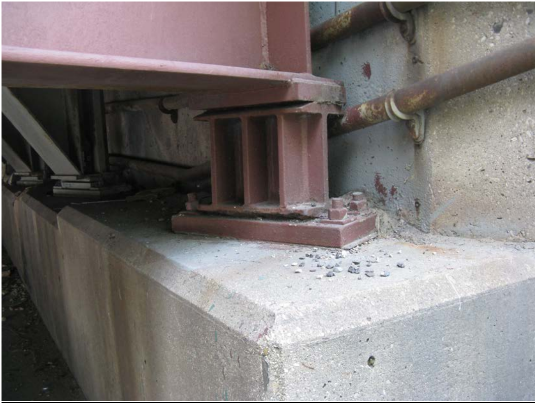
Photo 21 - Typical end beam bearing, beam 1 from north, West Abutment, looking southwest
