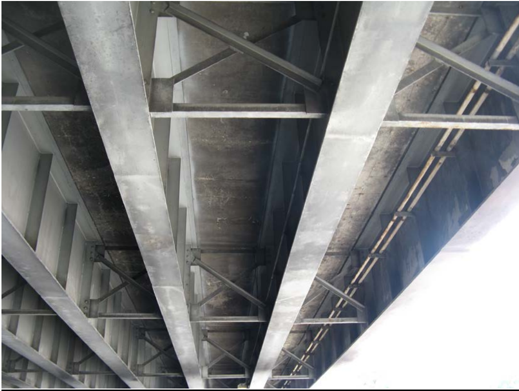
Photo 3 - Underside of Span 2, south end, looking east
