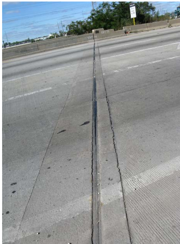
Photo 10 - East Abutment joint, looking north
