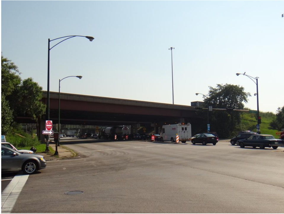
Figure 1. Elevation view, looking south
