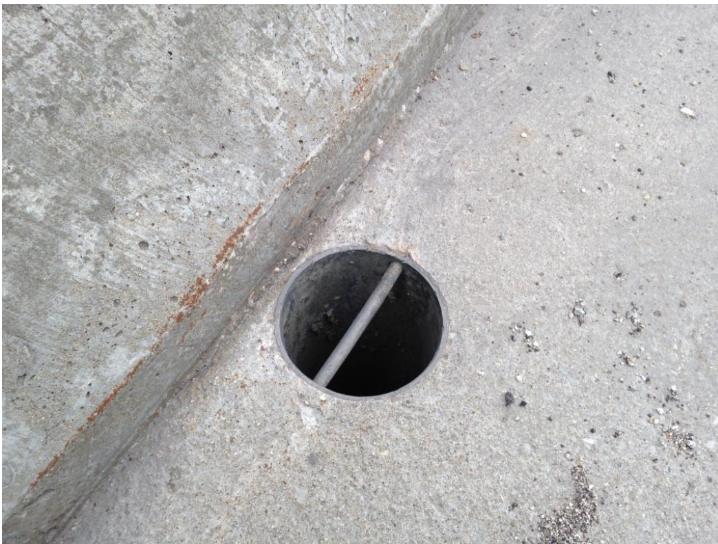
Photo 54: Top of deck showing deck drain free of debris (typ.).
