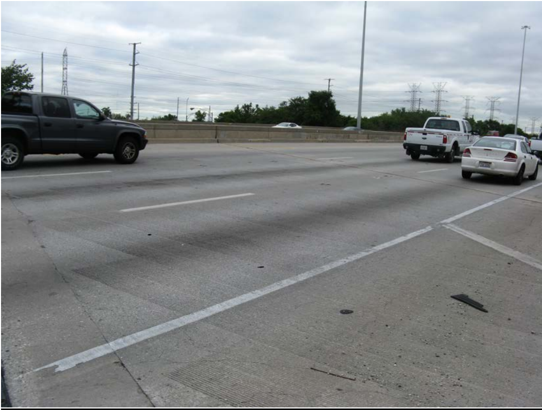
Photo 5 – Span 1, looking northeast
