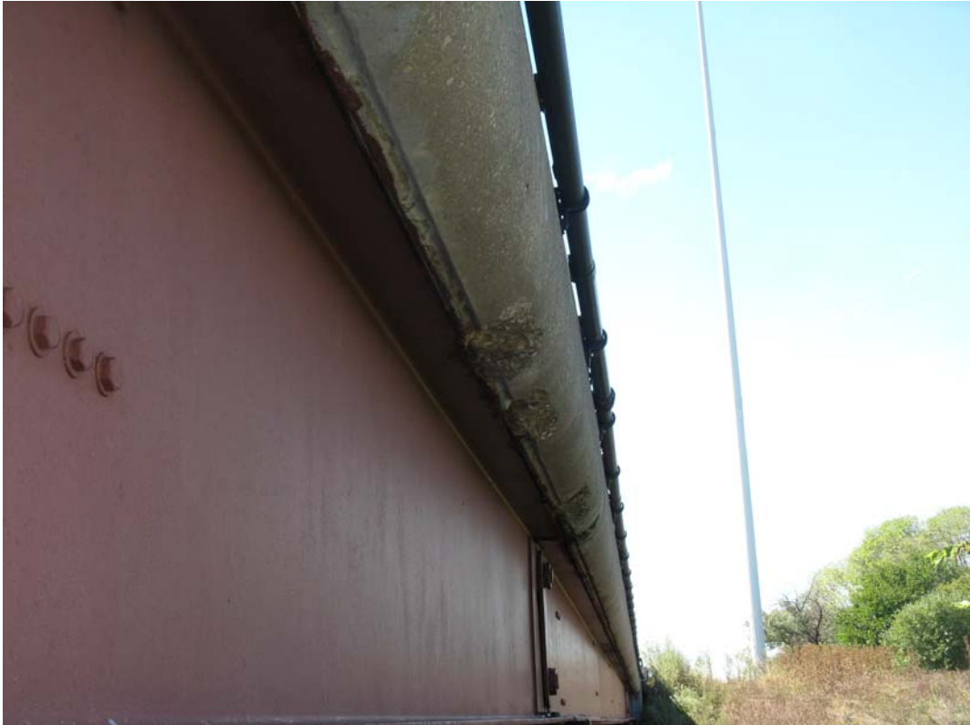
Photo 7 - North parapet in Span 1, looking west
