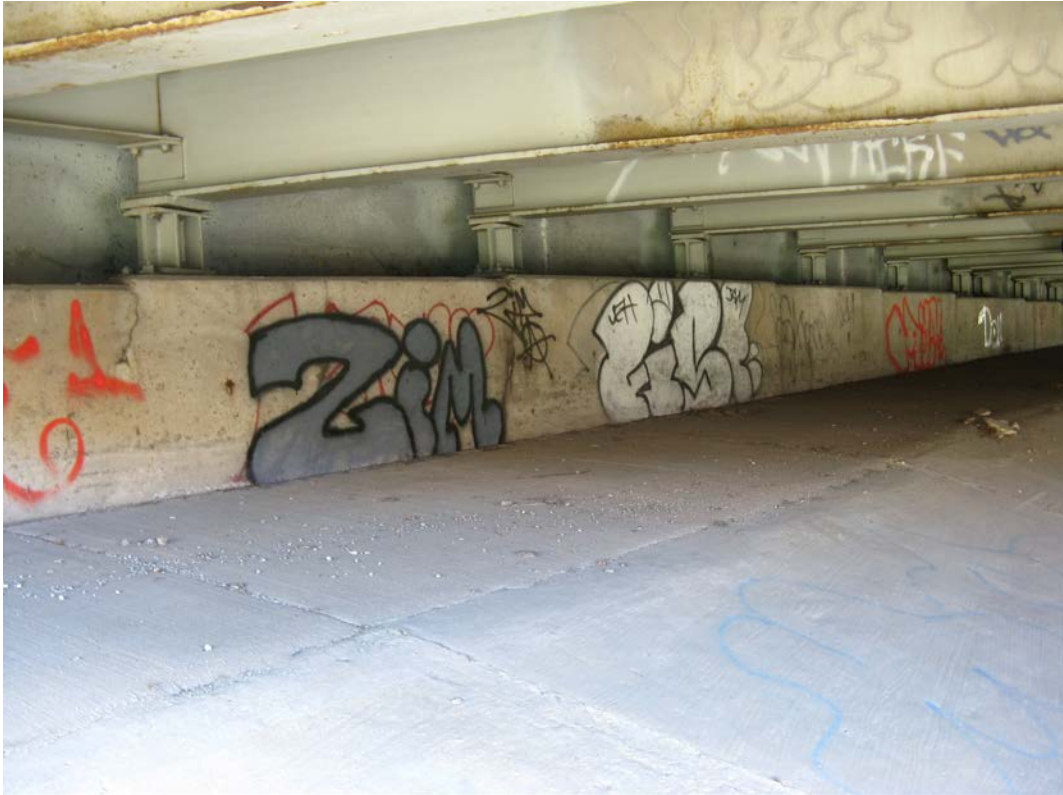
Photo 21 - East Abutment, looking southeast
