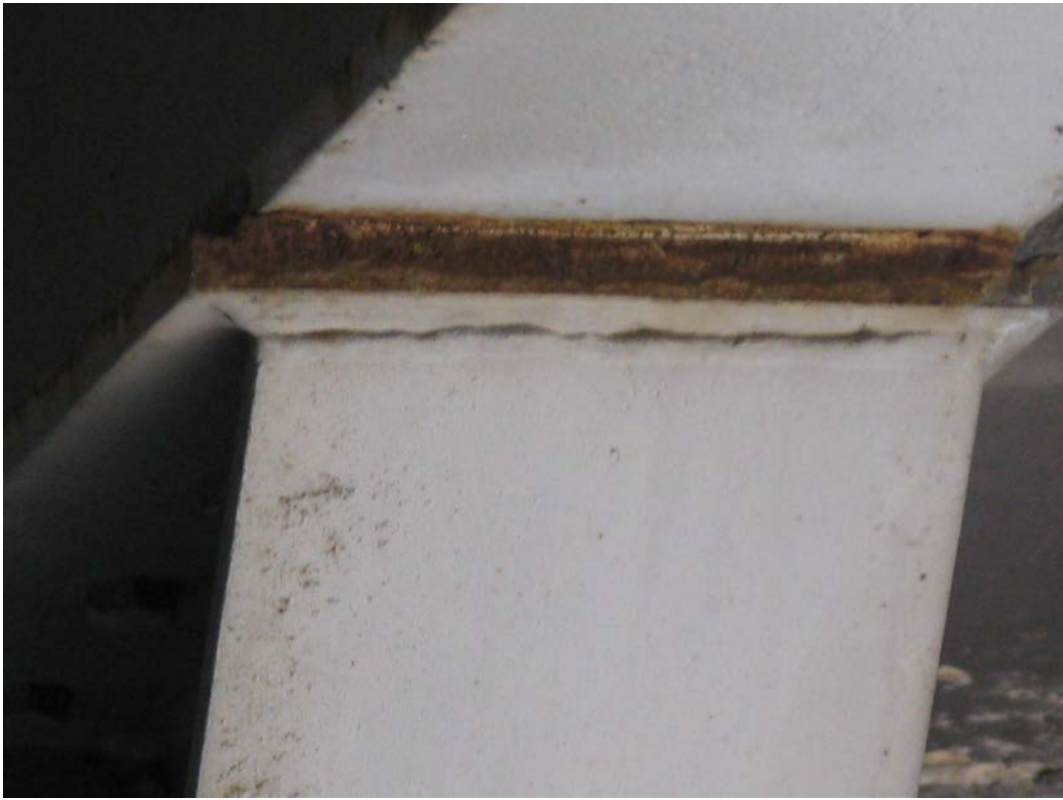
Photo 13 - Close up of photo 12
