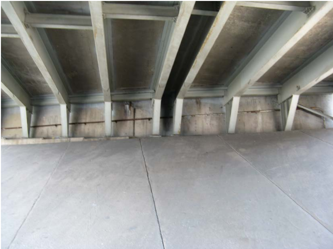
Photo 22 - East Abutment, looking east
