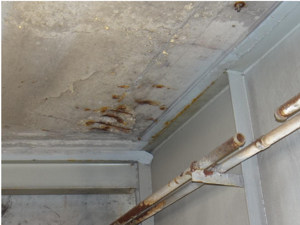
Figure 2. Typical view, deck soffit, southeast corner.
