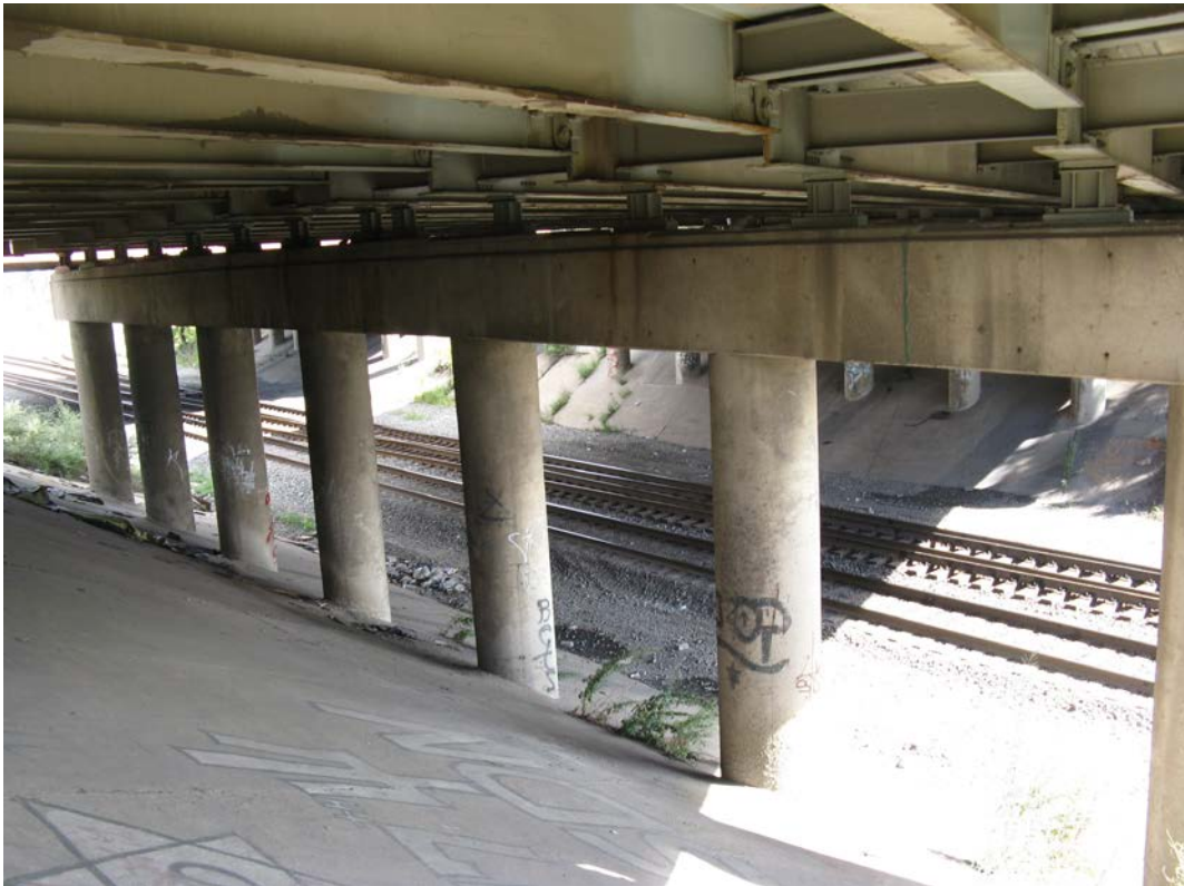
Photo 22 – Pier 1, looking northeast
