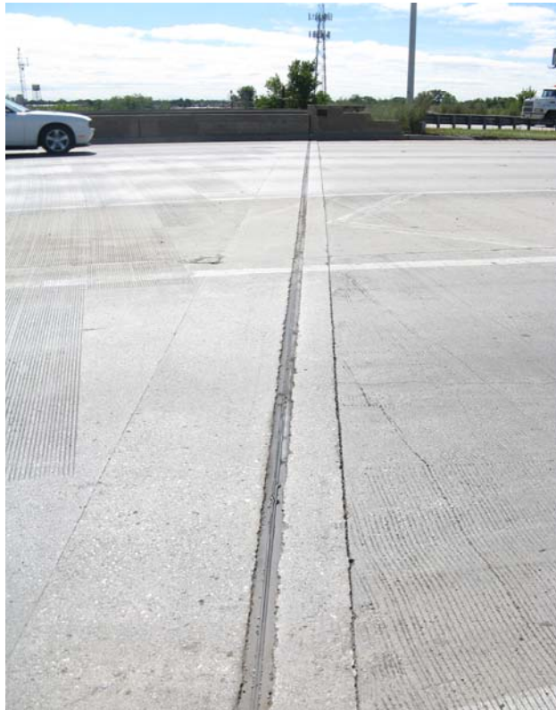
Photo 10 - West Abutment joint, looking south
