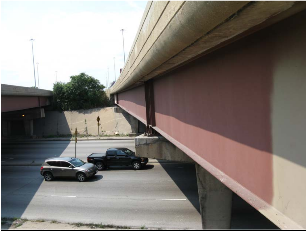
Photo 17 - South fascia beam, looking west
