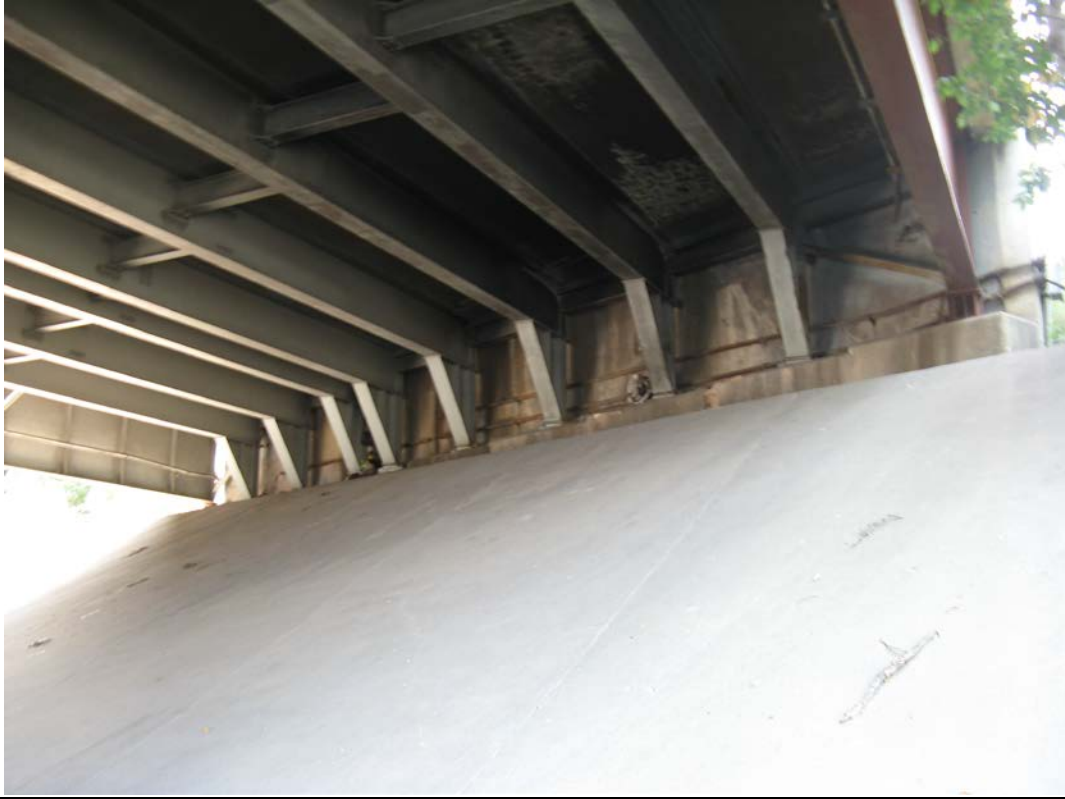
Photo 23 - West Abutment, looking southwest
