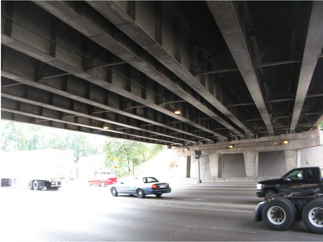
Photo 15 - Typical superstructure in Span 2, looking southwest
