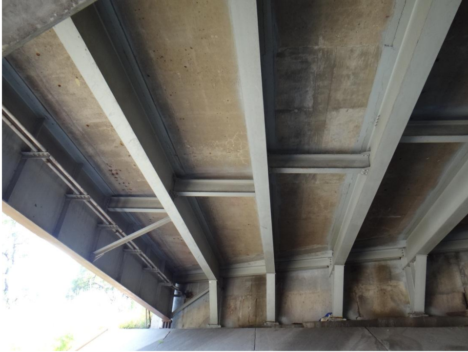
Figure 3. Typical view, deck soffit, west end.
