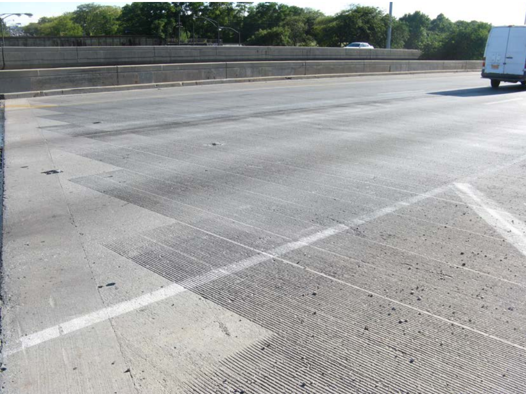
Photo 6 – Span 2, looking southwest
