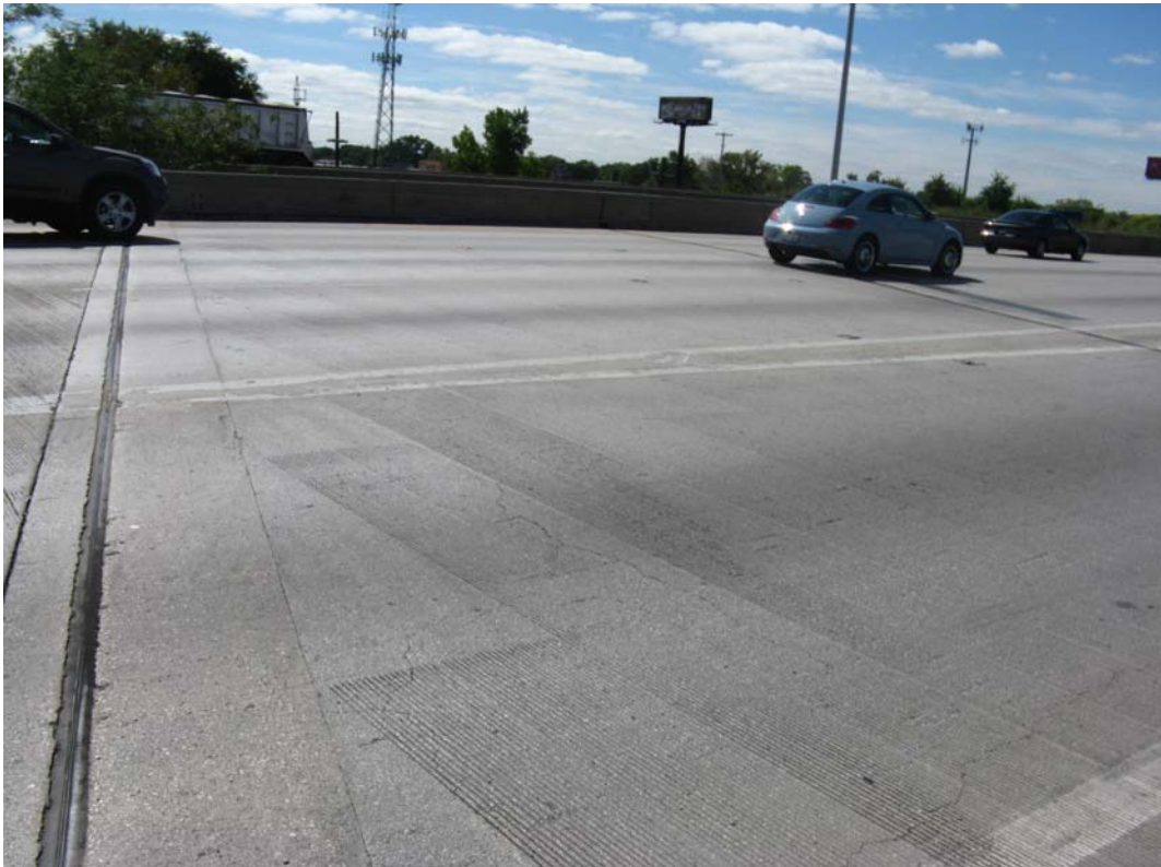
Photo 6 – Top of Deck Span 1, looking southwest
