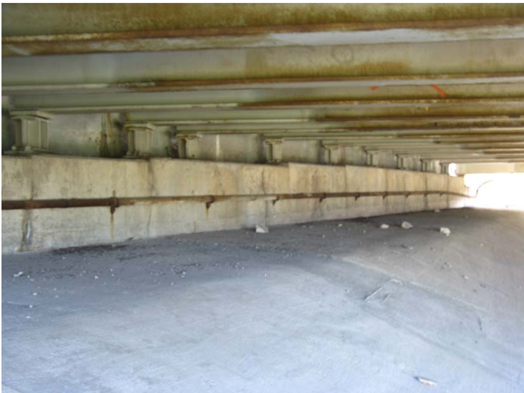
Photo 22 - East Abutment, looking southeast
