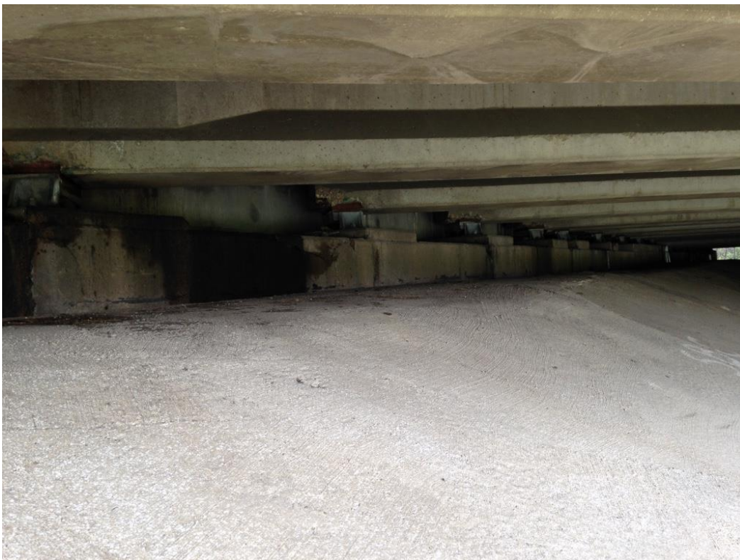
Photo 26: West abutment overall looking north along abutment from median.
