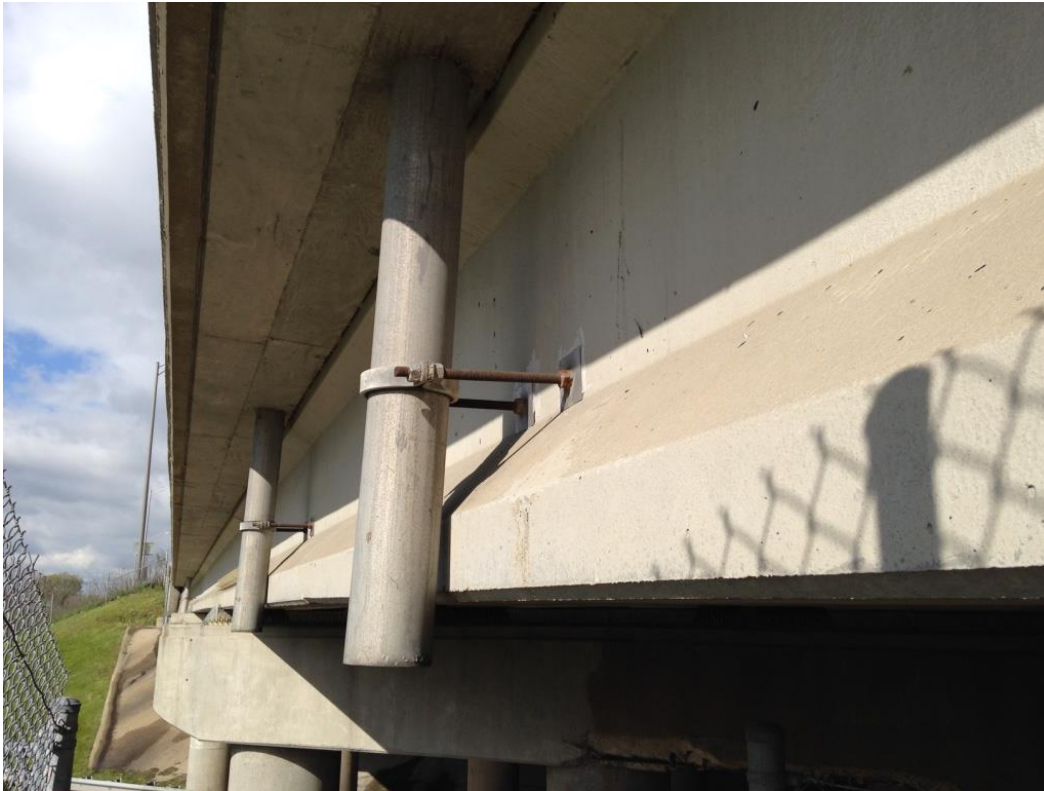
Photo 53: South end of bridge looking west showing deck drain down spouts.
