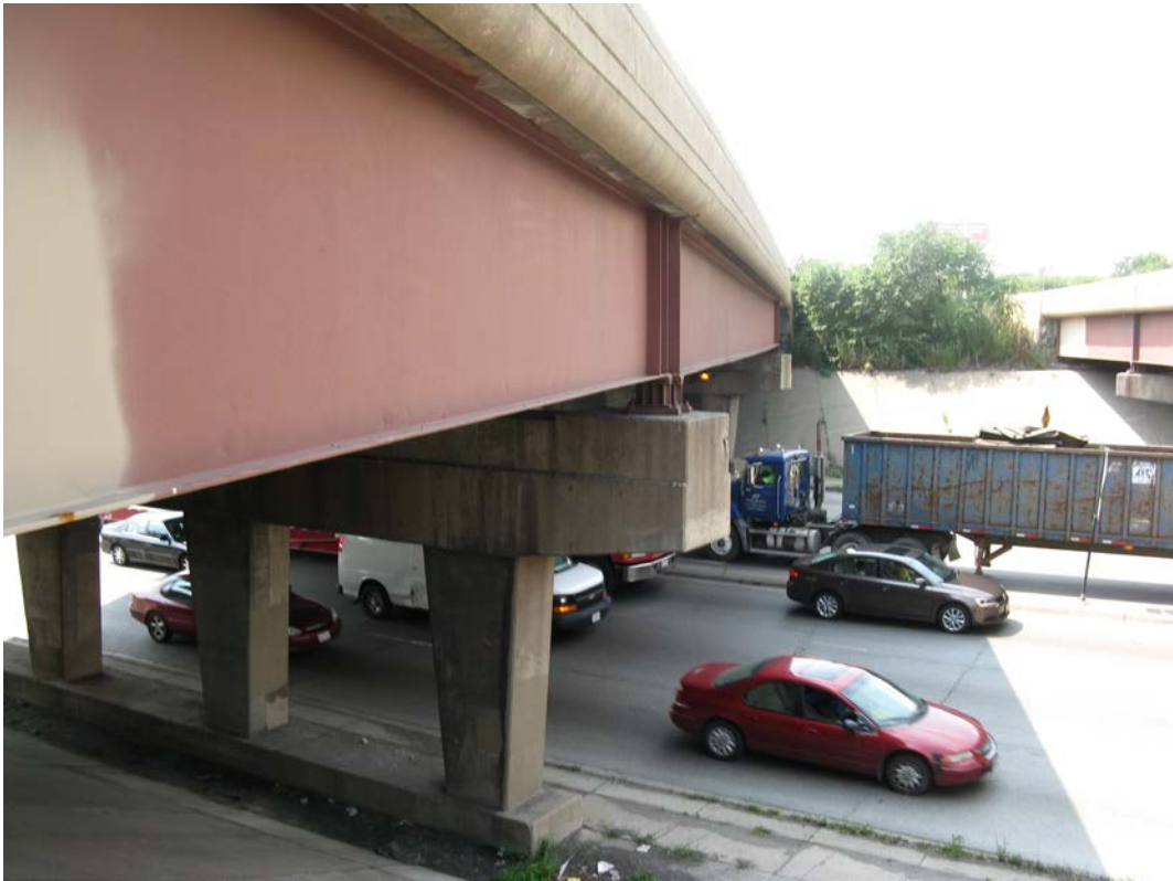
Photo 19 - North Fascia Beam, looking east
