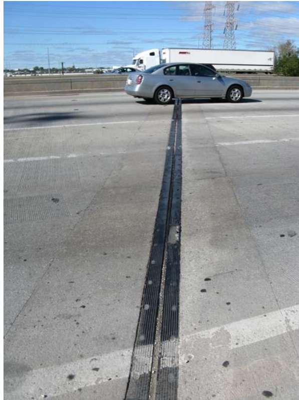
Photo 11 - Pier 2 joint, looking north
