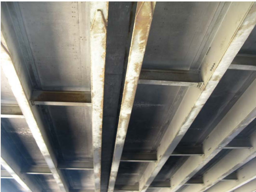
Photo 4 - Typical underside of Span 2, looking west
