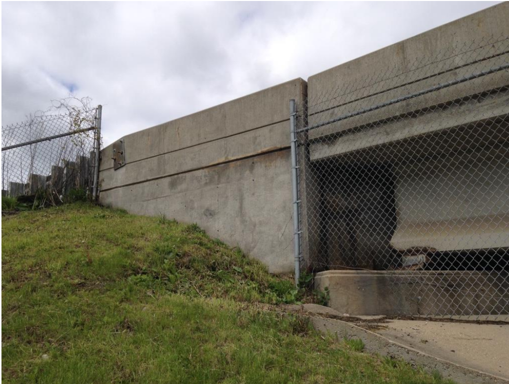
Photo 41: Southwest wingwall overall (typ.).
