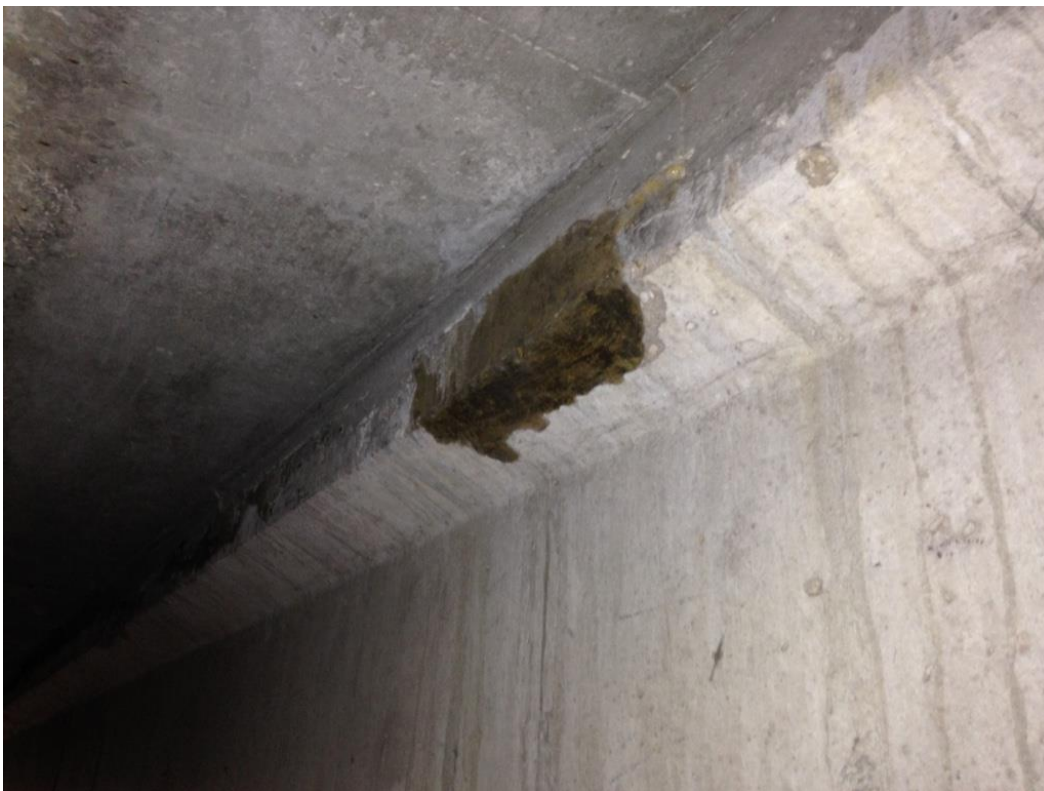
Photo 8: South face of girder 16 in span 3 showing previously patched area intact.
