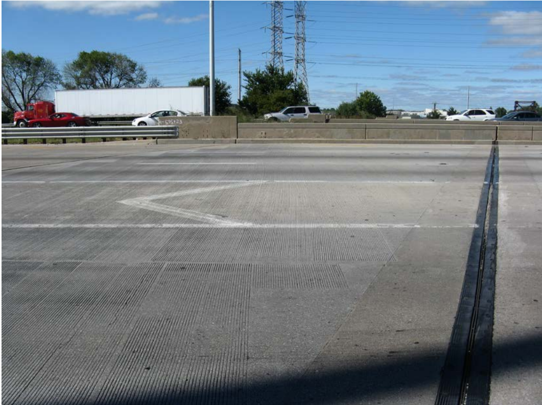
Photo 7 – Top of Deck in Span 1, looking northwest
