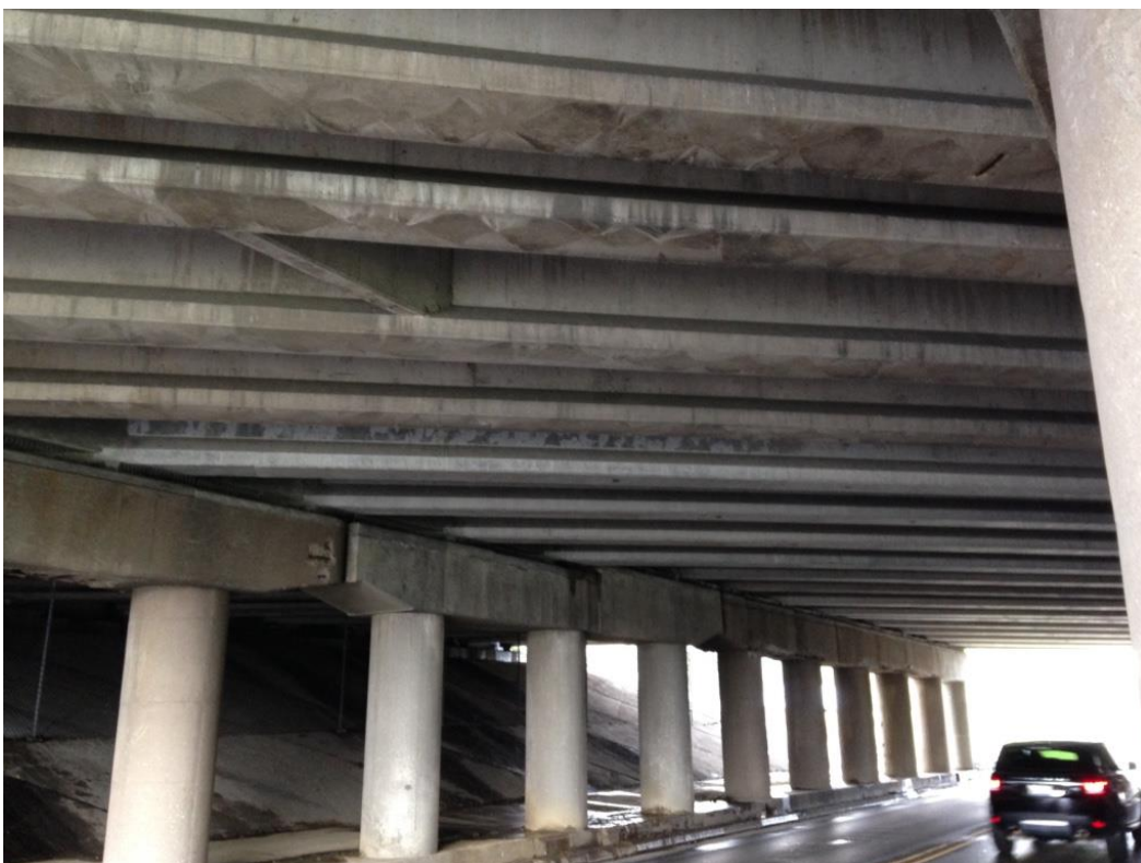
Photo 4: Span 2 overall looking south.
