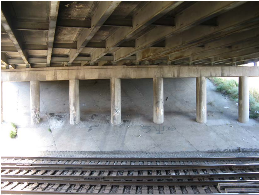
Photo 24 - Pier 1, looking west
