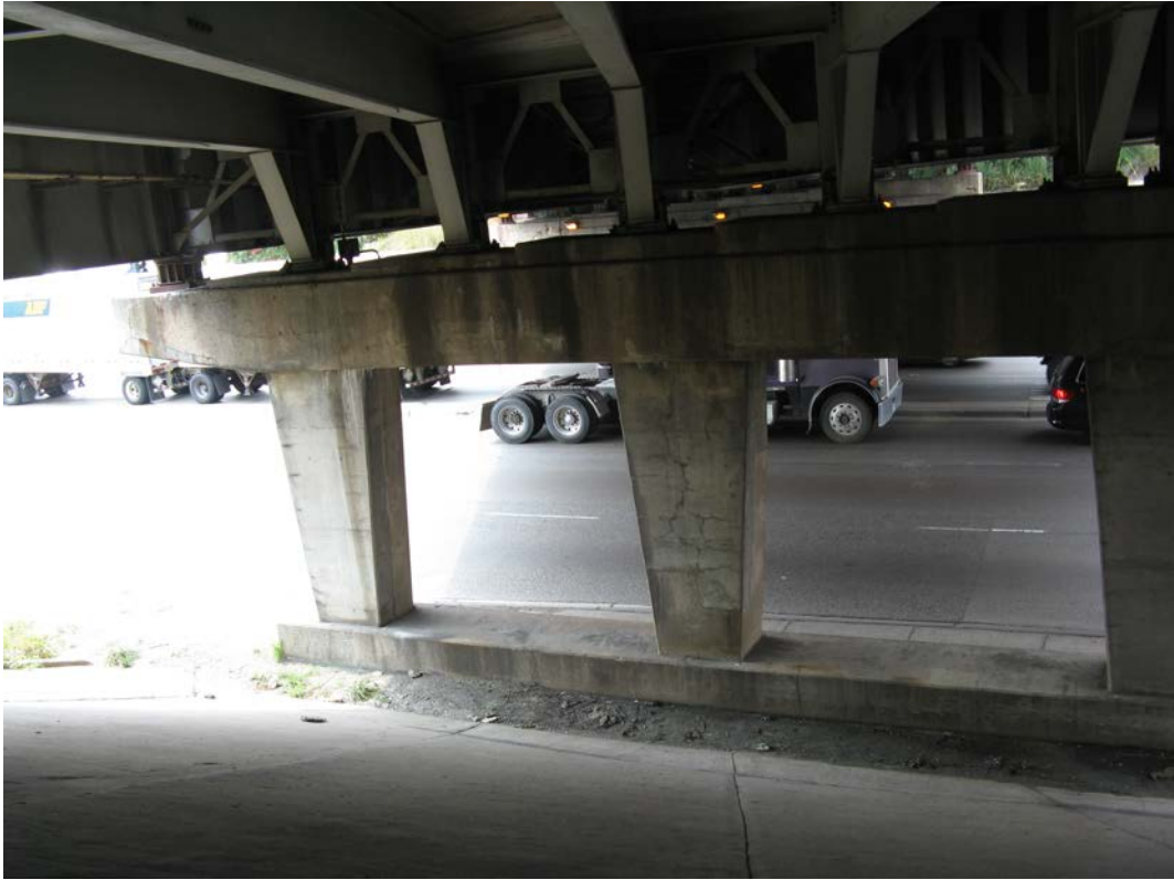
Photo 27 - East Pier, looking southwest
