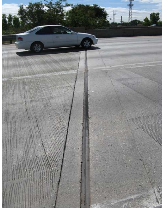
Photo 13 - East Abutment joint, looking south
