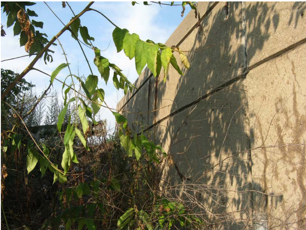
Photo 30 – Southwest wingwall, looking west
