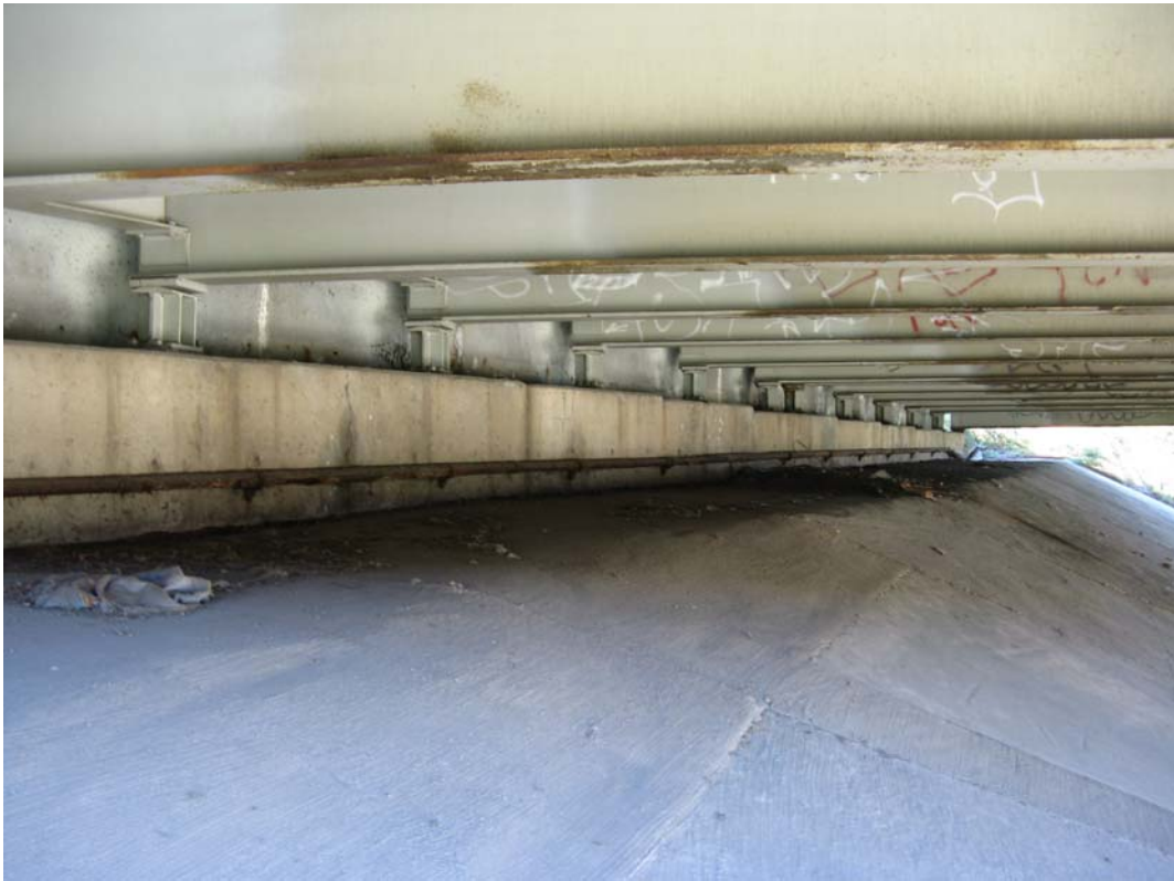
Photo 23 - West Abutment, looking northwest
