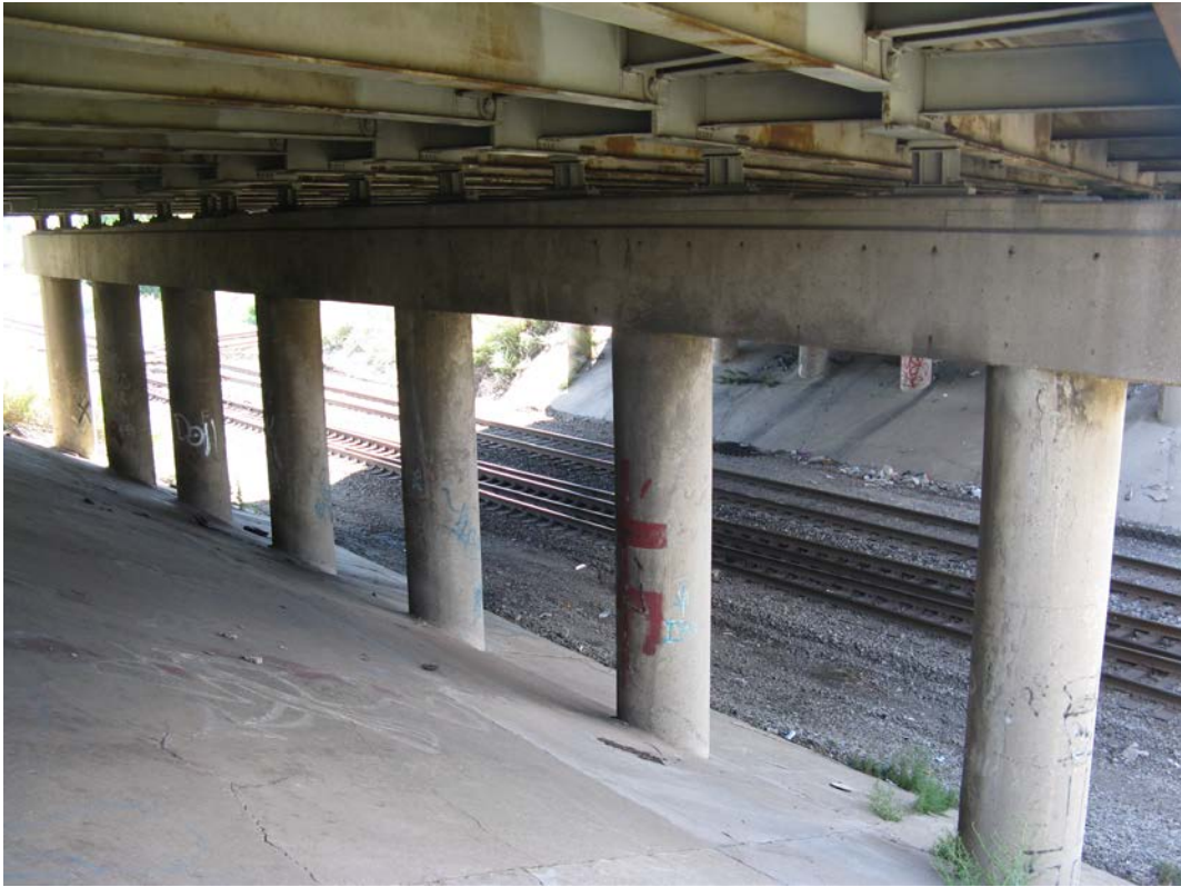
Photo 25 – Pier 2, looking southwest
