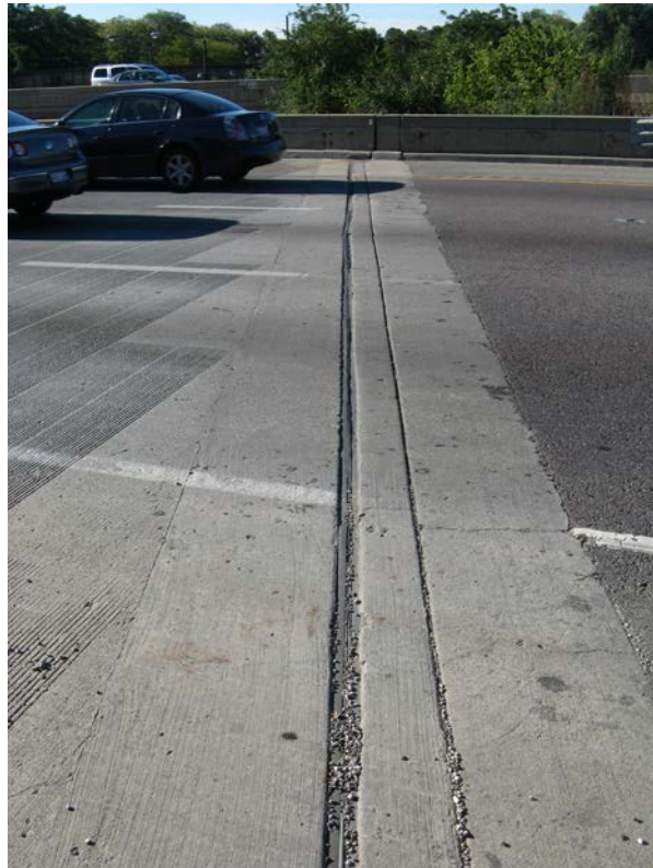
Photo 8 - East Abutment joint, looking south
