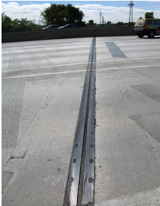
Photo 12 – Pier 2 joint, looking south
