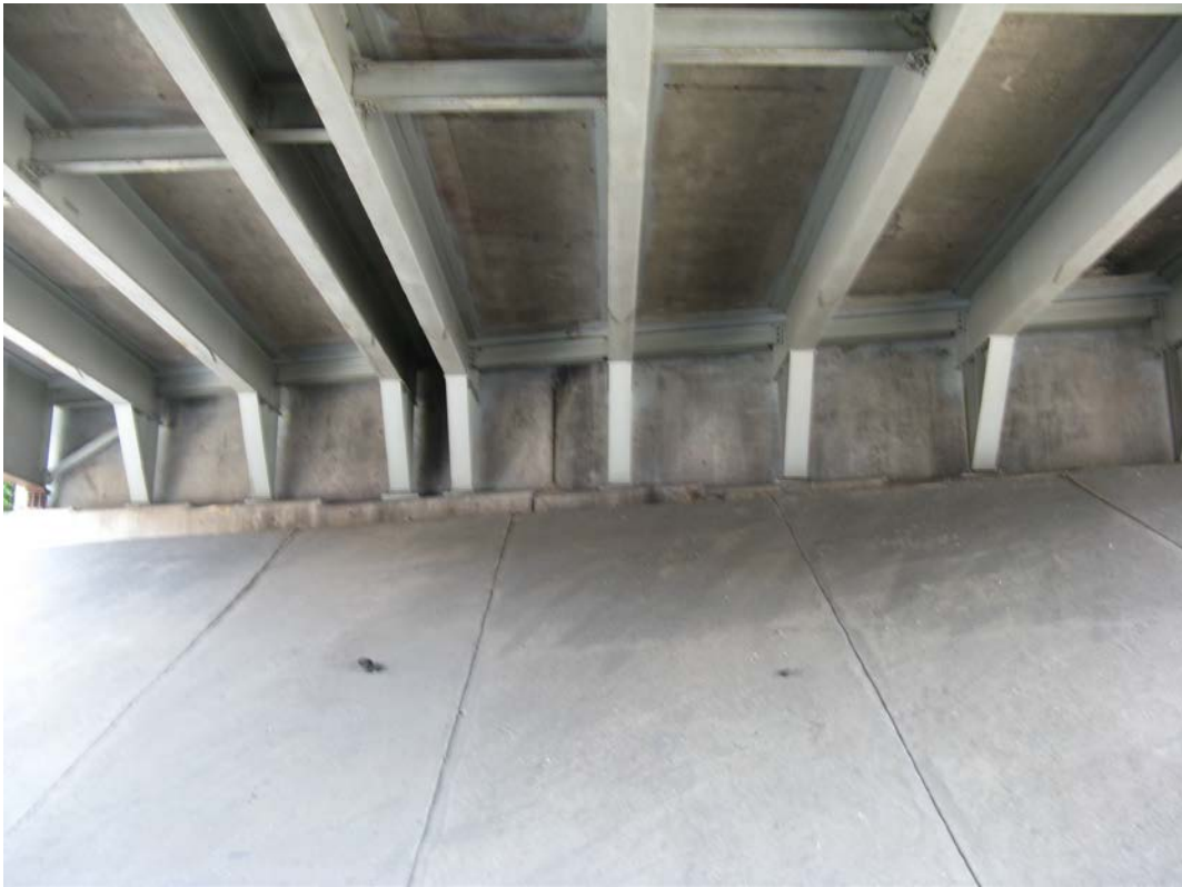
Photo 23 - East Abutment, looking east
