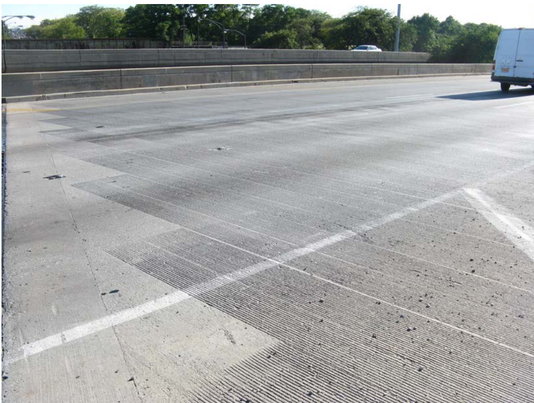
Photo 6 – Span 2, looking southwest
