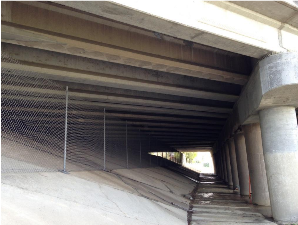
Photo 5: Span 3 overall looking south showing fence around west abutment.
