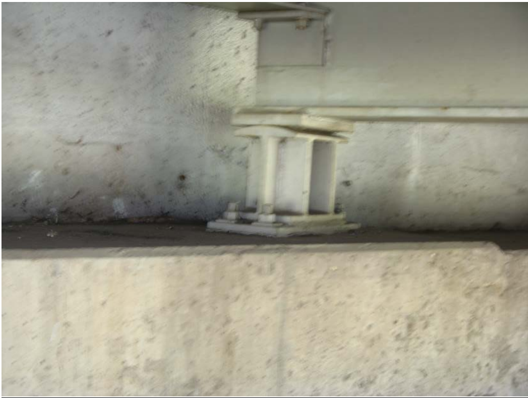
Photo 19 - Typical bearing at East Abutment, looking southeast
