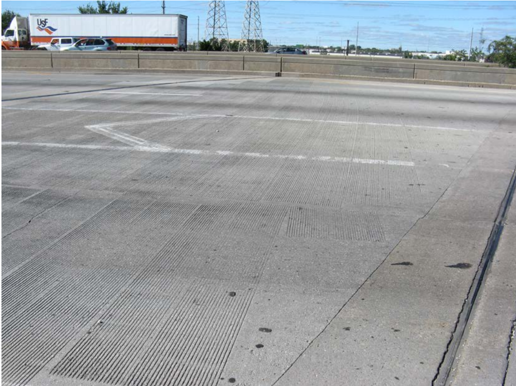
Photo 5 – Top of Deck in Span 3, looking northwest
