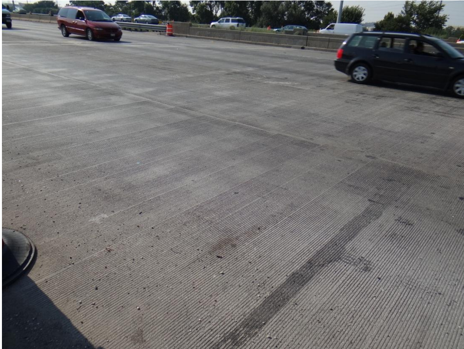
Figure 4. Typical view, deck top surface, looking northwest
