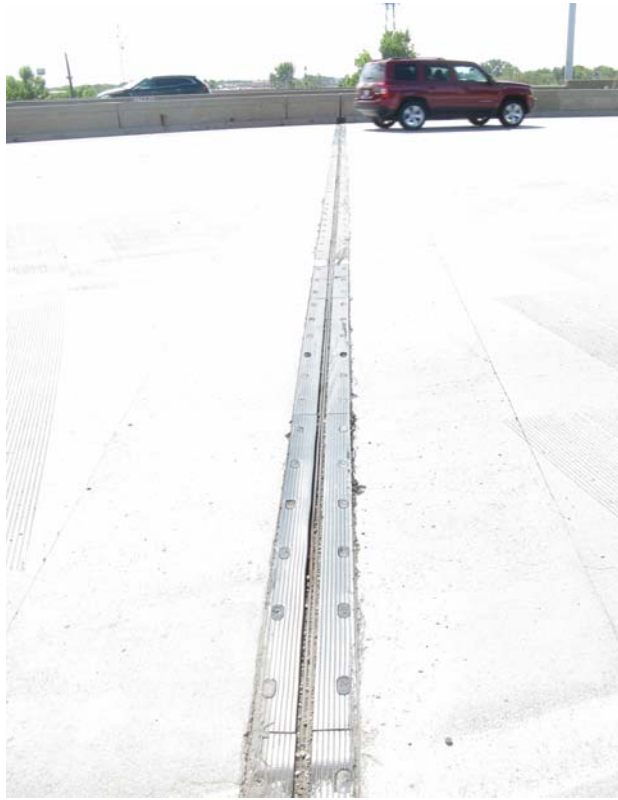
Photo 11 – Pier 1 joint, looking south
