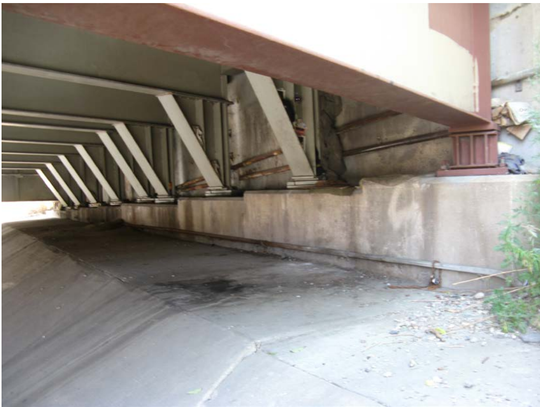
Photo 24 - West Abutment, looking southwest
