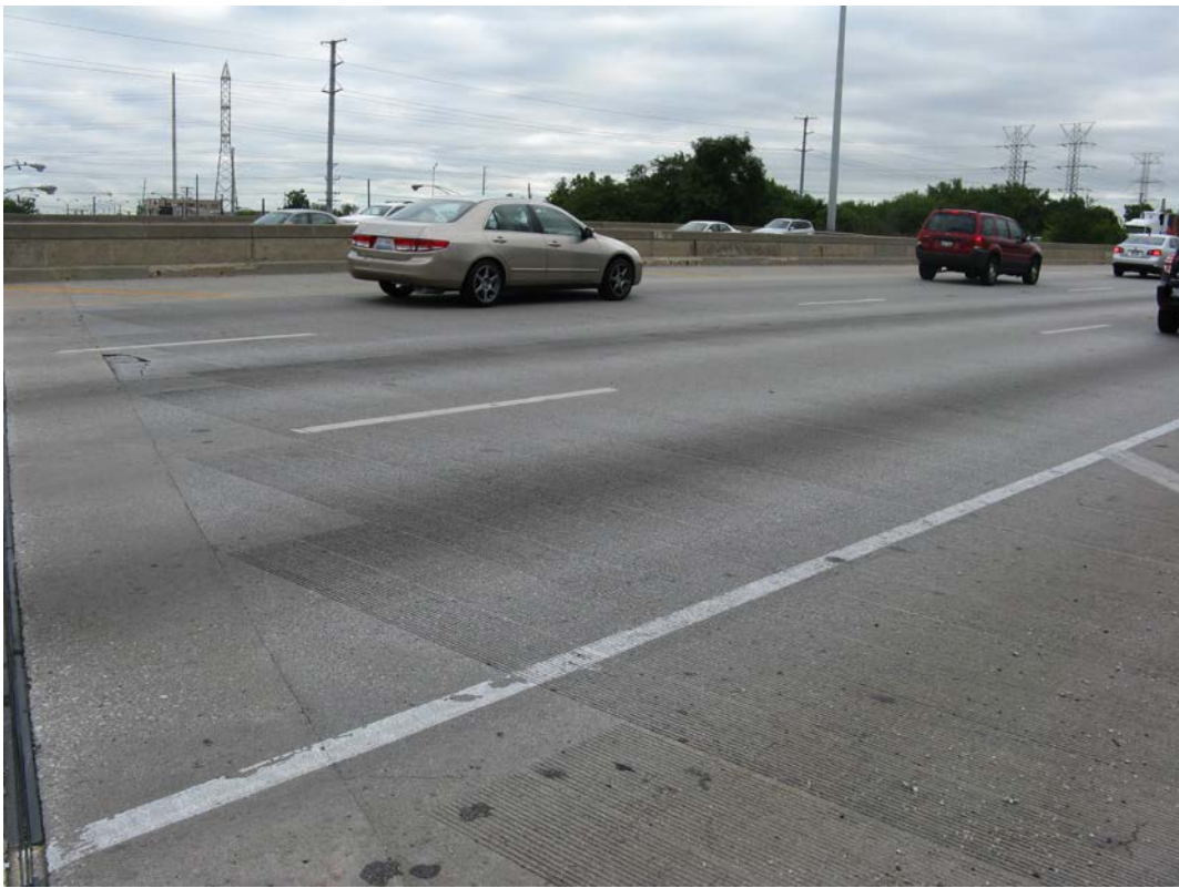
Photo 6 – Span 2, looking northeast
