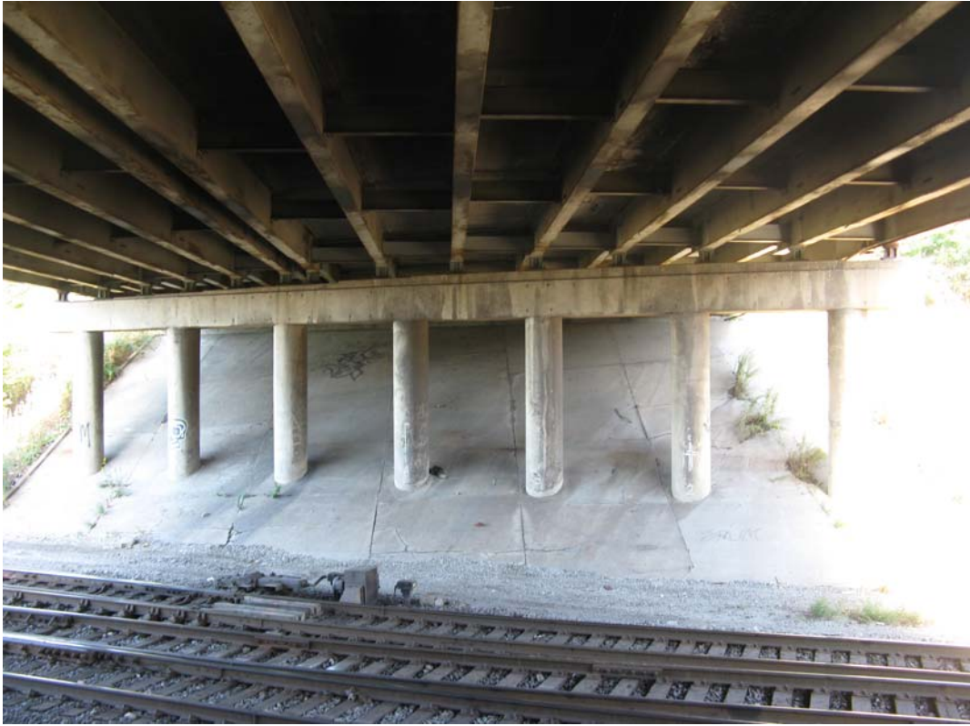
Photo 25 – Pier 2, looking east
