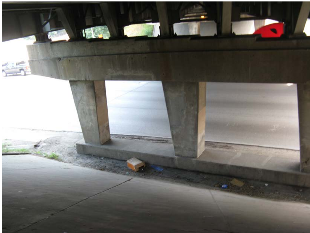
Photo 36 - West Pier, west face, north end, looking northeast
