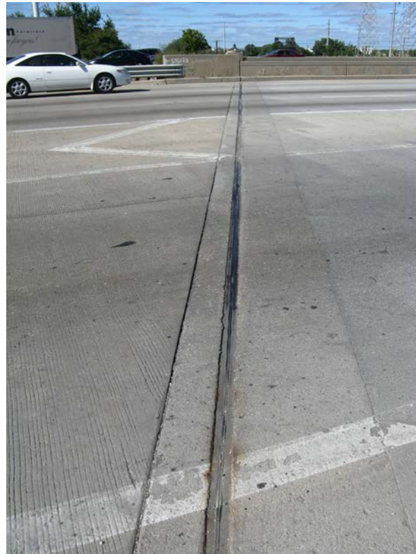
Photo 13 - West Abutment joint, looking north
