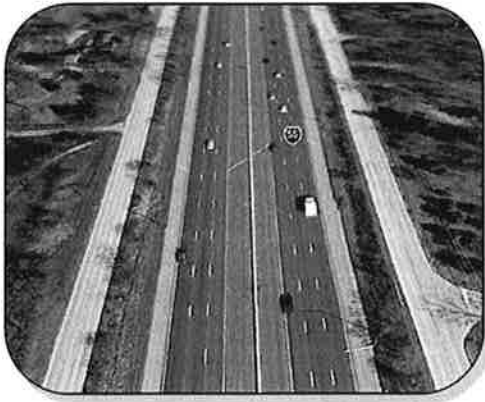
Figure 1 – I-55 east of I-355 to west of Harlem Avenue
