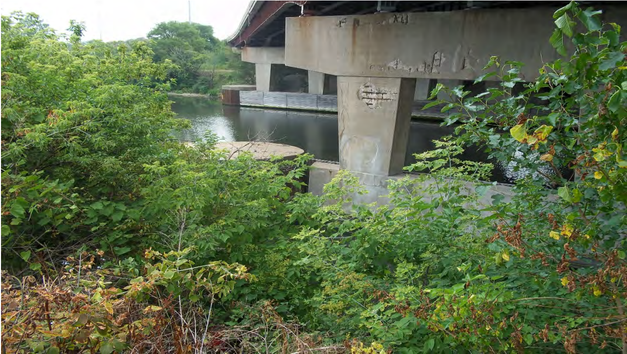
US-0. Looking East at upstream face of I-55 from Northwest bank
