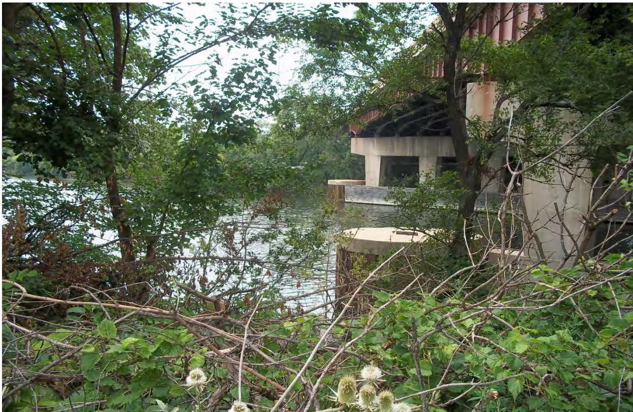
DS-0 Looking West at downstream face of I-55 from Southeast bank
