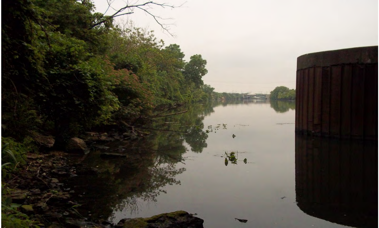
US-0 Looking Northeast from Northwest Bank
