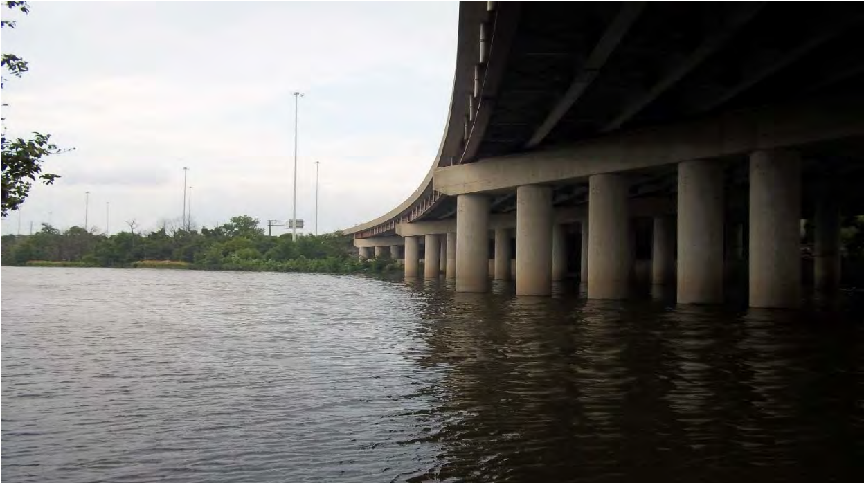
US-0. Looking East at upstream face of I-55 from Northwest bank
