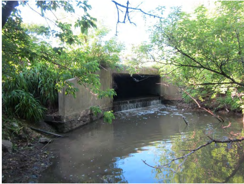
Figure 1. South elevation of I-55 and frontage roads over a stream.
