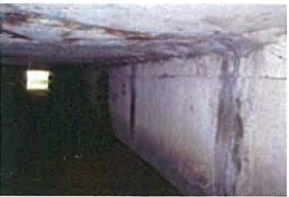
0015_Culvert-General View Lc
