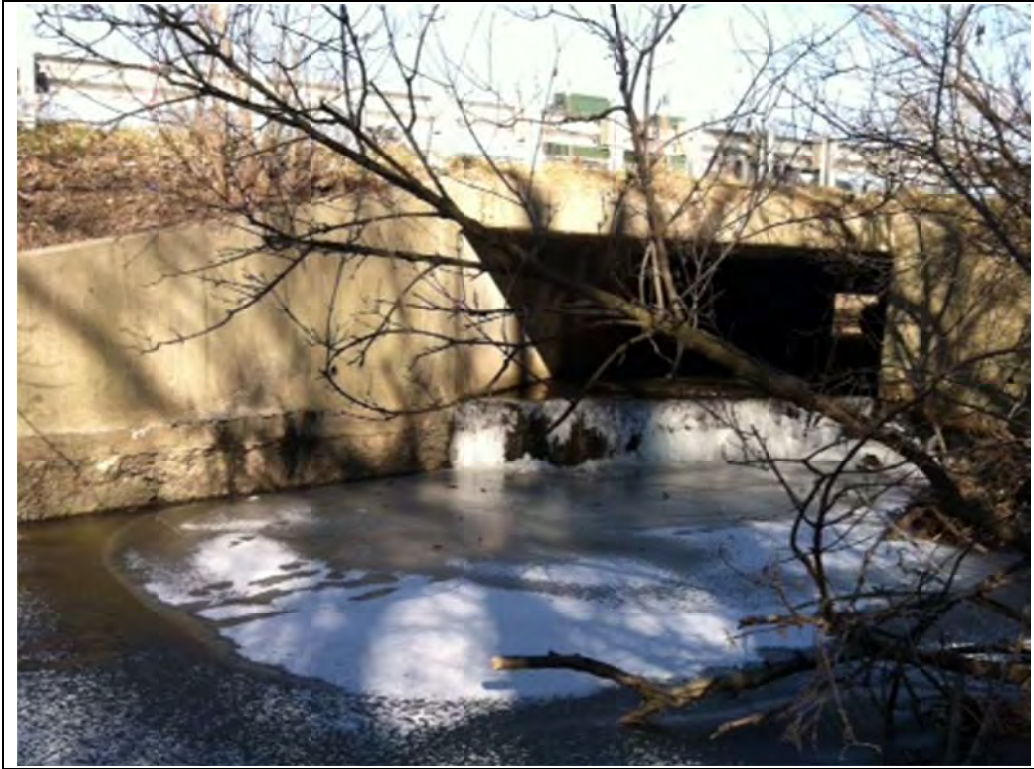
Photo #3 – Downstream Face of East Branch Sawmill Creek (Looking Northeast)
