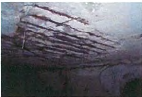
Culvert-Central Section Major Sp
