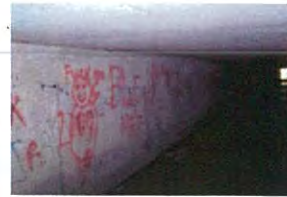
108_0008_Culvert-W Wall Loc
