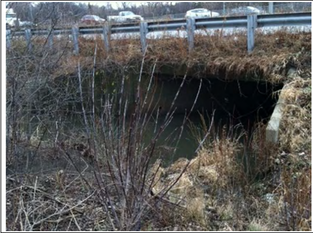
Photo #1 – Upstream Face of East Branch Sawmill Creek (Looking Southeast)
