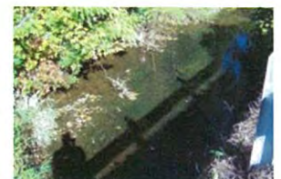
0019_Channel-General View of C
