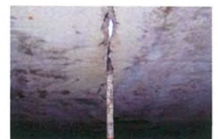
Culvert-Full Depth Xverse Crk T
