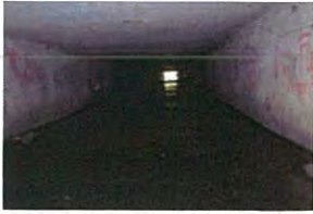
_0006_Culvert-General View I
