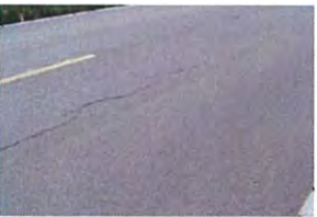
Surface-Roadway Over Culve
