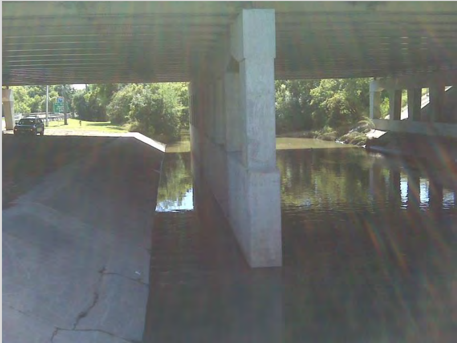
18. Looking South downstream at concrete slopewall under I-55 Bridge
