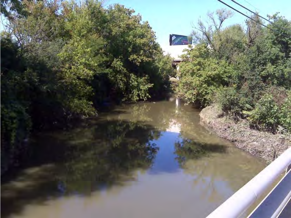
13. Flag Creek looking upstream, northwest from Wolf Road Bridge
