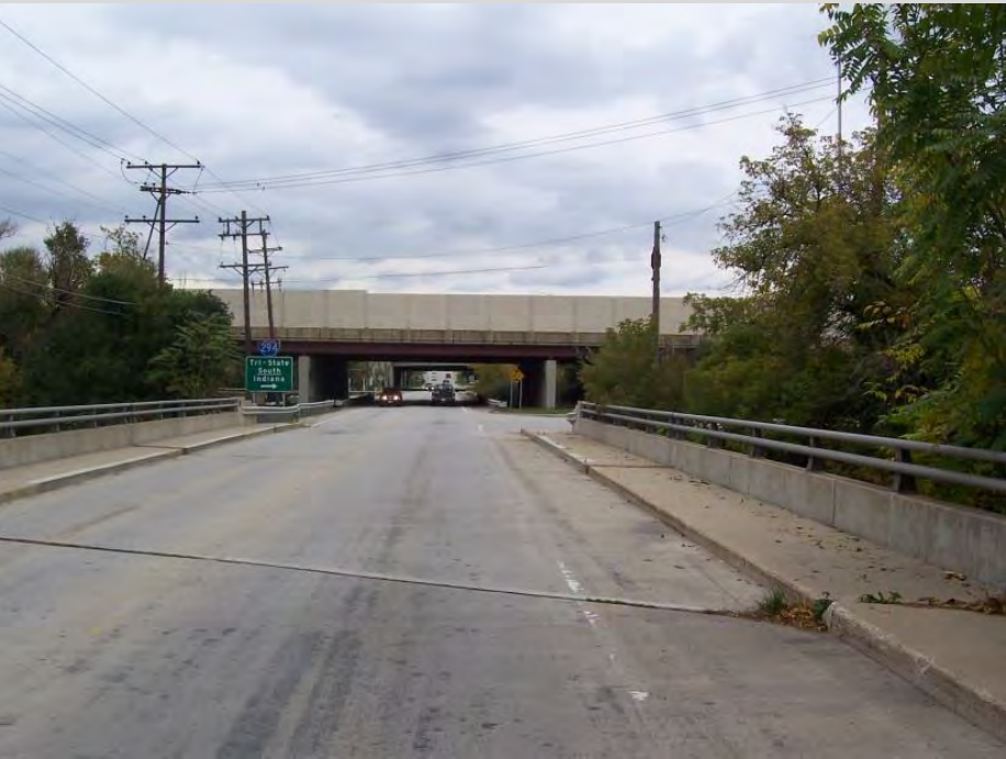
9. Wolf Road Bridge over Flag Creek, looking North
