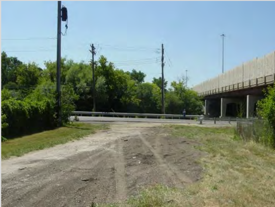
7. Access road looking West at Wolf Road and I-55 Bridge
