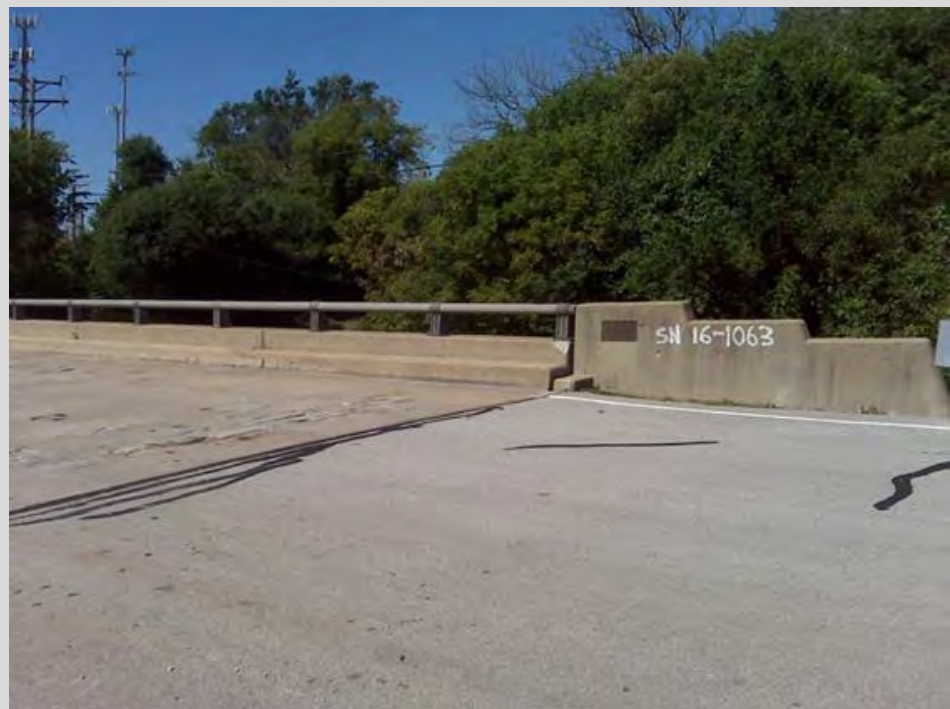
16. Wolf Road Bridge over Flag Creek
