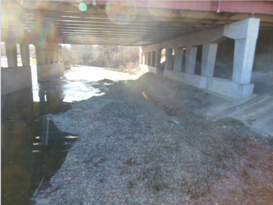
21. Flag Creek looking South downstream under I-55 Bridge in low-flow condition
