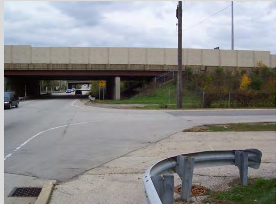
8. Intersection of Wolf Road and 71 st Street, looking North at I-55 Bridge
