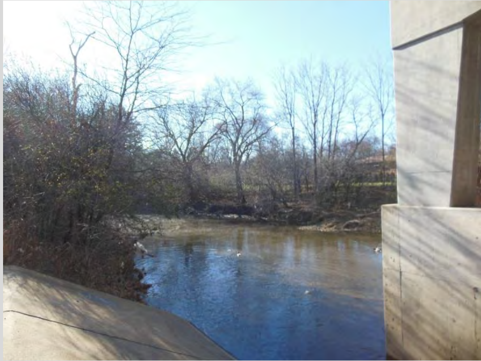
26. Flag Creek looking downstream, southeast, from under I-55 Bridge.
