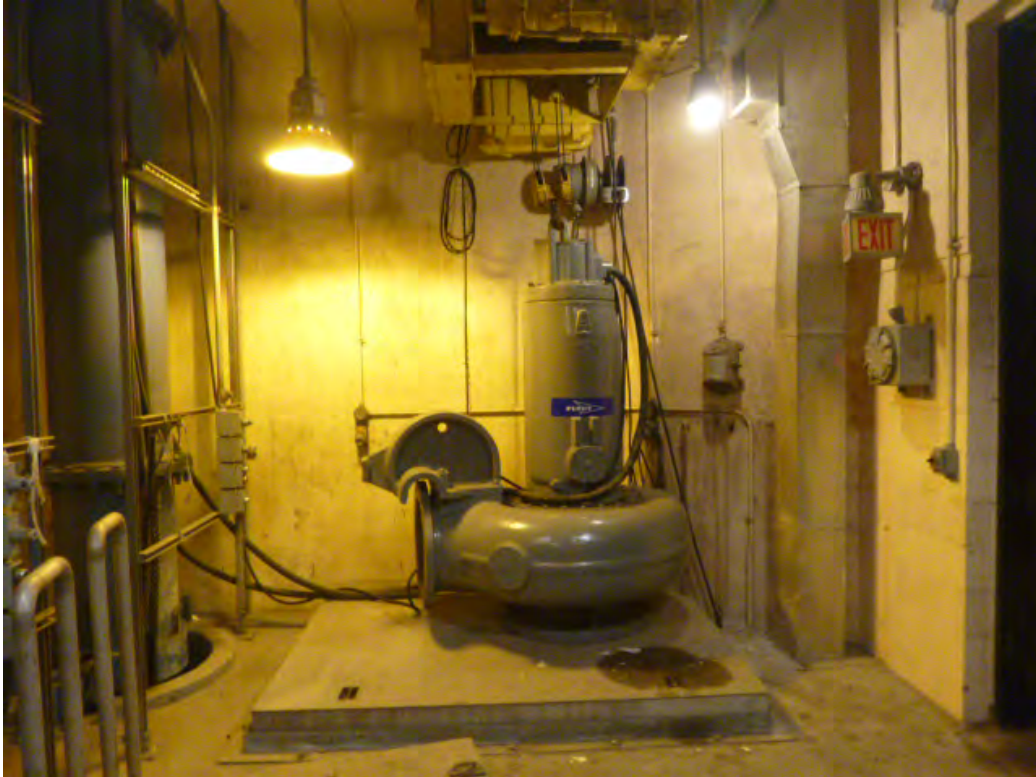
8. PS 30, pump room, intermediate floor, looking south
