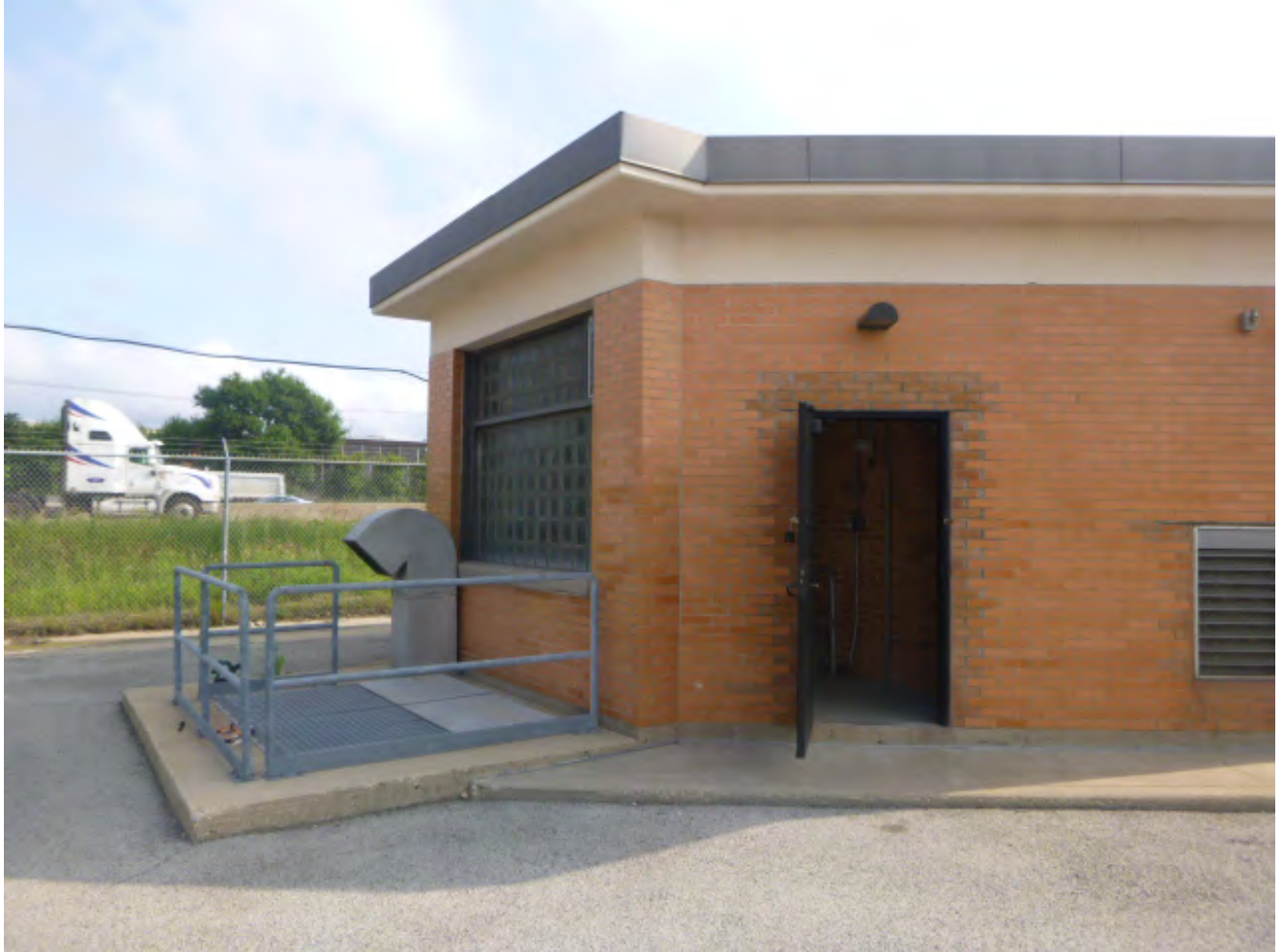
1. PS 30 Building, view from the southwest
