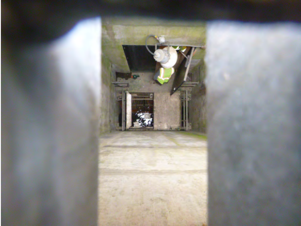
2. PS 30, looking down air shaft at trash rack
