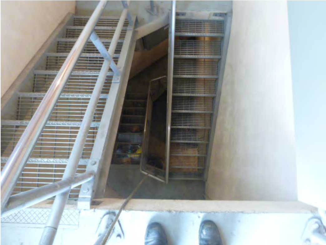
3. PS 30 looking down toward wet well
