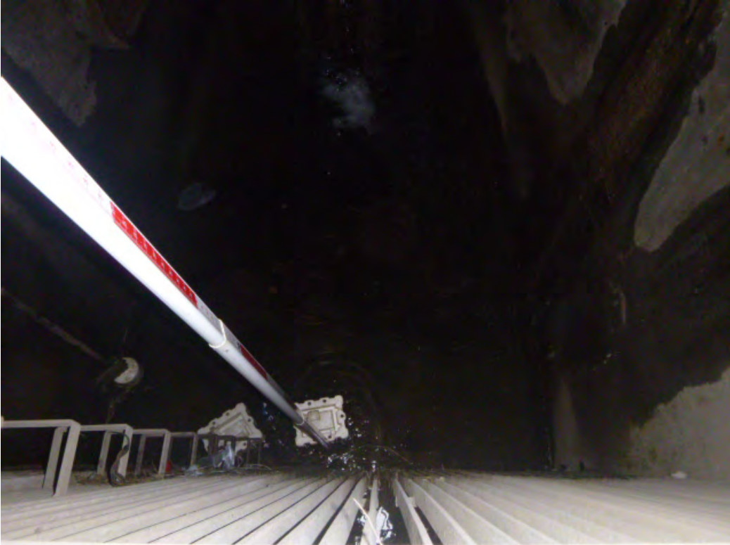
5. PS 30, looking down toward wet well
