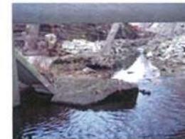
0220207-20111220-0022- Channel~Channel at end o...
