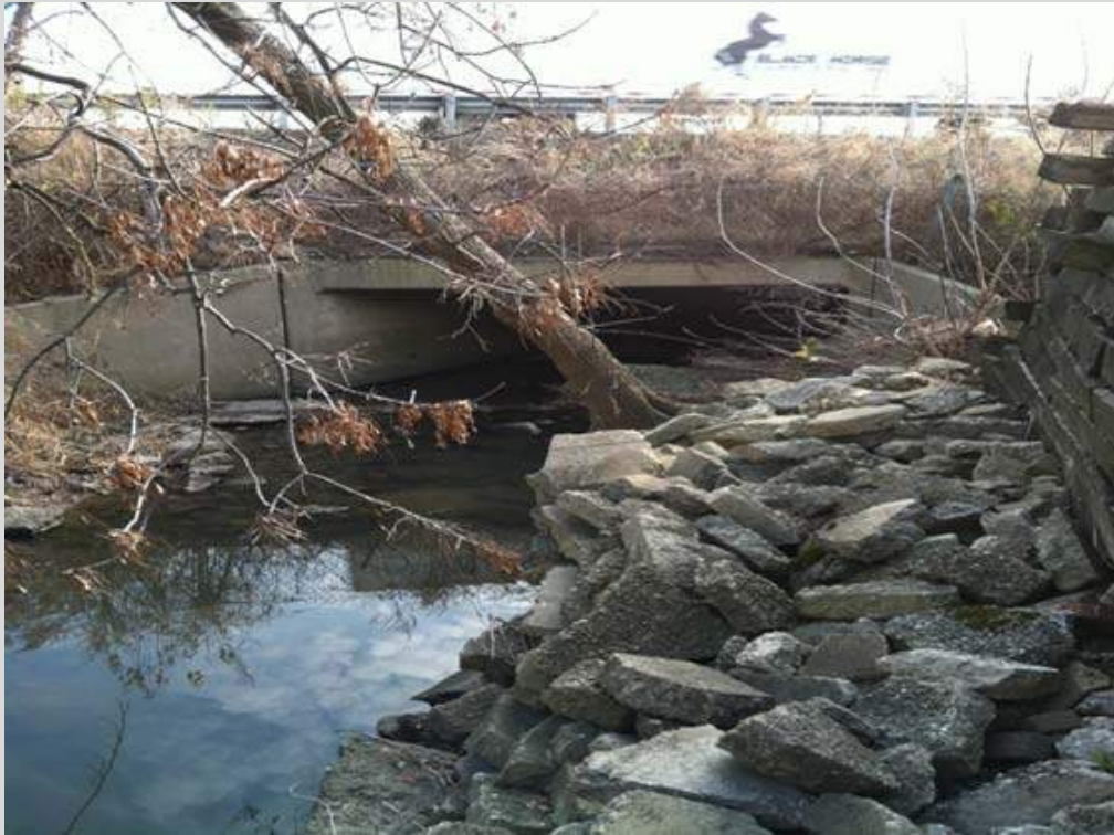
7. Looking Downstream I-55 Culvert at U/S Face.
