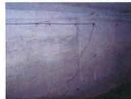
0220207-20111220-0021- Culvert~End of cable Esti...
