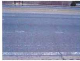
0220207-20111220-0001- Deck Surface~Typ surface...
