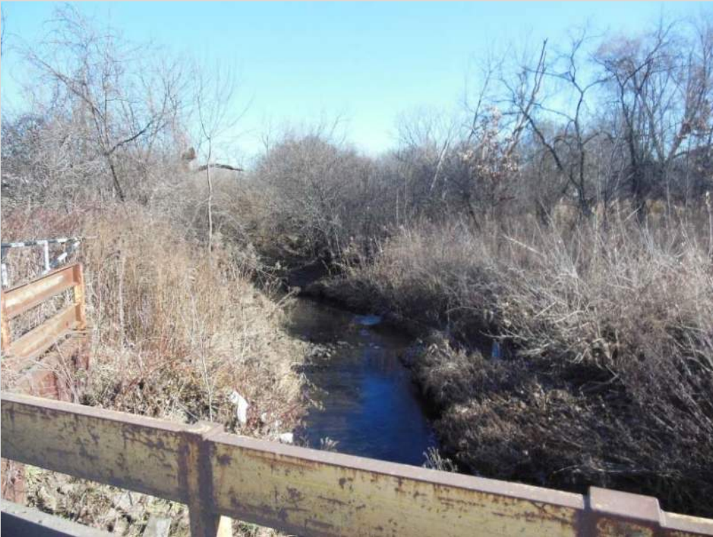
3. Looking at Downstream Floodplain at Private Bridge.
