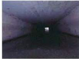
0220207-20111220-0010- Culvert~General culvert co...
