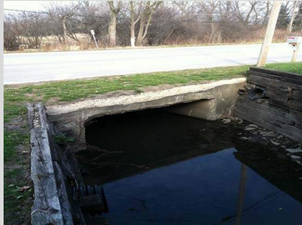
8. Looking Upstream North Frontage Road Culvert at D/S Face.
