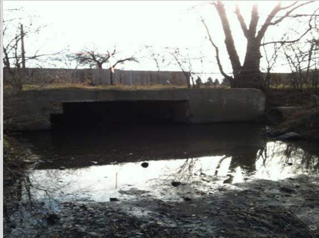
12. Upstream face of North Frontage Road Culvert.
