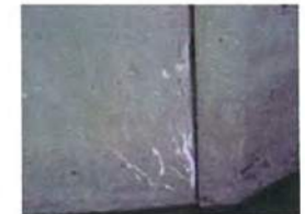
0220207-20111220-0023- Wingwalls~Efflorescence...
