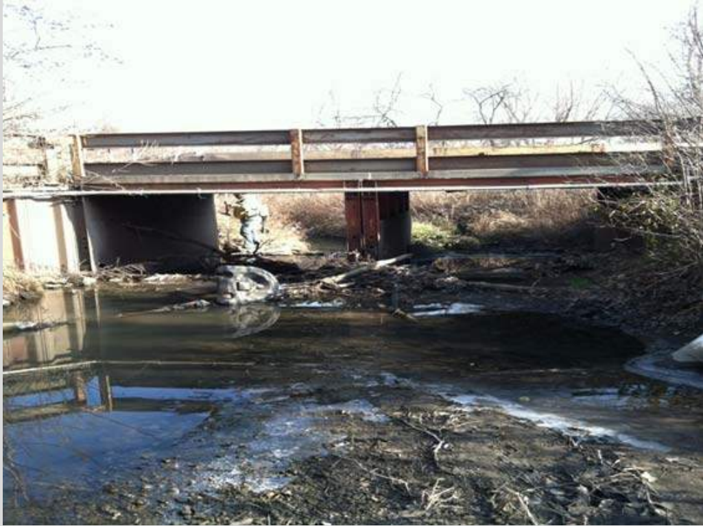
1. Looking Upstream at Private Bridge.
