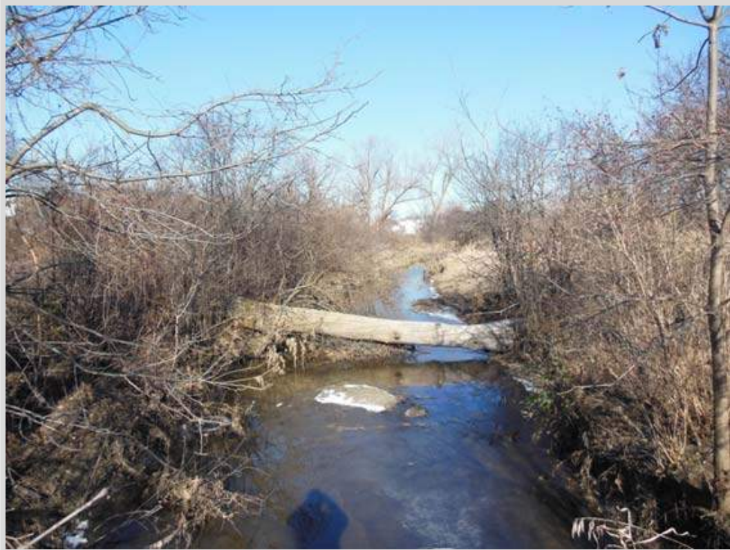
11. Floodplain Upstream of North Frontage Road Culvert.
