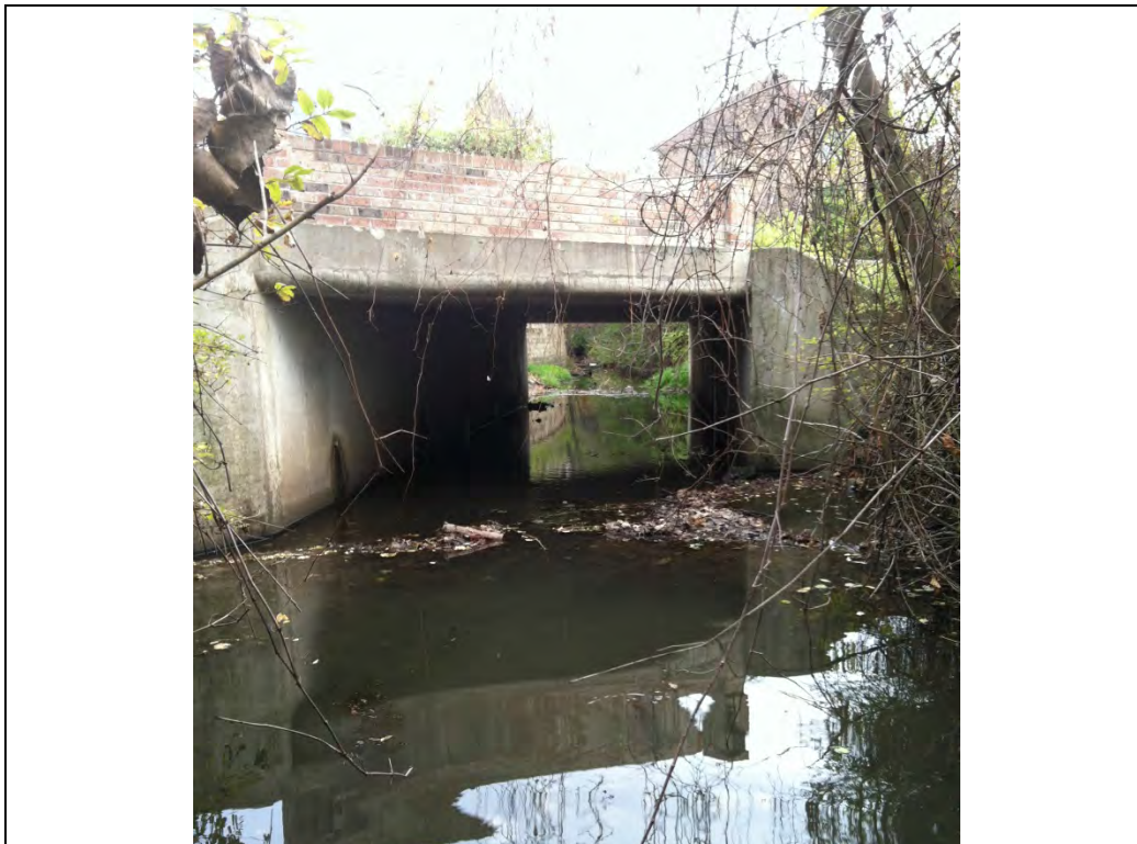
Photo #25 – Upstream Face of Kimberly Court Culvert (Looking East)
