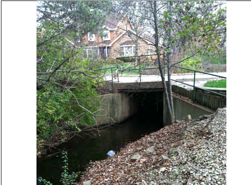
Photo #15 – Upstream Face of Carlisle Court Culvert (Looking East)
