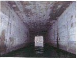
46 - General condition S section
