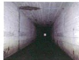
39 - General condition N section
