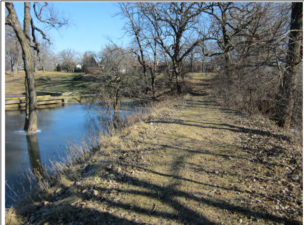
Photo #8 –Golf Course Berm (Looking East)
