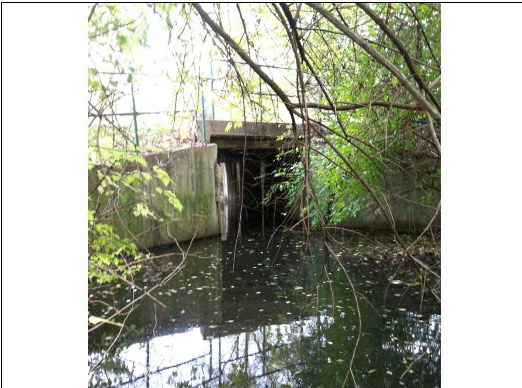
Photo #21 – Upstream Face of Kentwood Court Culvert (Looking East)
