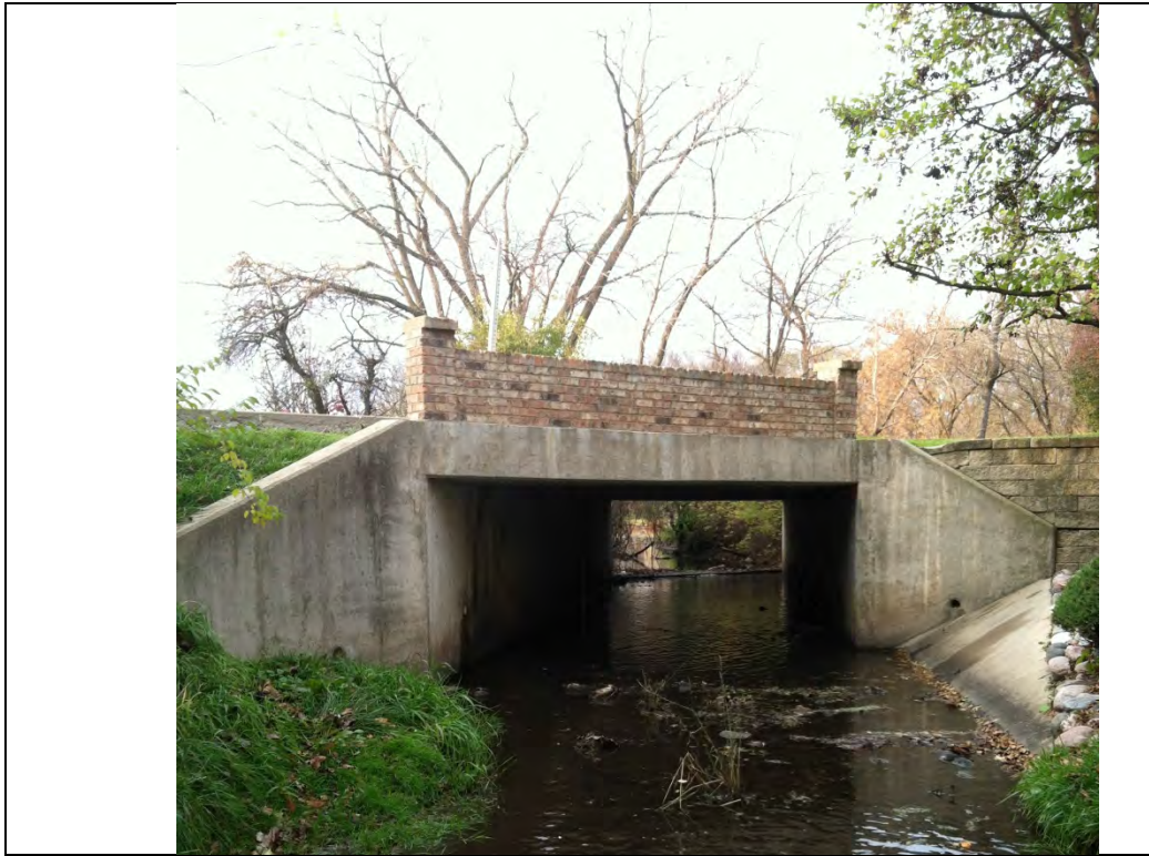
Photo #24 – Downstream Face of Kimberly Court Culvert (Looking West)
