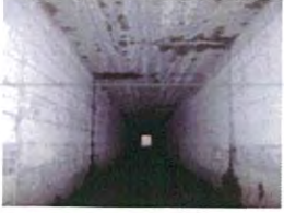
41 - General condition N section
