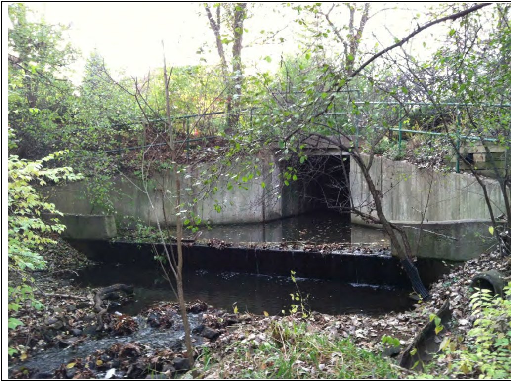
Photo #20 – Downstream Face of Kentwood Court Culvert (Looking West)
