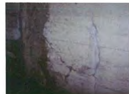
25 - Random cracking
