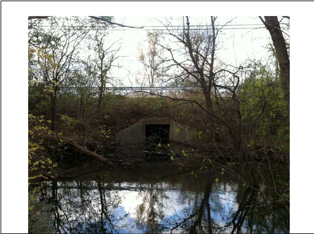
Photo #1 – Downstream Face of Wards Creek Culvert (Looking North)
