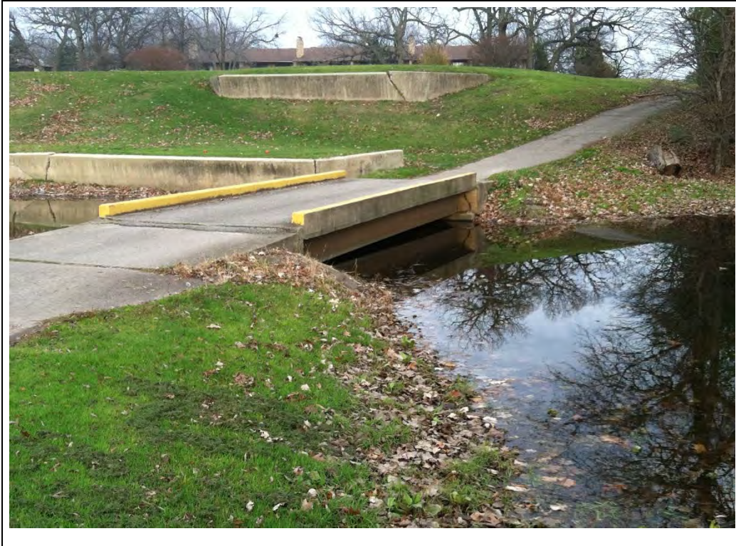
Photo #10 – Golf Course Bridge #1 (Looking Northeast)
