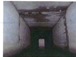
44 - General condition mid to S section lkg S
