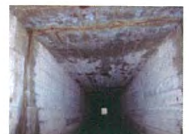
40 - General condition N section
