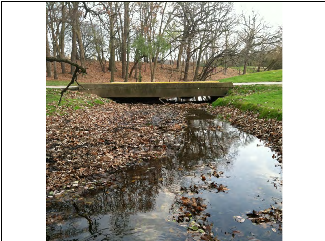
Photo #13 – Golf Course Bridge #2 (Looking South)
