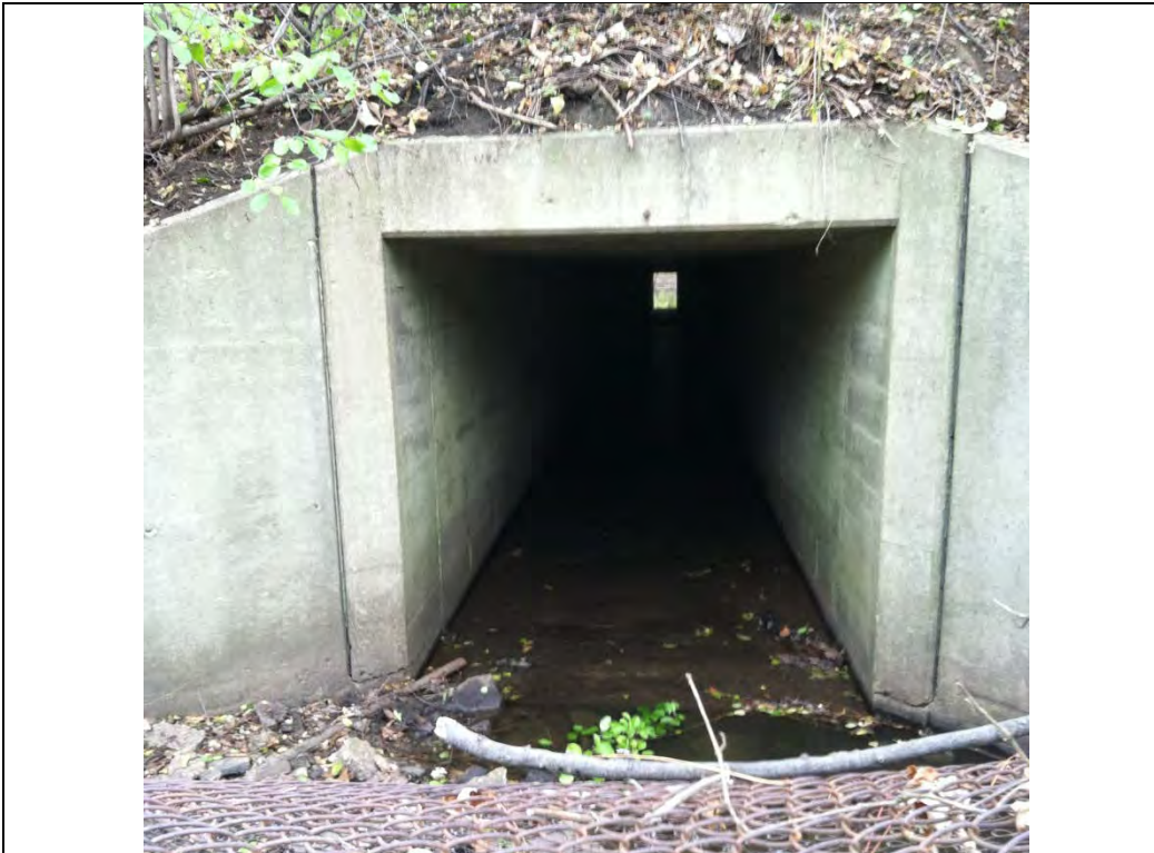
Photo #2 – Upstream Face of Wards Creek Culvert (Looking South)
