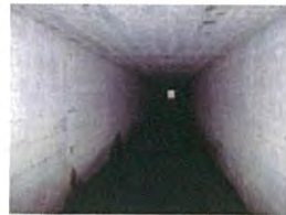
38 - General condition N end
