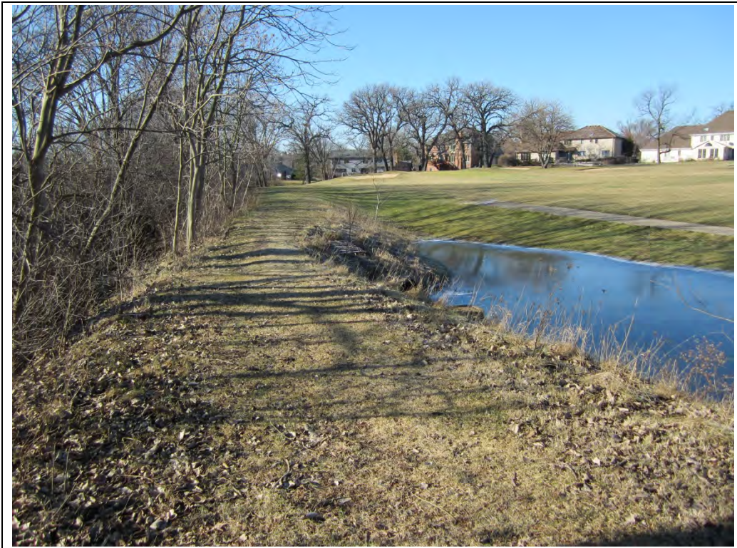
Photo #7 –Golf Course Berm (Looking West)
