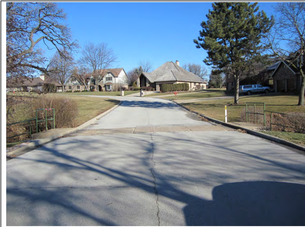
Photo #18 – Carlisle Court (Looking North)
