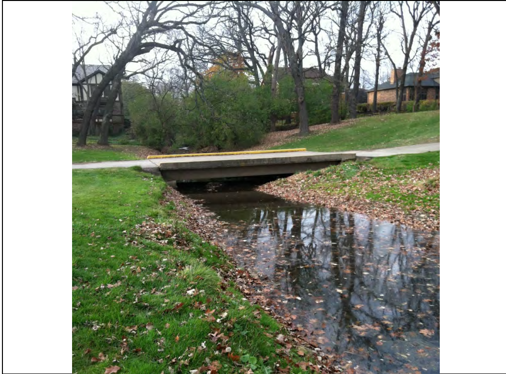
Photo #12 – Golf Course Bridge #2 (Looking North)
