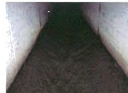
28 - flow break possible minor settlement or chang...
