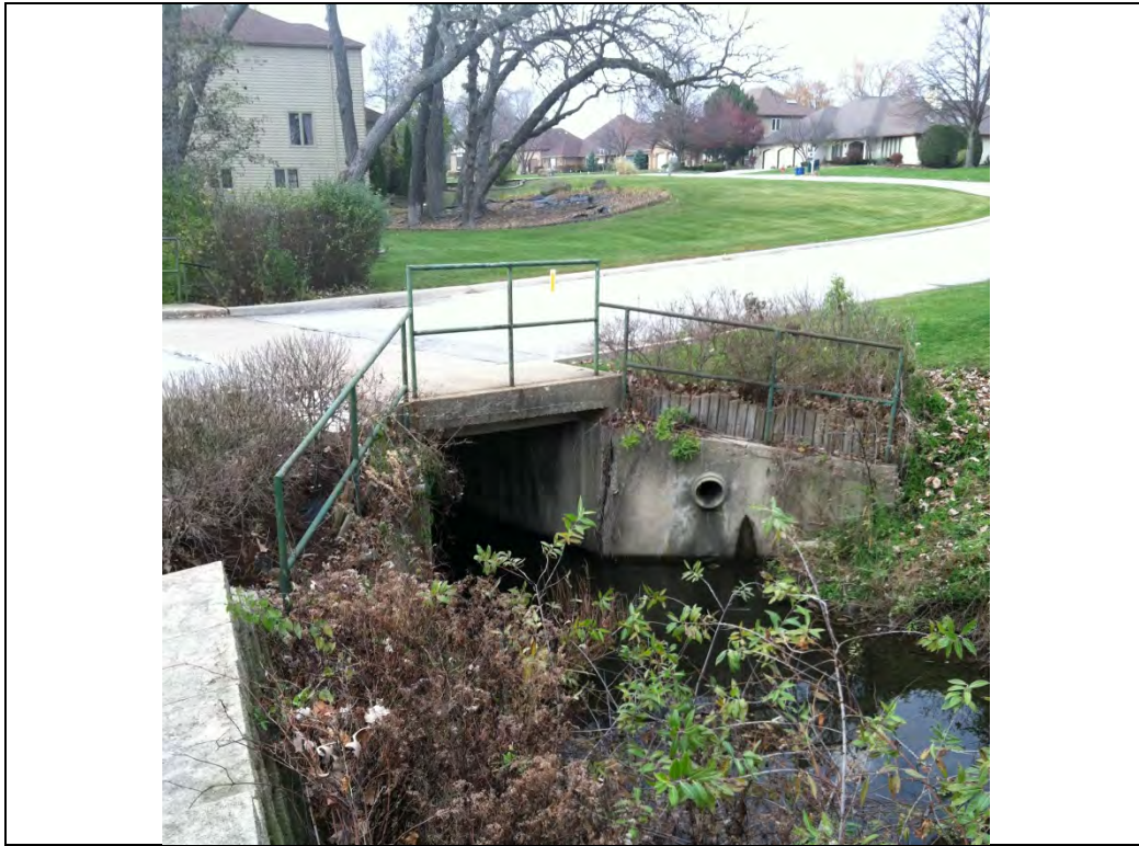
Photo #14 – Downstream Face of Carlisle Court Culvert (Looking West)
