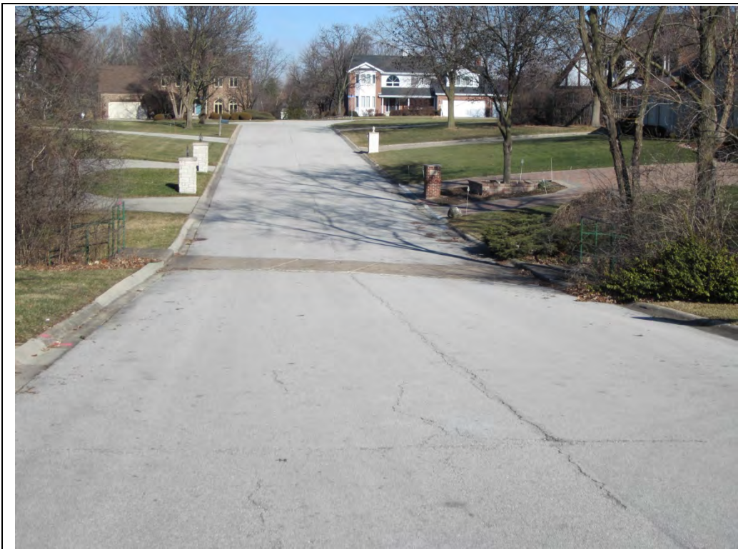
Photo #19 – Kentwood Court (Looking Northwest)
