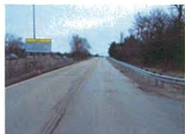
02 - S Frontage Rd approach lkg E
