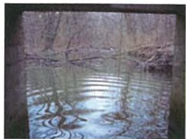
47 - S end and channel Note electric cable
