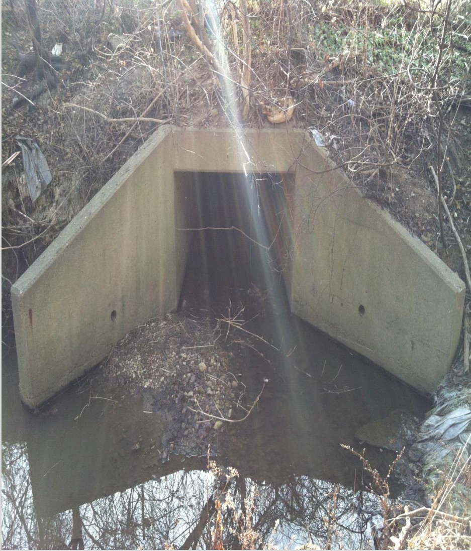
29. Upstream Face of I-55 Structure Culvert
