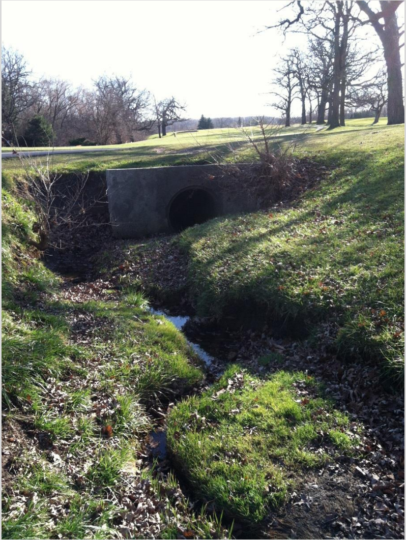
38. Upstream face of Golf Cart Culvert
