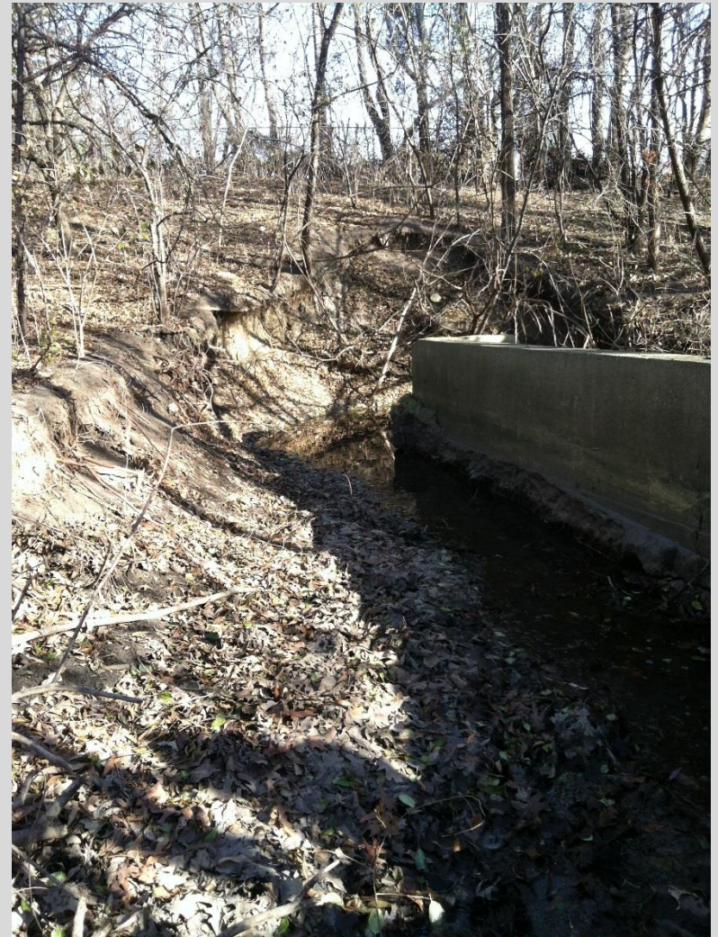
36. Upstream face of Weir showing creek bypass
