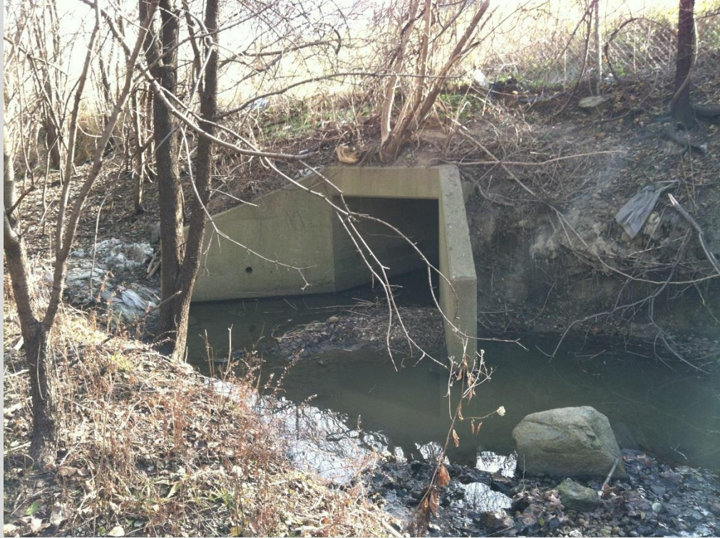
30. Upstream Face of I-55 Culvert
