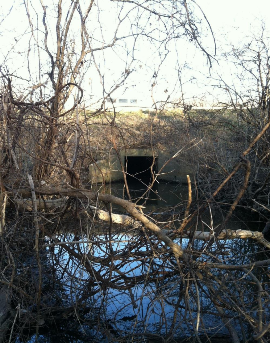
28. Downstream Face of I-55 Structure Culvert
