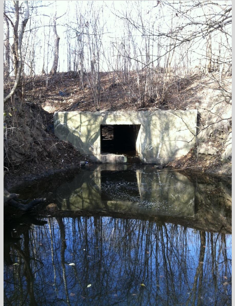
31. Downstream Face of North Frontage Road Culvert
