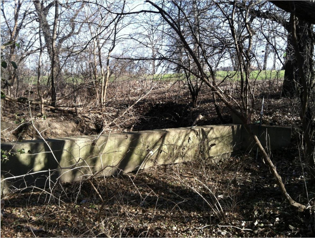
35. Photo along Face of Weir
