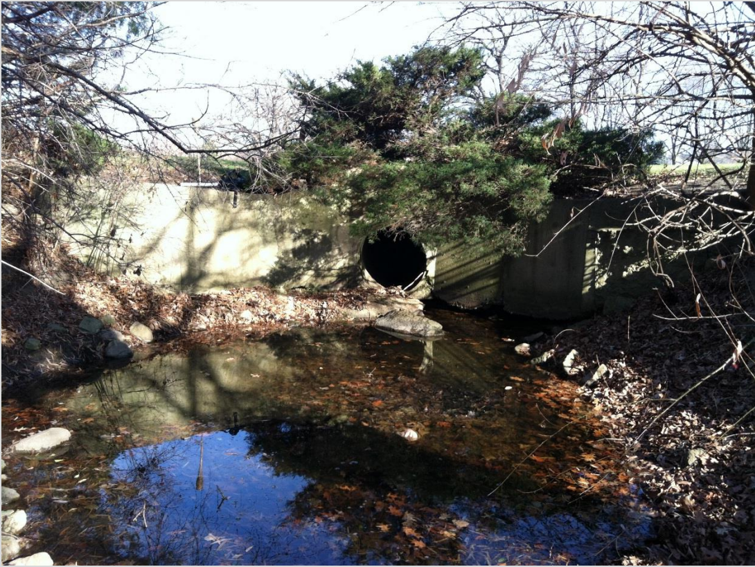
37. Downstream face of Golf Cart Culvert
