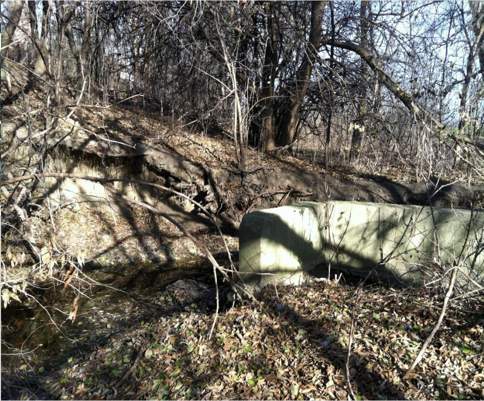
34. Downstream Face of Weir showing creek bypass
