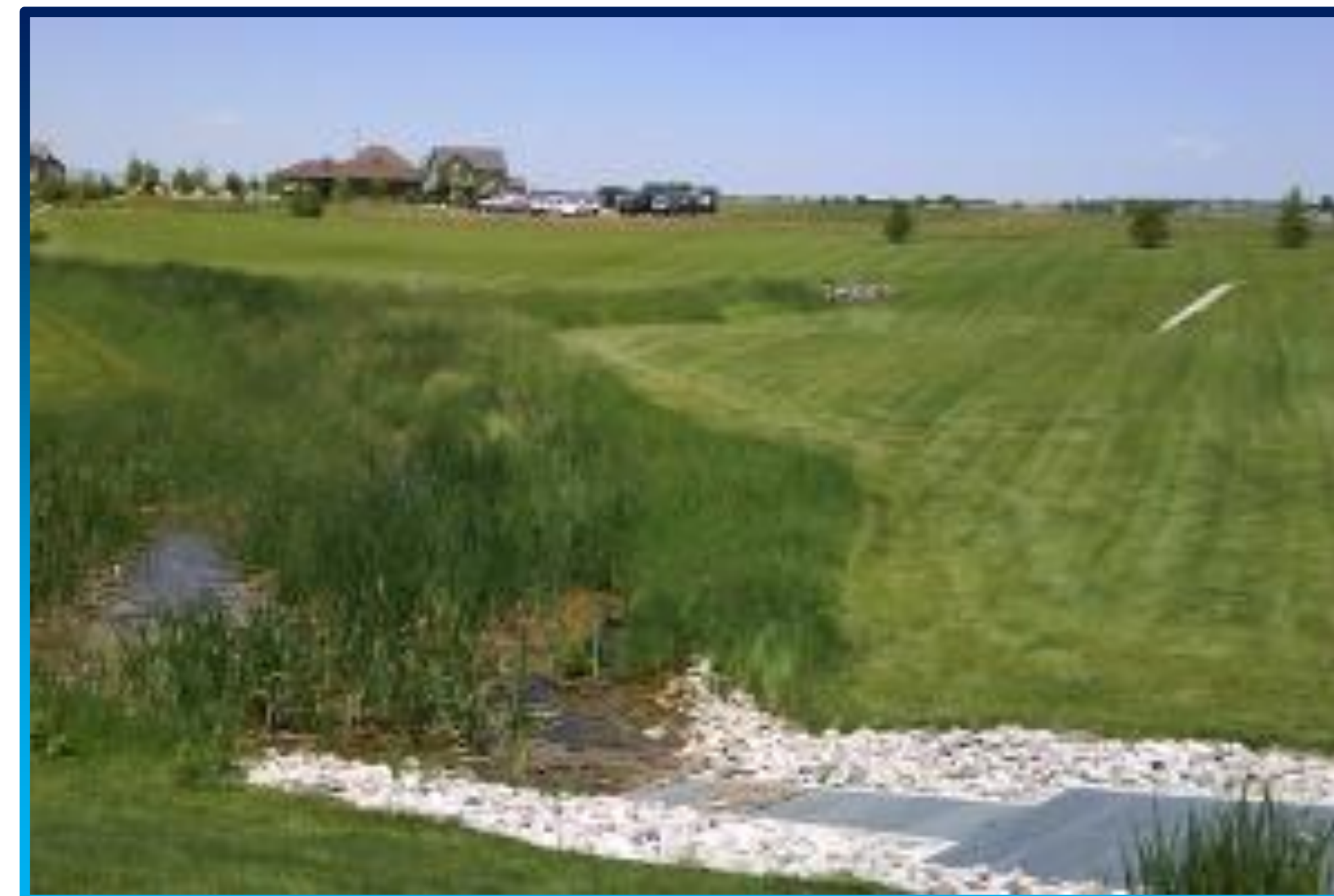
PIPE INLET PROTECTION
