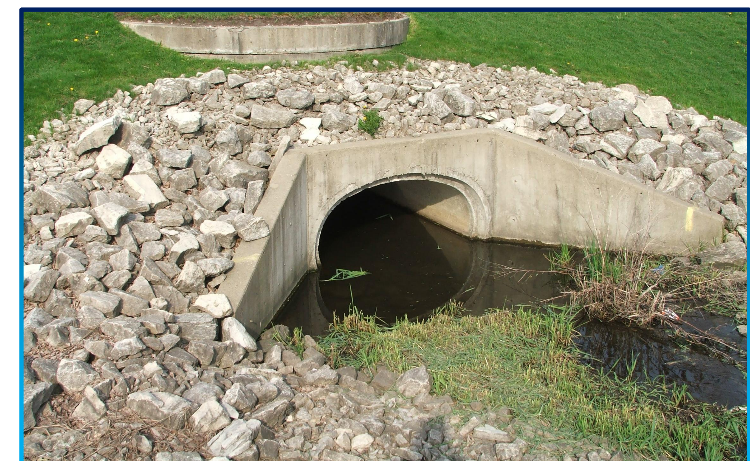
PIPE OUTLET PROTECTION
