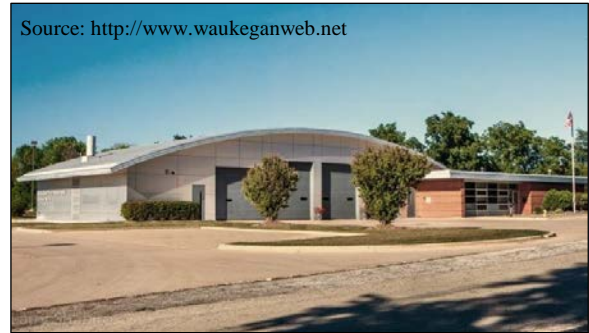
▲ A mountable median at Yorkhouse Road will provide a clear path for fire trucks turning to and from the Waukegan Fire Department Station #5.
