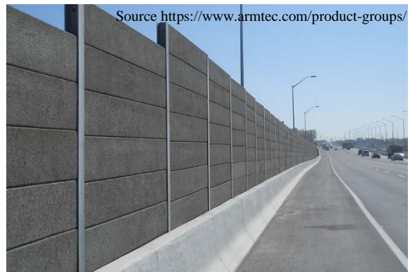
▲ Noise walls, such as the one shown above, reduce overall noise levels. IDOT will decide whether to build walls based on the desires of the property owners and residents who will benefit from them.
