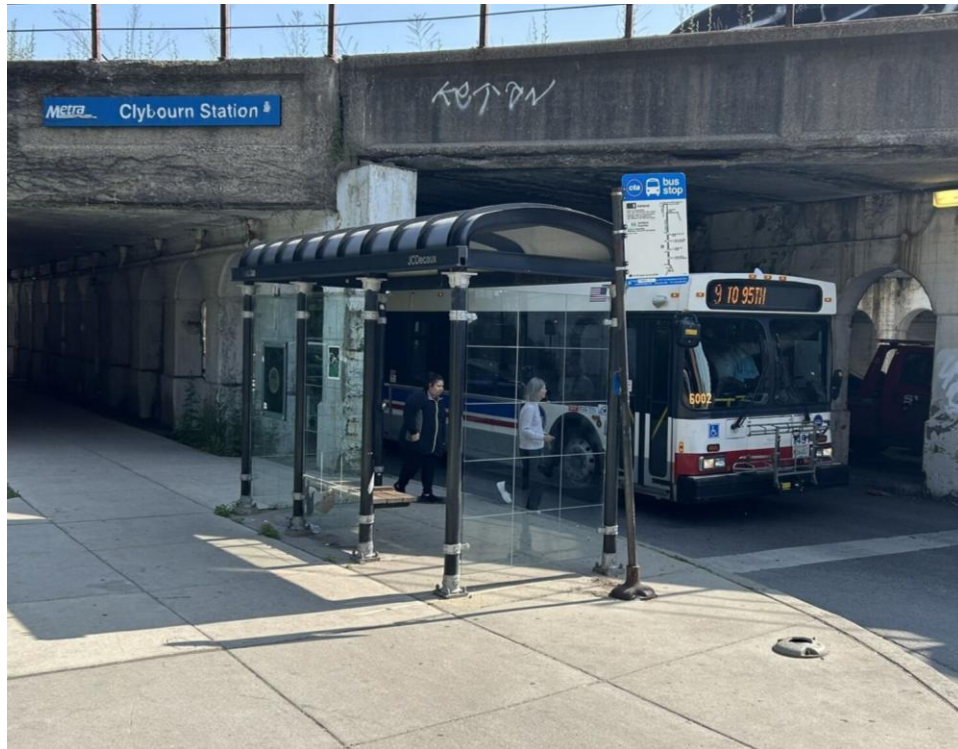
Transit Service – CTA Route 9 Southbound Stop W. Cortland, Looking North
