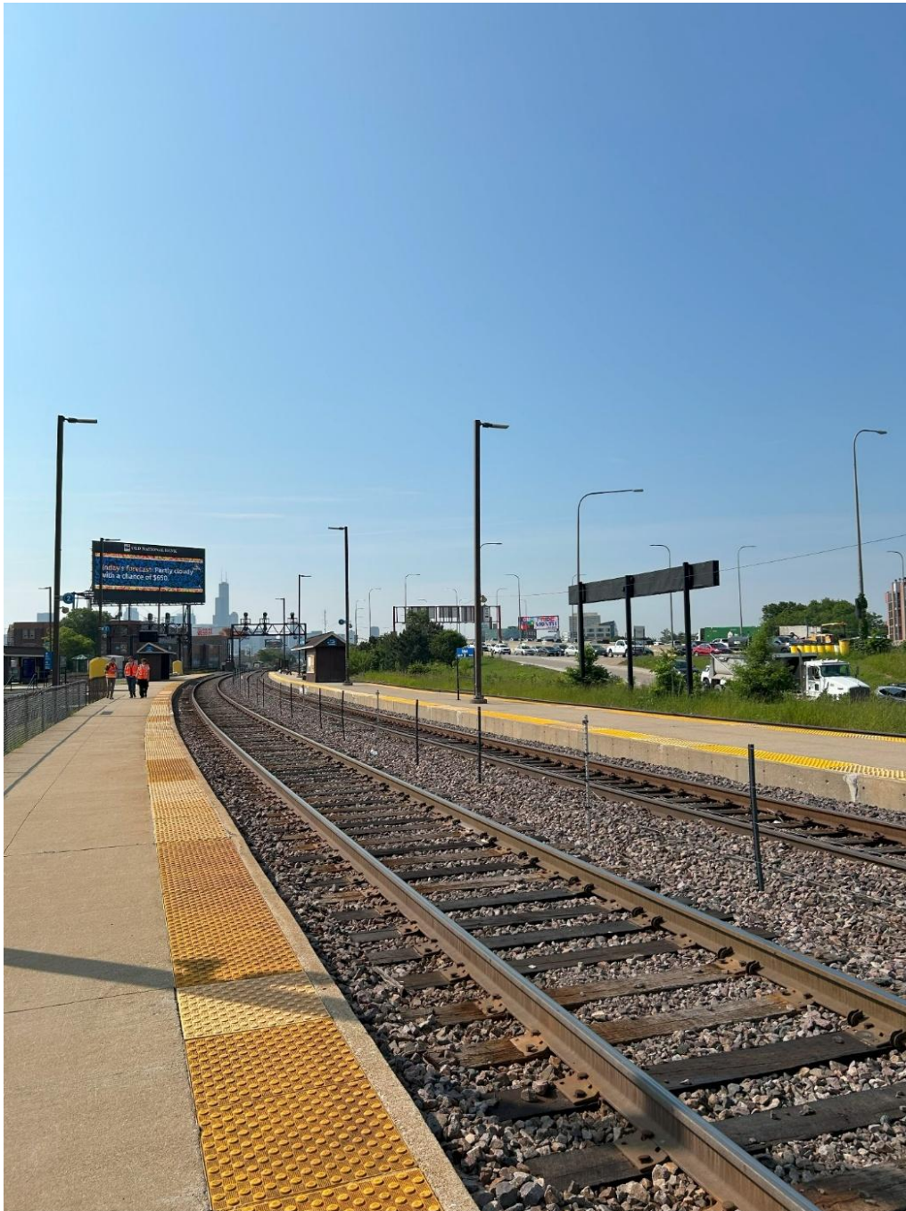
Metra Clybourn Station – Center and West Platform Looking South
