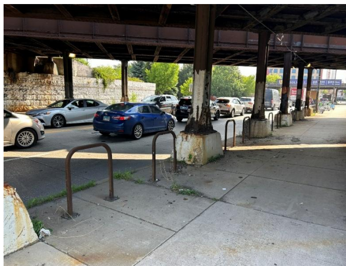
Figure 15-Road Congestion Metra Clybourn Station
