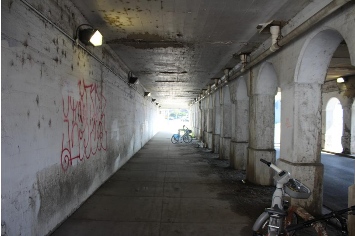
Pedestrian Corridor looking West along West Cortland Street
