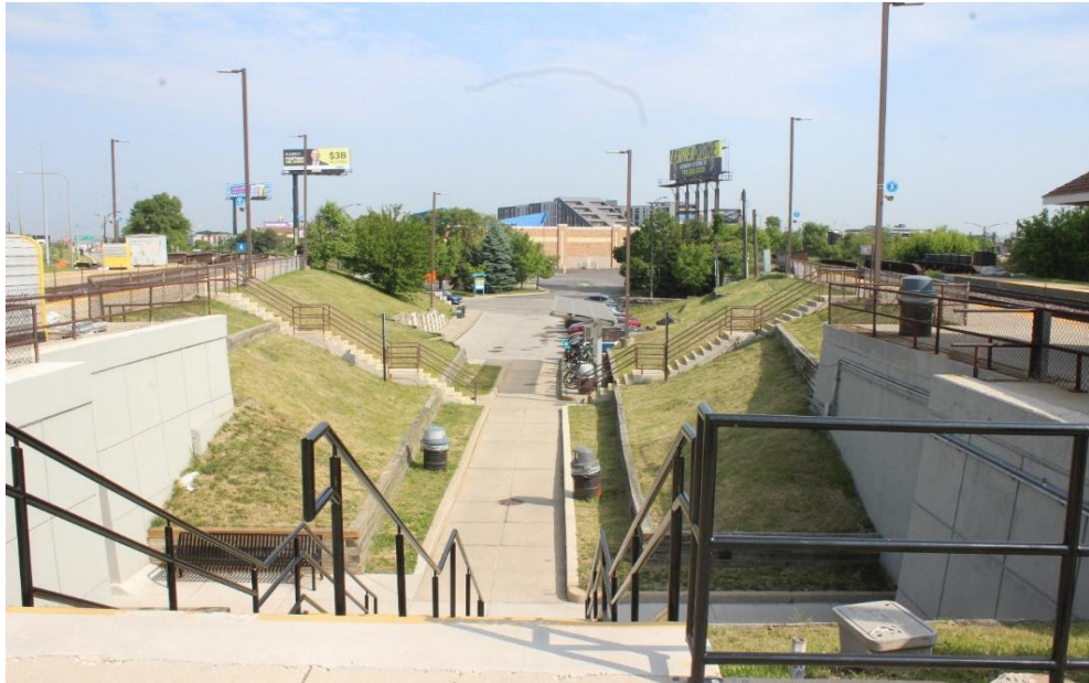
Metra Clybourn Station West Armitage Entrance, Auto and Bicycle parking areas. Looking North
