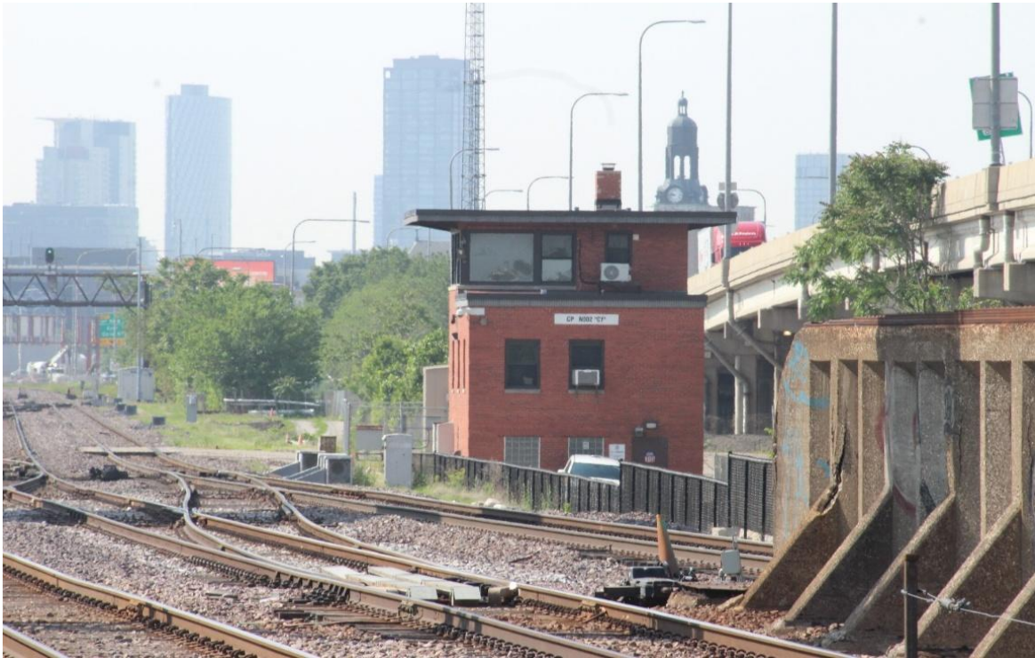
Historic Signal Tower – Approximate Crossing Area of 606 Trail. Looking South and West
