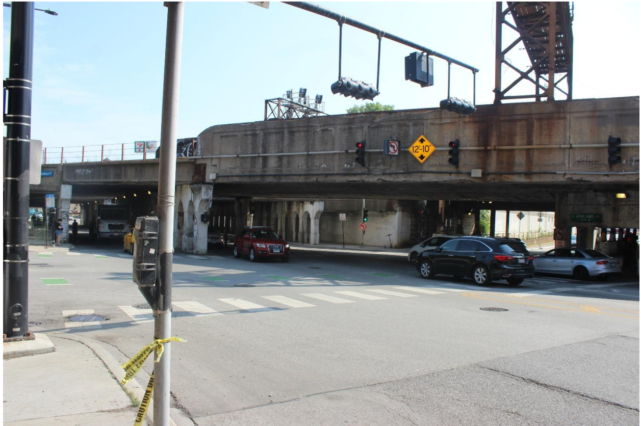
Looking Northeast at Intersection of Ashland Ave and W Cortland Street
