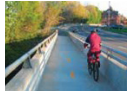
Sample separated shared-use path on bridge. Source: FHWA
