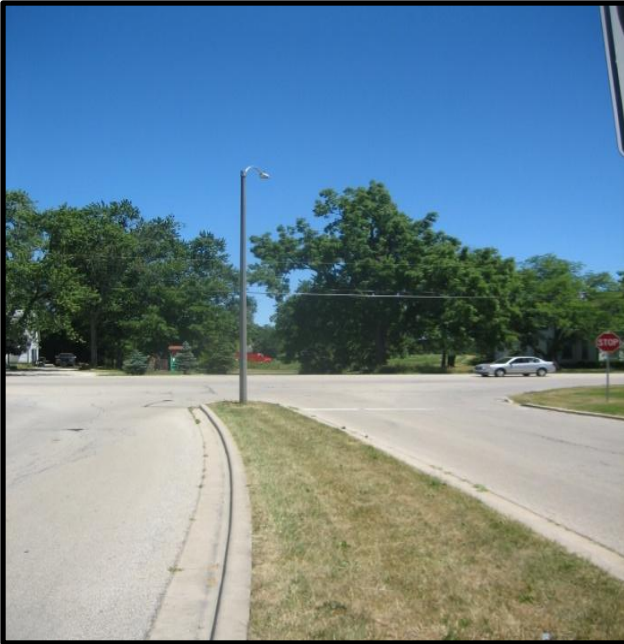
PICTURE 5 – Looking east on Independence Boulevard towards U.S. Route 45; Cobra-head on separate pole.
