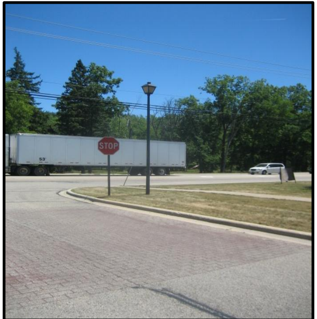
PICTURE 4 – Looking east on Country Place towards U.S. Route 45; Decorative lighting. 0
