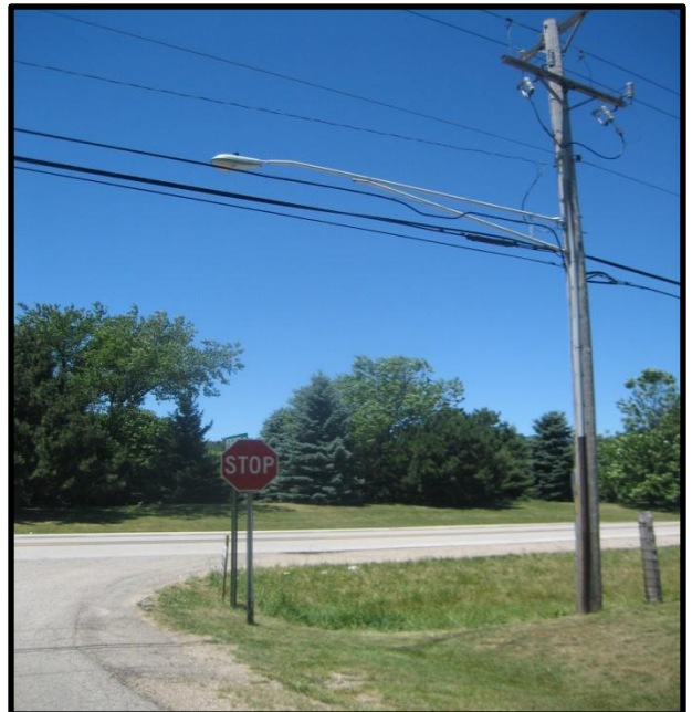
PICTURE 8 - Looking west on West Pedersen Drive towards U.S. Route 45; Cobra head on separate pole. (Typical for Burr hollow Drive)
