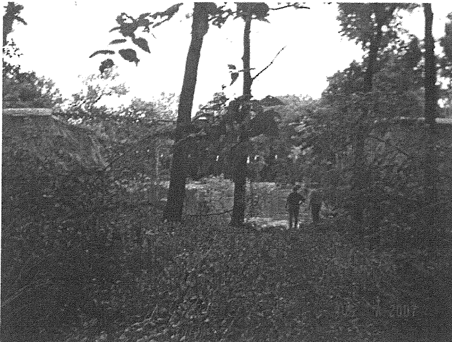
Chicago Northwestern Railroad Embankment Failure
