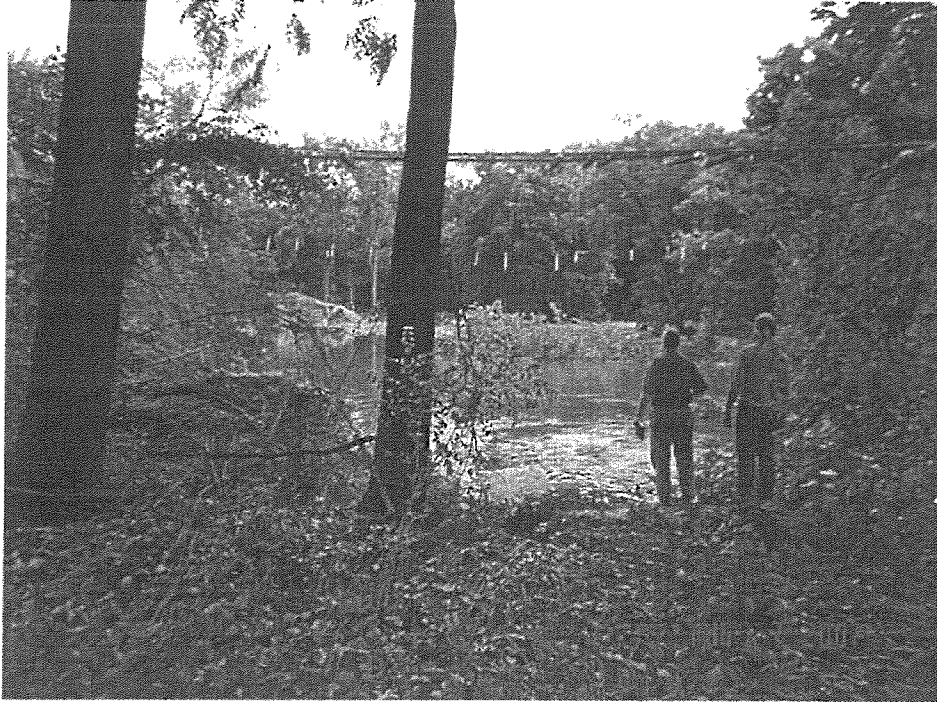
Chicago Northwestern Railroad Embankment Failure
