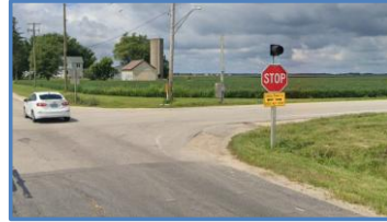
Flashing Beacons with Stop Sign at Intersection Crossing on Chicago Rd
