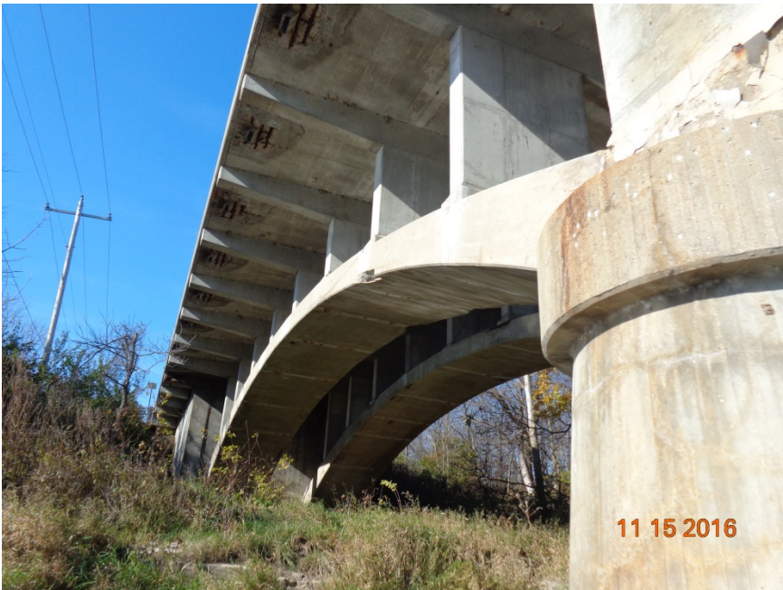
General Condition of Underside (Span 1)
