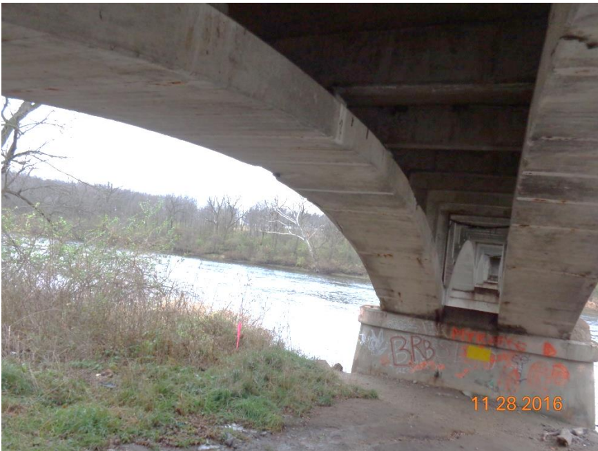
General Condition of Underside (Span 5)
