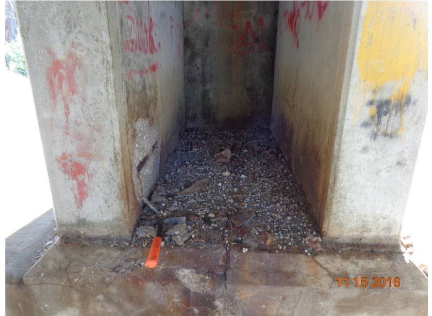
Pier and Columns under Joint
