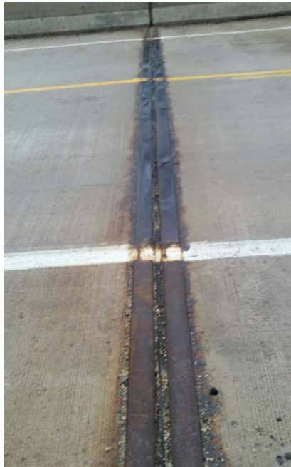
West Abutment Expansion Joint
