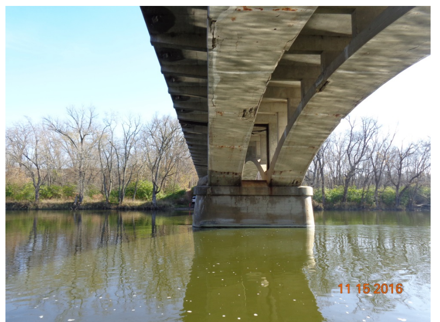
General Condition of Underside (Span 2)
