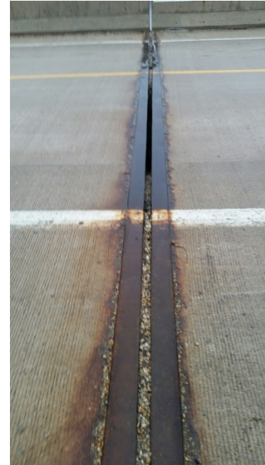
Pier 3 Expansion Joint
