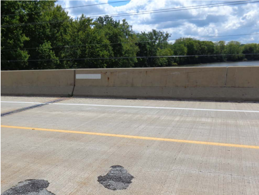
Typical Bridge Rail
