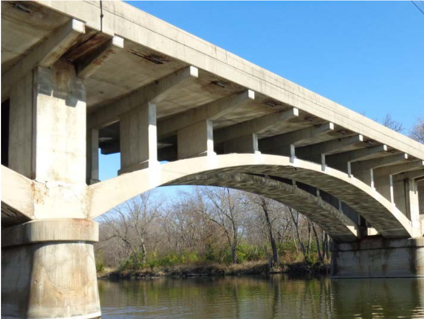
General Condition of Underside (Span 3)
