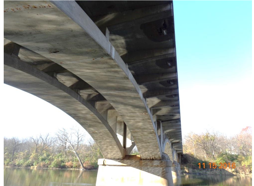
General Condition of Underside (Span 4)
