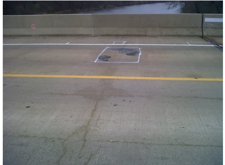
General Condition of Deck
