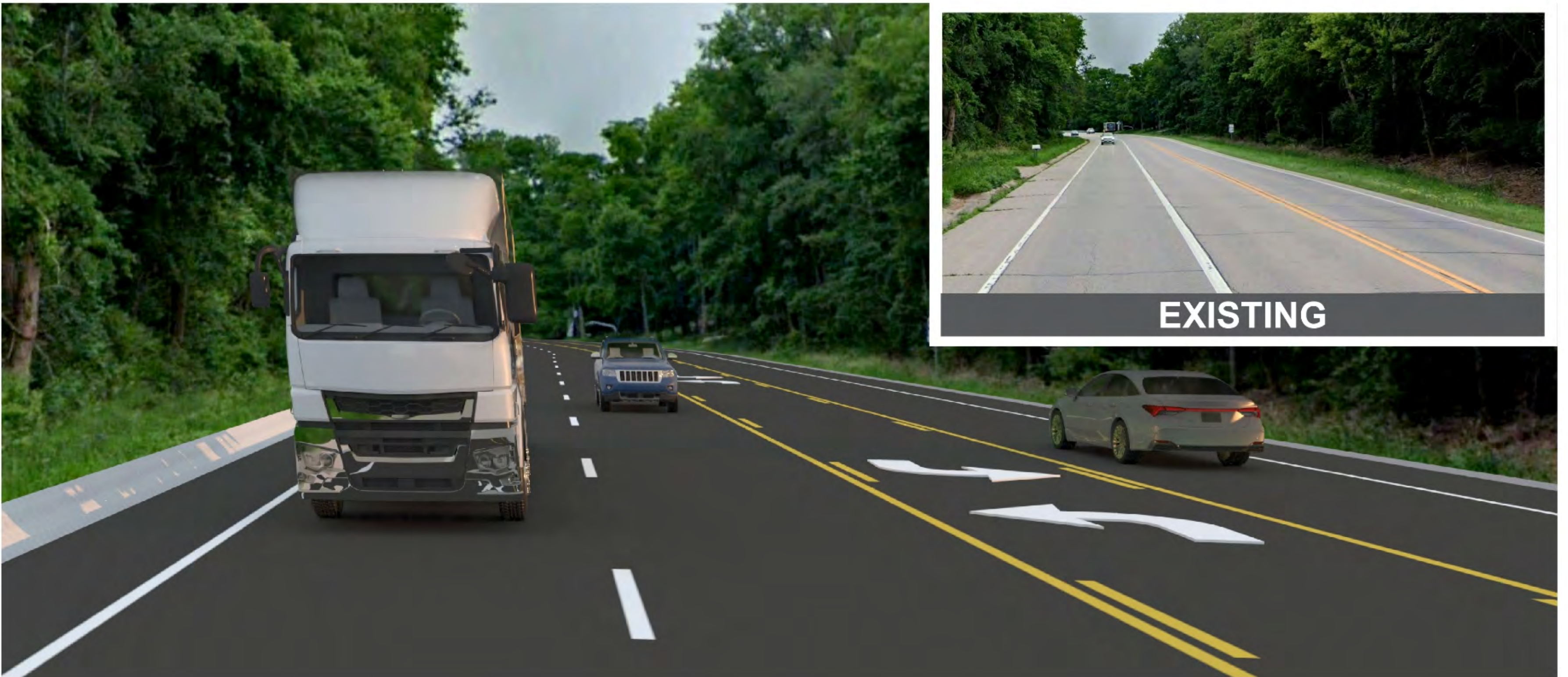
IL 9: 3-Lane Suburban Section with Truck Climbing Lane From beginning of project to Banner looking east
