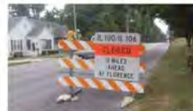
The Florence bridge closed to vehicle traffic on June 28 due to structural issues found during a routine inspection. (H-W Photo/Deborah Gertz Husar)
