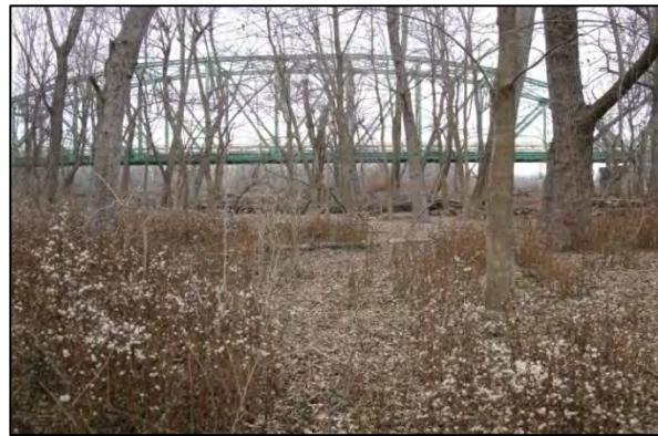
Photo D.6 - Forested Wetland Near Alternative 4 (Florence Bridge in background)
