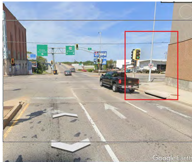
Figure 2-4. Intersection at North 3rd Street and Broadway Street (Red Box Indicates Building Potentially Causing Sight Issue)
