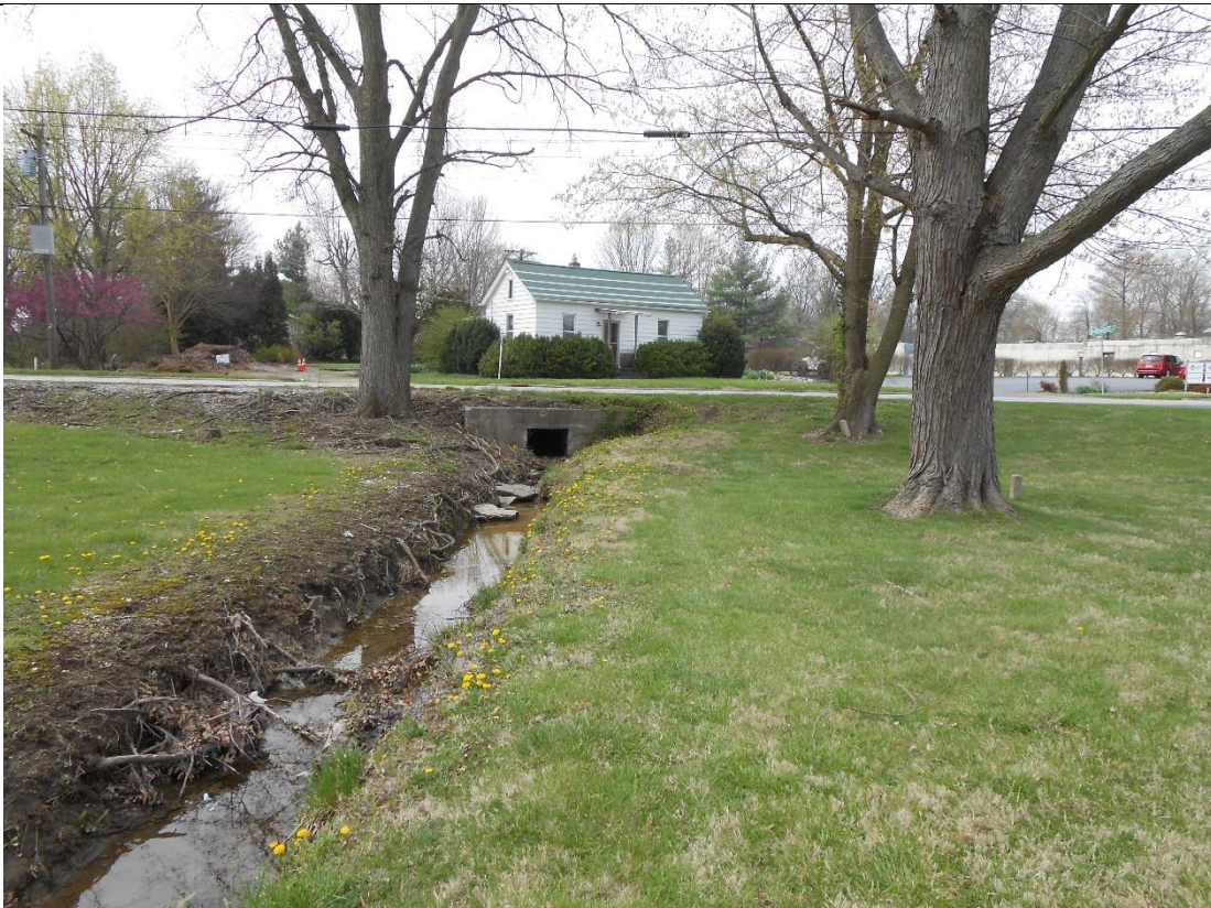
36" x 36" box culvert looking south at W. Delmar Ave.
