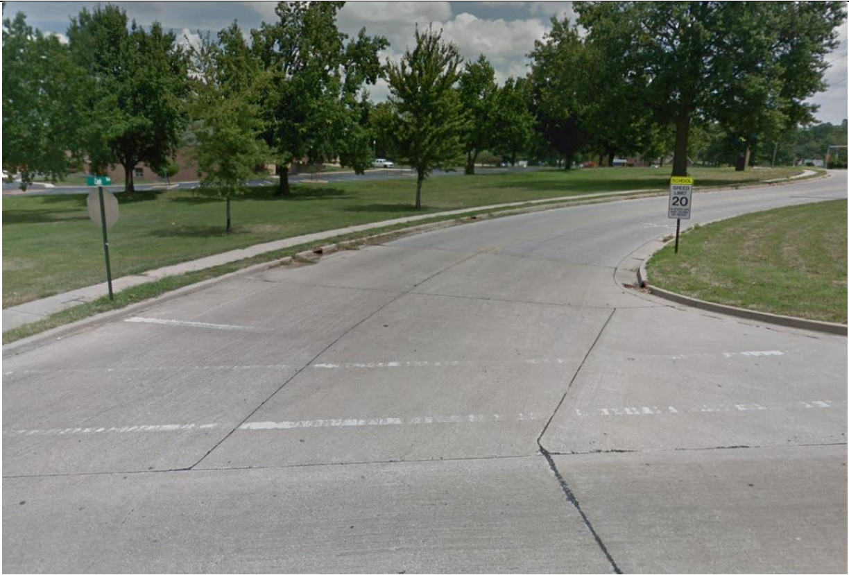
Looking east at Cook St. from Pierce Ln.
