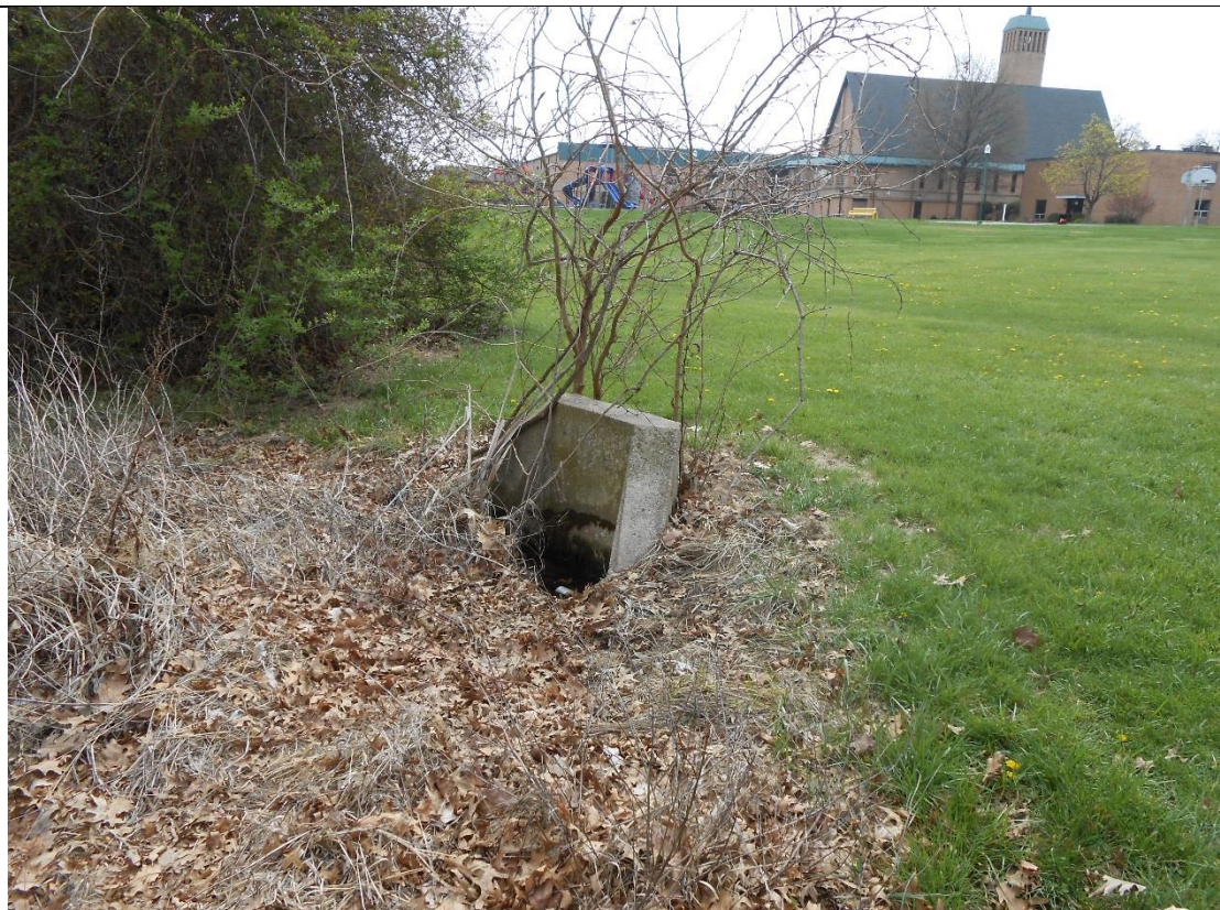
3 ft. x 3 ft. inlet at the north limit of the Evangelical United Church of Christ property
