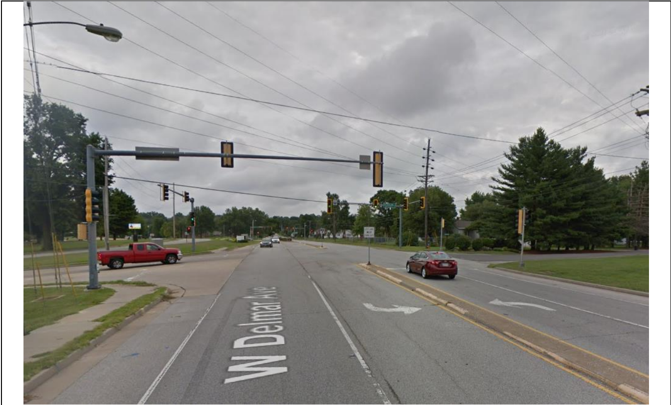
IL 3 looking east at the intersection with Pierce Ln.
