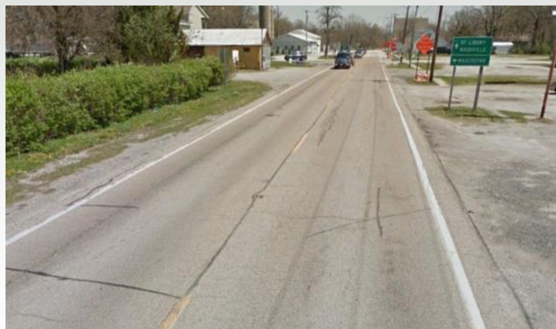
IL Route 4/15 east of 4 th St. looking east. The image shows the non-policy shoulder along this section
