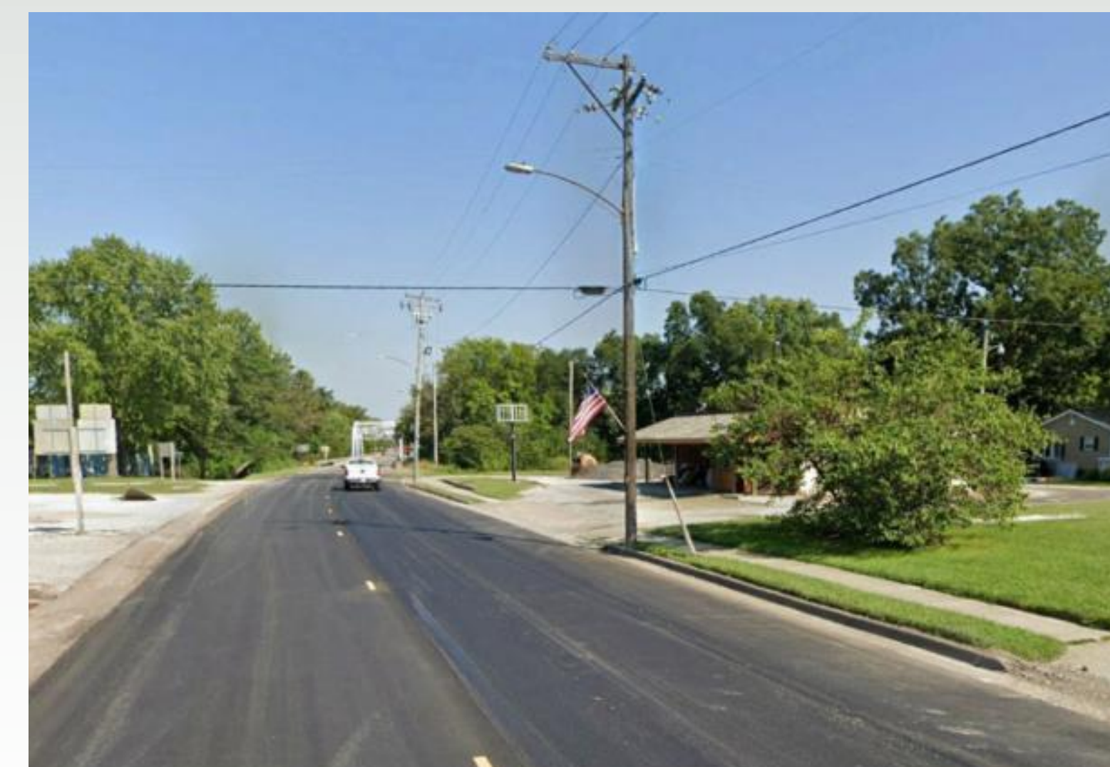
IL Route 4/15 just east of 2nd St. looking east. This image shows existing power poles within the clear zone.
