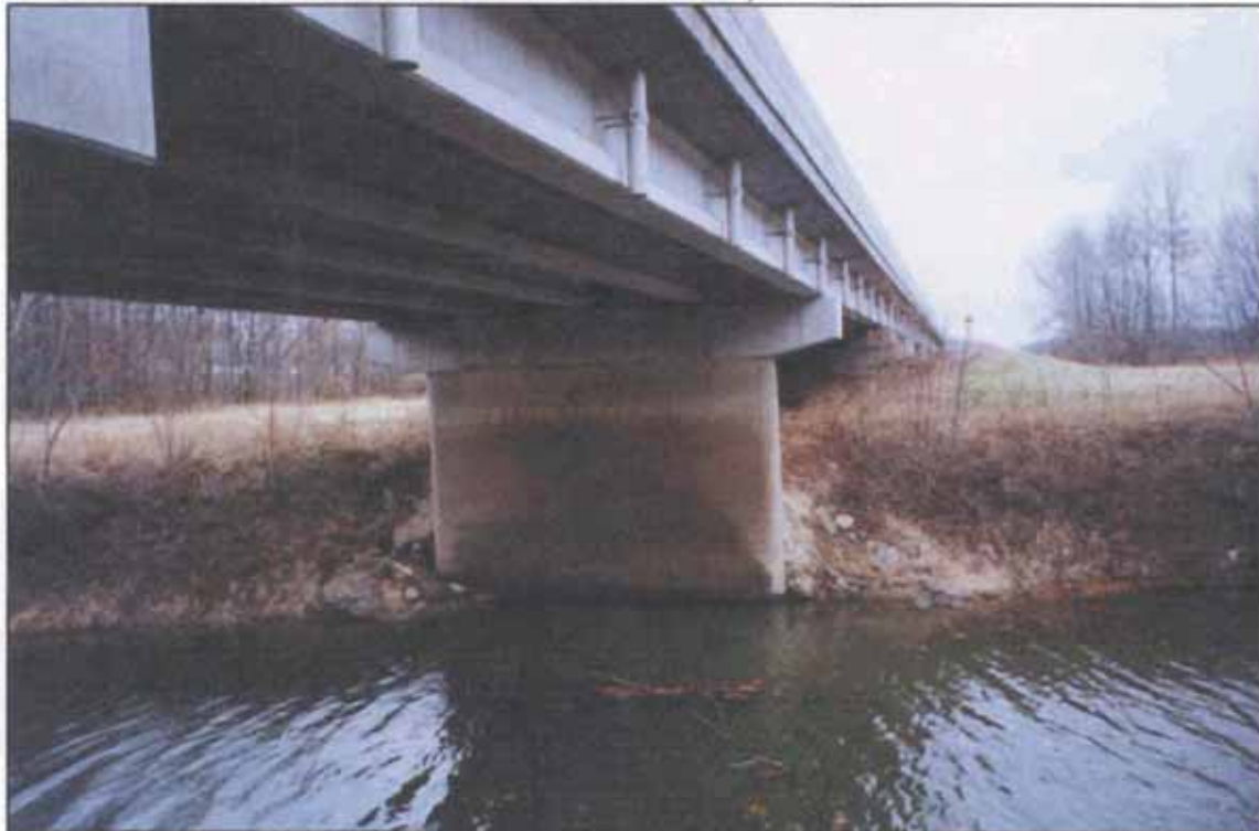
TYPICAL HAMMERHEAD PIER 5 FROM 1983, FACING EAST
