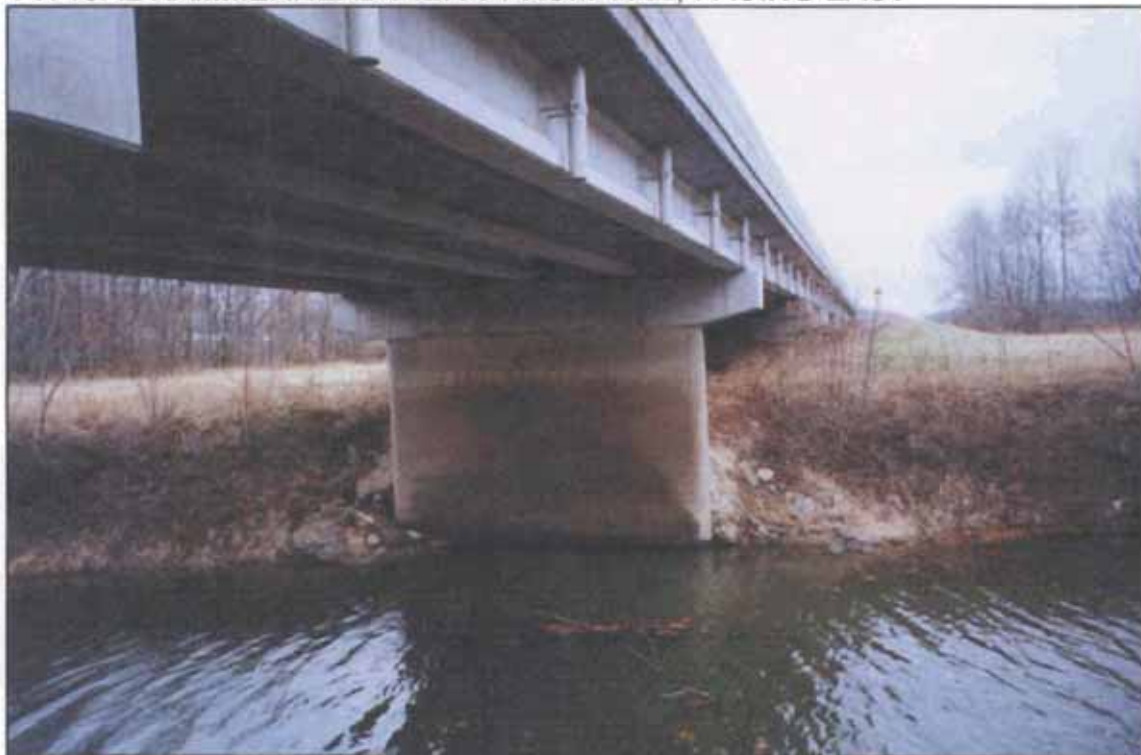
TYPICAL HAMMERHEAD PIER 5 FROM 1983, FACING EAST
