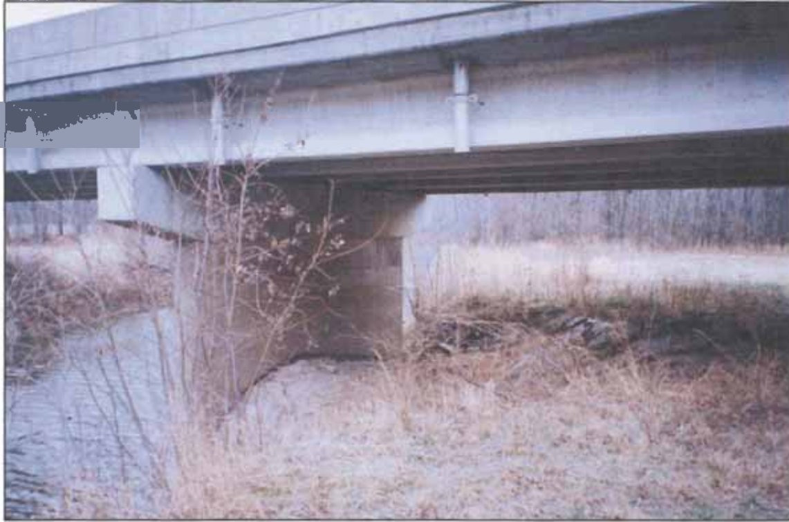
PIER 5, FACING NORTH
