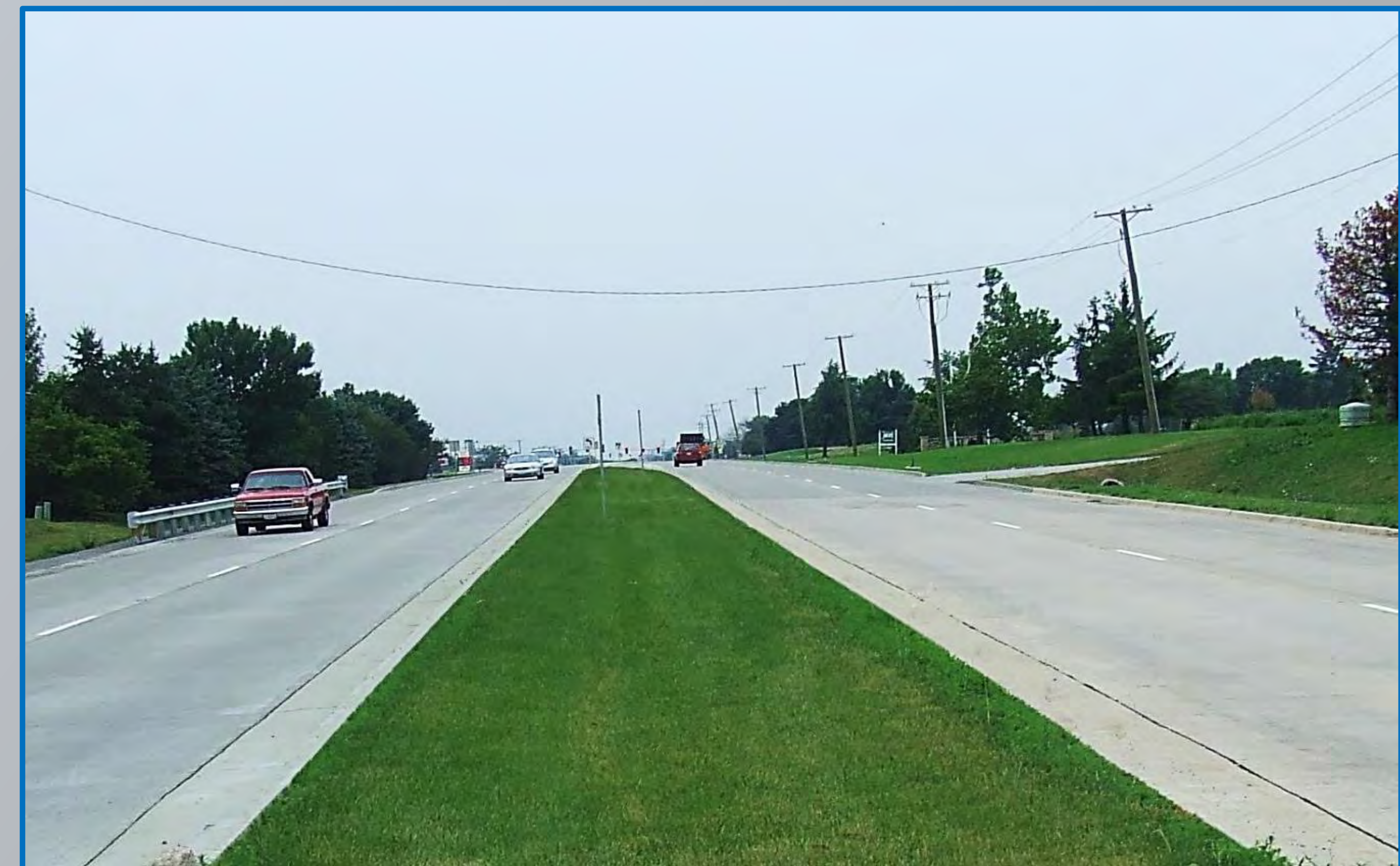
Example of a Landscaped Barrier Median
