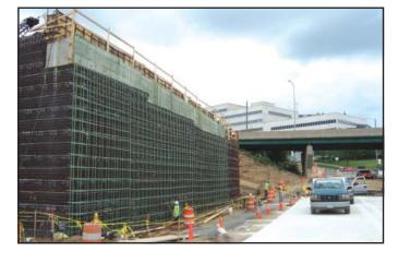
soil that not only gives strength to the entire soil mass, but also provides structural flexibility throughout the reinforced soil mass.
