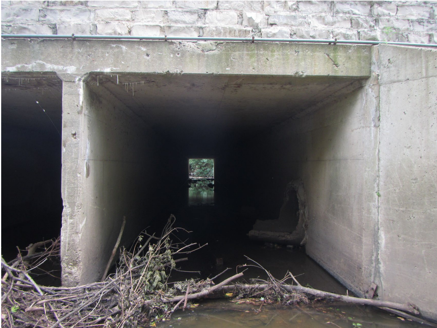
Figure 14: Existing culvert north headwall (cell 1)
