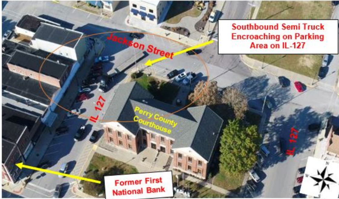
Figure 11 – Southbound Semi – Parking Spot Encroachment – IL 127
