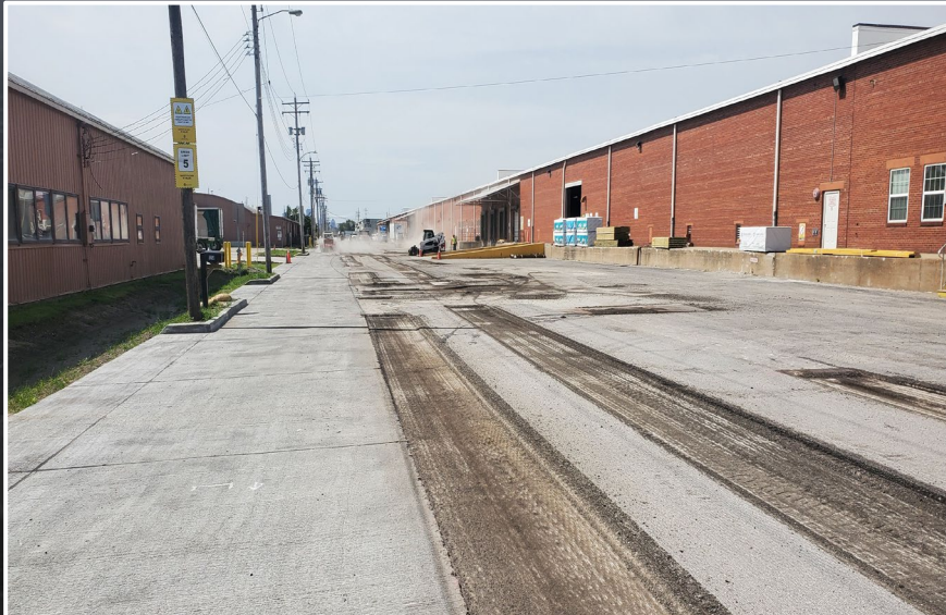
Removal of Degraded Pavement
