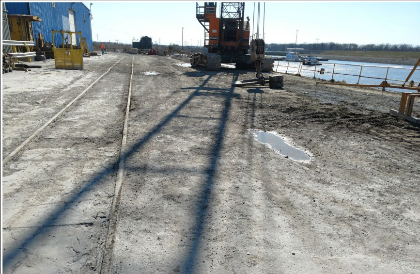
Original Dock Surface (Looking South)
