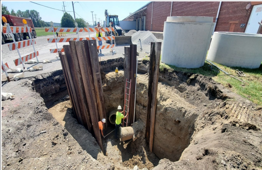
Original Sewer System is Deep
