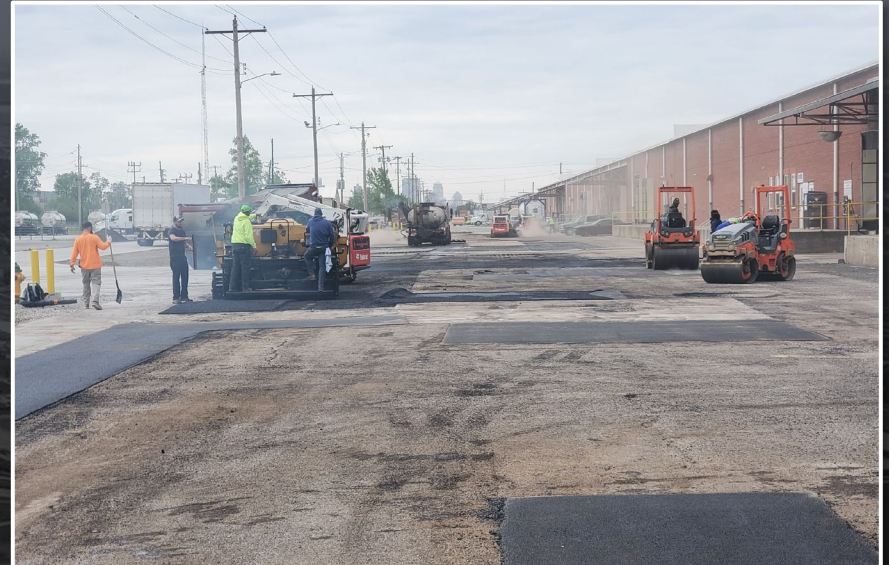
Patching of Degraded Pavement
