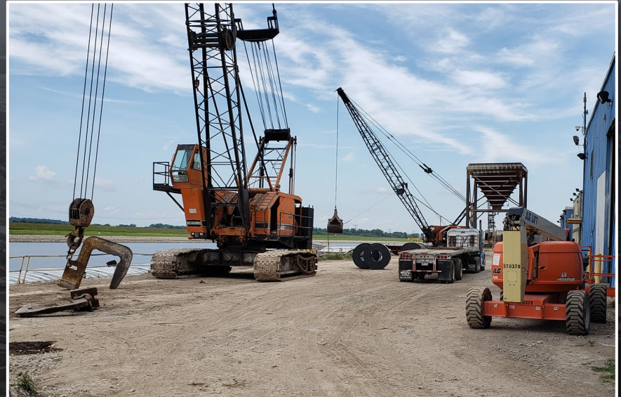
Original Dock Surface (Looking North)
