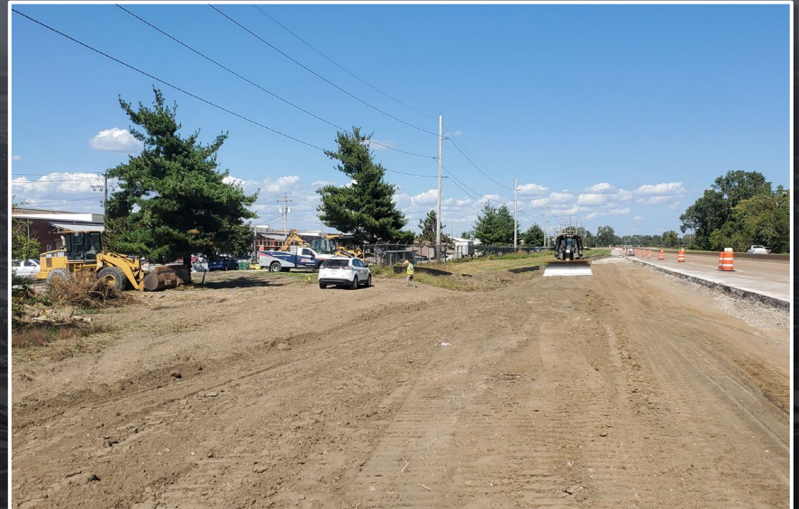
Cutting of New Deceleration Lane at Rt. 3
