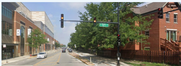
IDOT and CDOT collaborated to install barrier protected bike lanes on a state route, creating a more complete street.
