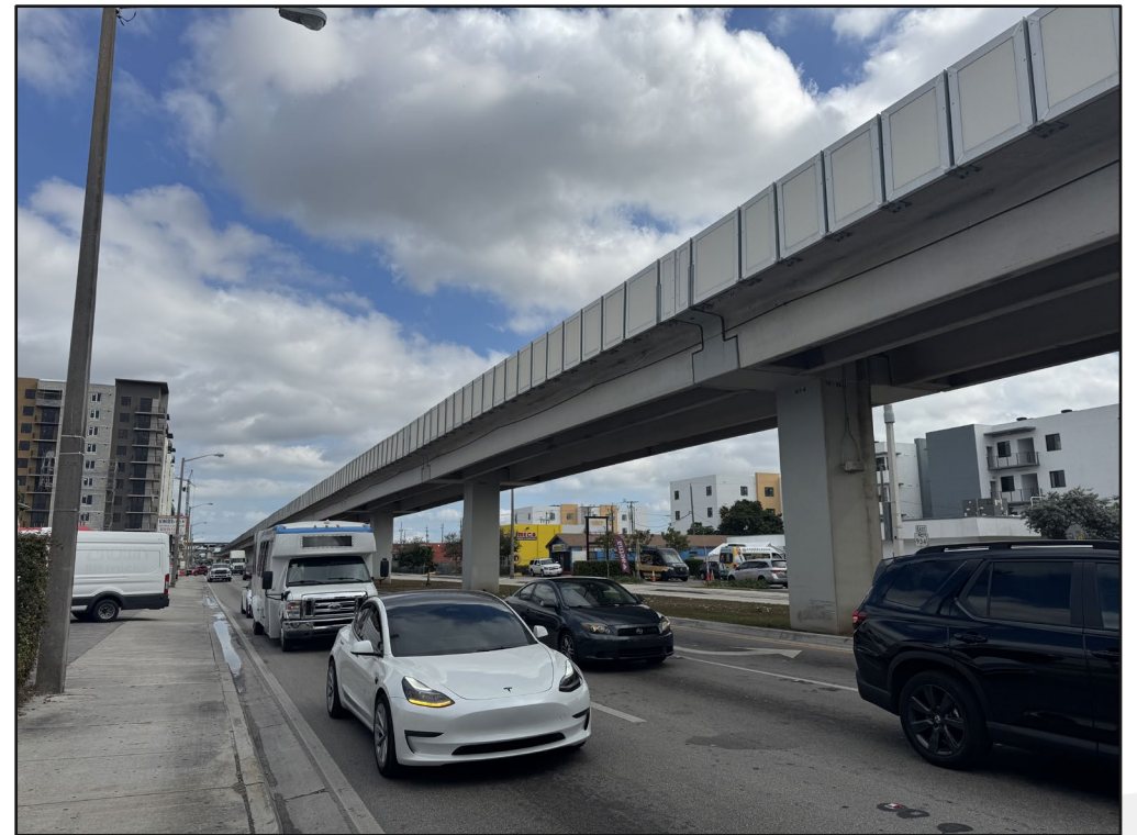
Miami Metrorail over 5-Lane Roadway
