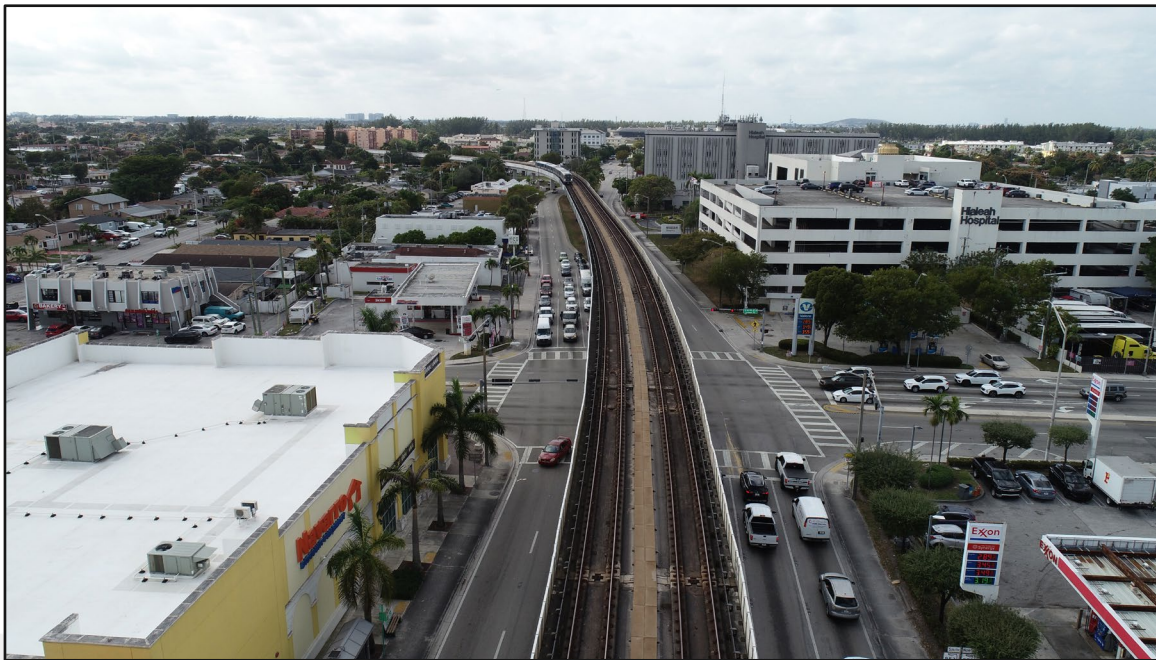
Miami Metrorail over 5-Lane Roadway
