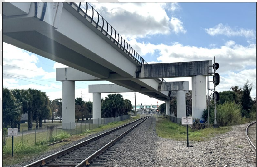
Figure 13 - Example of Elevated Track Constructed Over a Freight Railroad
